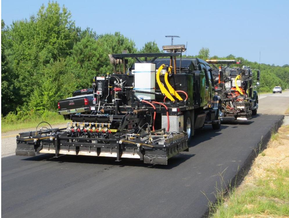
Figure 10: Hot-in-place recycling equipment on Section N8.
