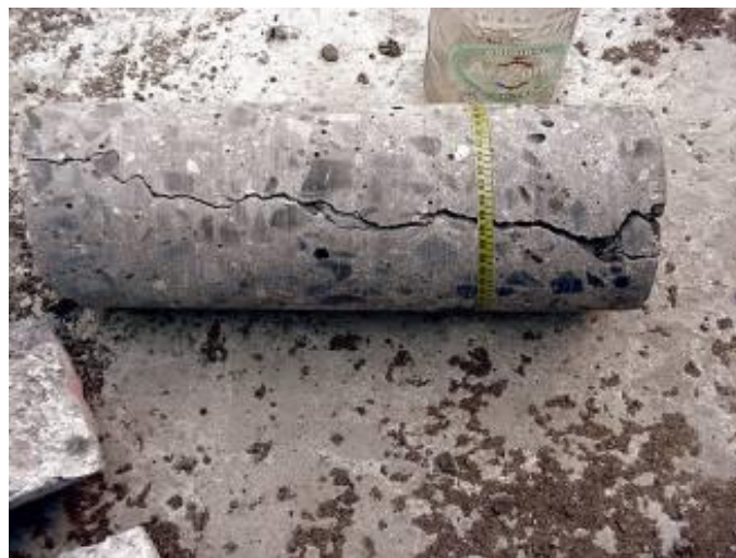
Figure 2-7: Concrete Core from Footing Where Insulation Blew Off During Cold Weather
