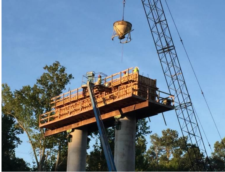
Figure 5-2: Photograph of Albertville Bent Cap
