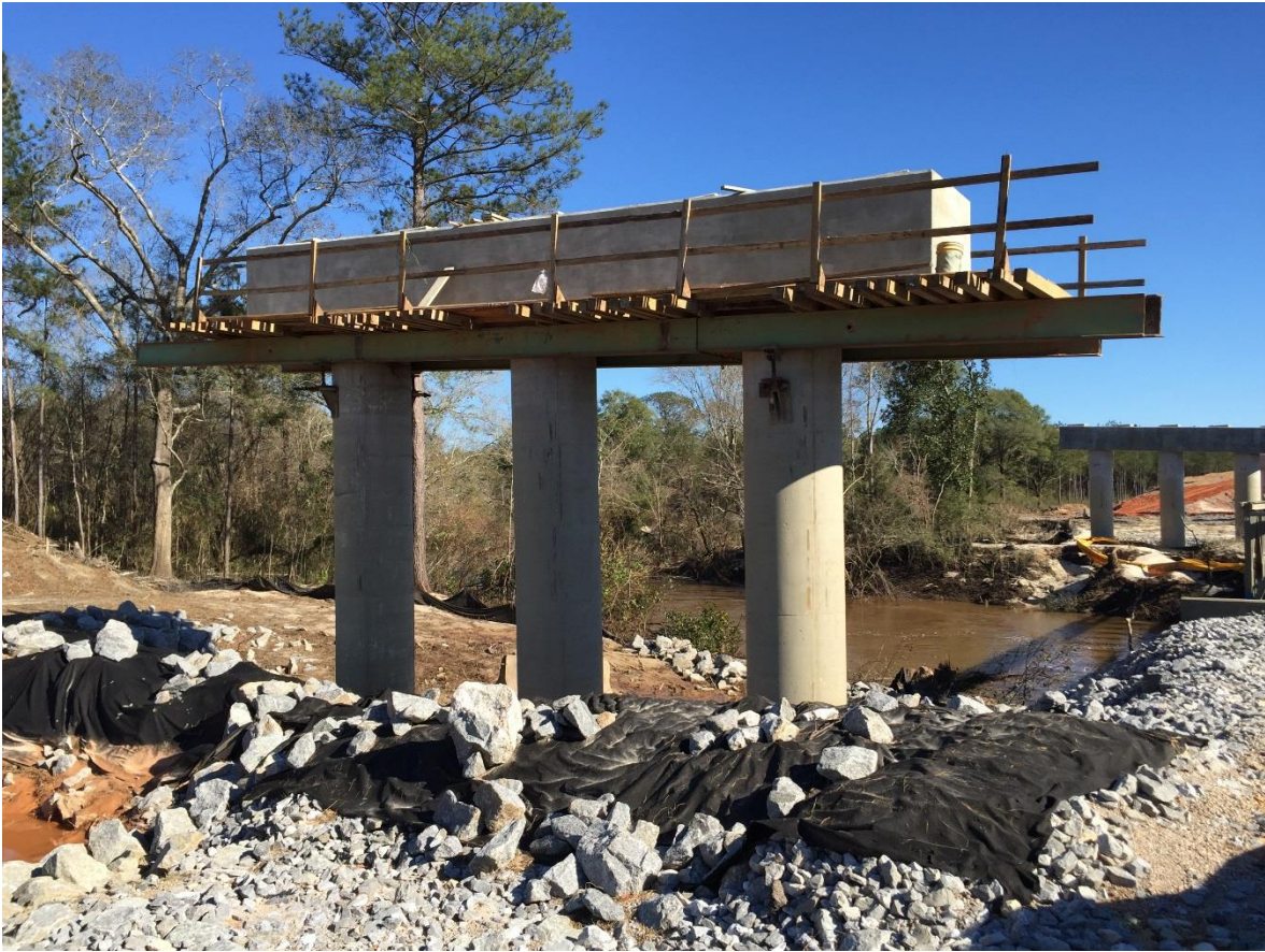
Figure 5-20: Photograph of Elba Bent Cap
