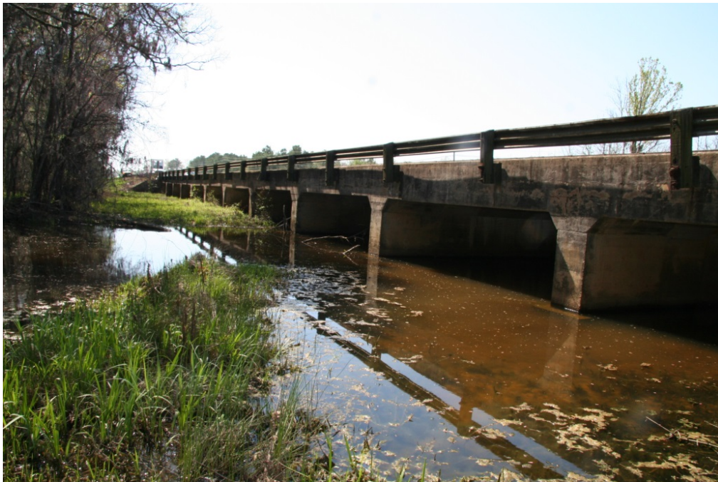
Figure 1-1: View of East Side of Barnes Slough Bridge
