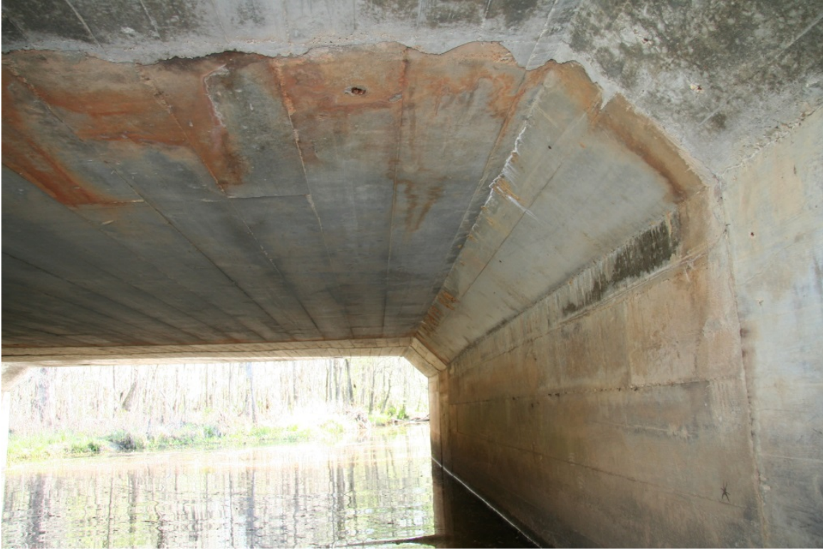
Figure 1-2: Bottom View of the Barnes Slough Bridge Looking East
