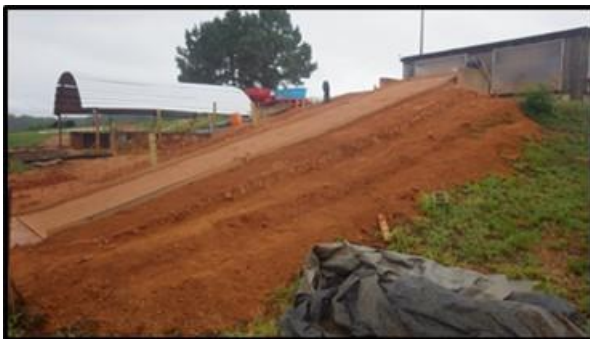
(a) terracing of side slopes for compaction
