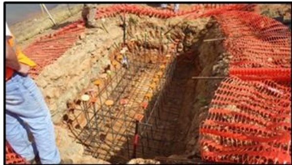
(b) steel reinforcement for basin
