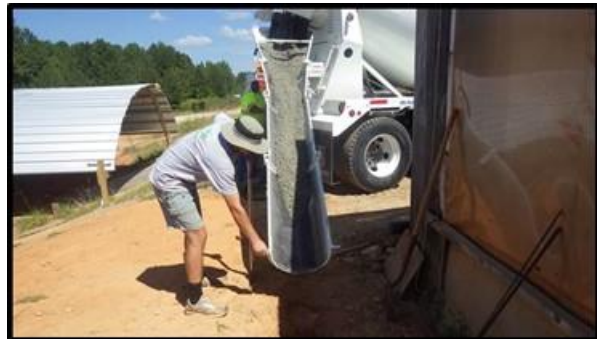
(b) pouring concrete footings
