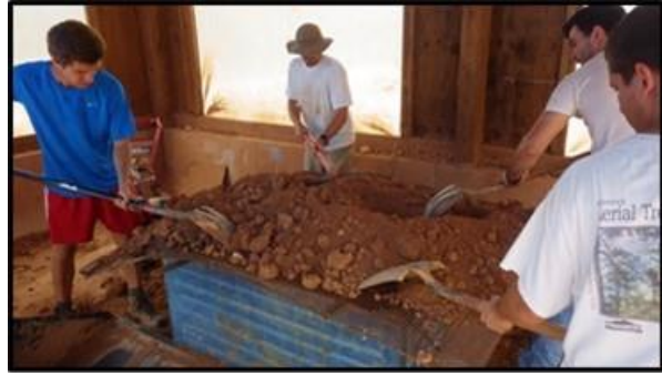
(b) screening the soil stockpile
