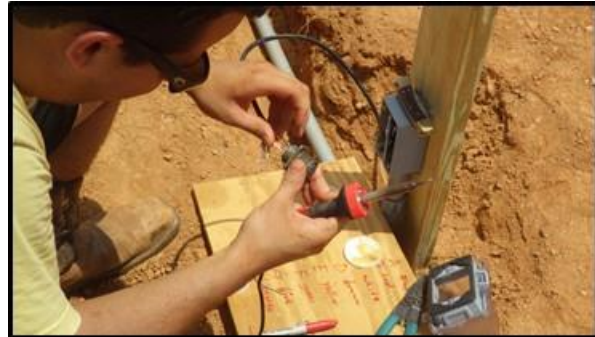
(b) installation of MIL-spec plug
