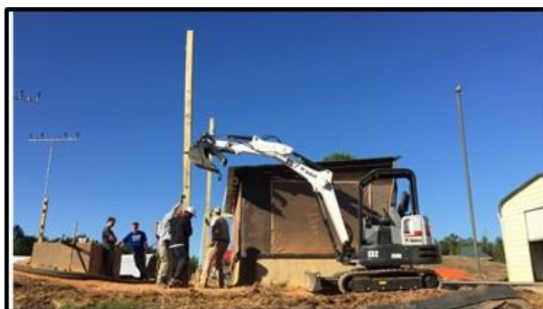
(e) installing top two support posts
