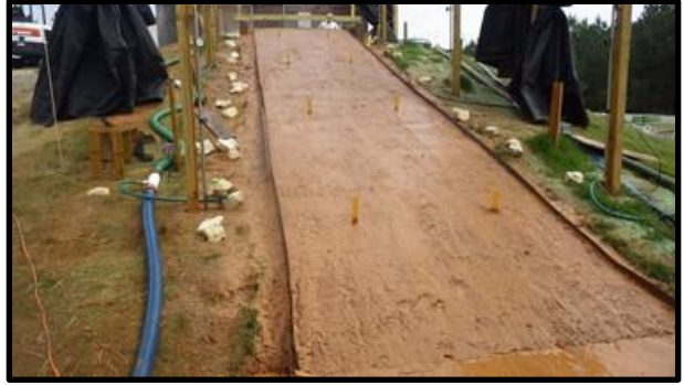
(b) slope erosion after interval 1
