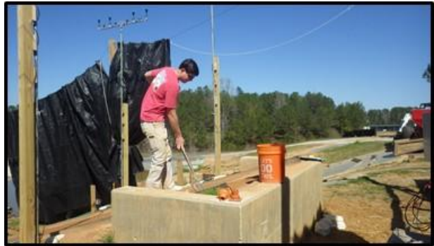
(b) excavating drive cylinder
