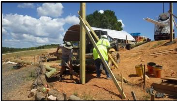
(c) placing concrete in post holes
