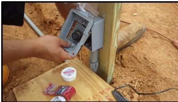
(c) installation of the gang box
