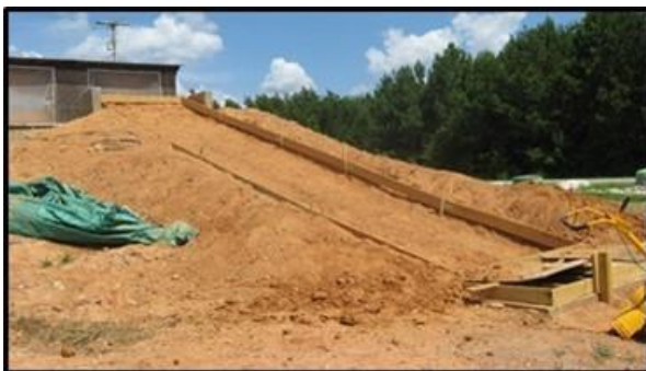
(a) excavation of test plot
