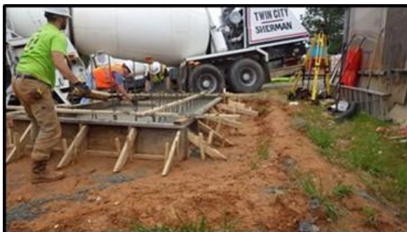
(c) pouring retaining wall footing
