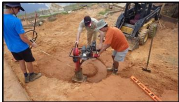
(b) compaction of slope with a rammer
