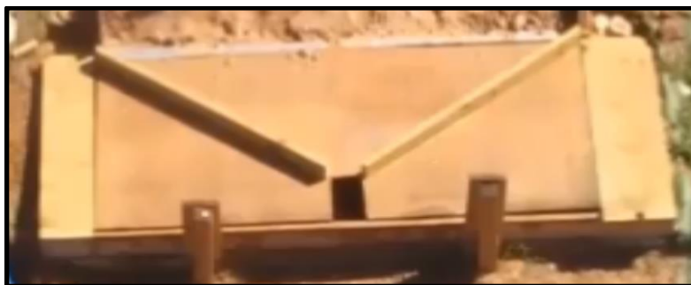
Figure 5.6 Flume for Channeling Runoff.
