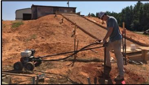
(a) drilling holes with an auger
