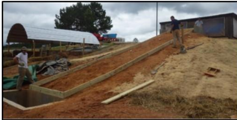
Figure 3.15 Test Plot Border Construction.
