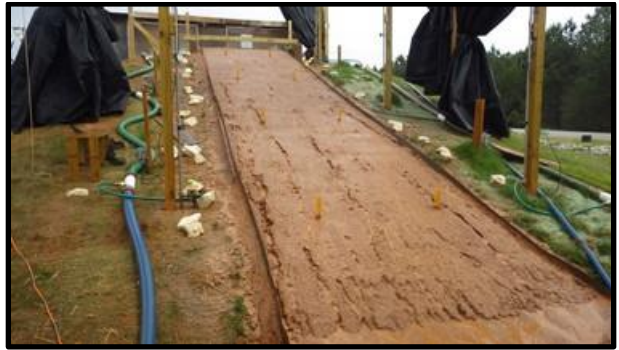
(f) slope erosion after interval 5
