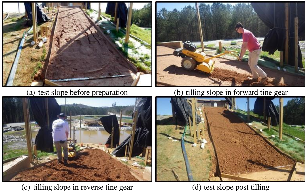
Figure 4.7 Slope Preparation Using Tiller.
