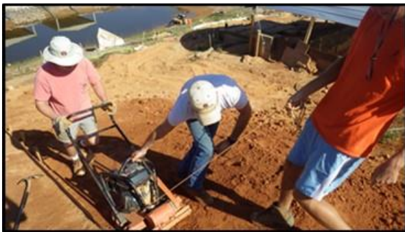
(c) compaction of slope with a plate compactor
