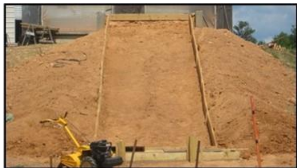
(b) excavation of test plot
