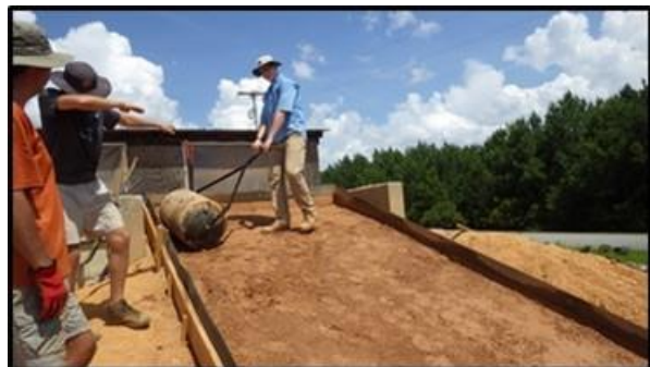
(f) compacting soil with a turf roller
