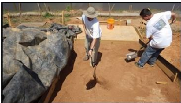
(e) spreading soil with shovels
