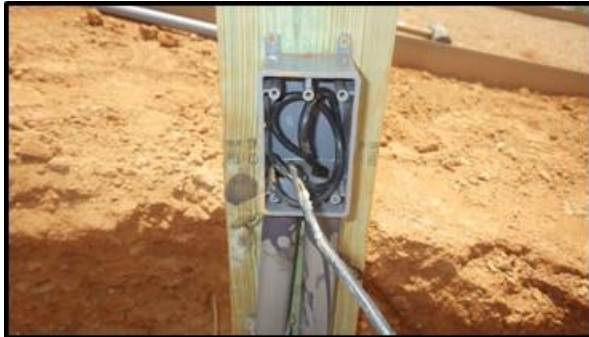
(a) installation of junction box and cable
