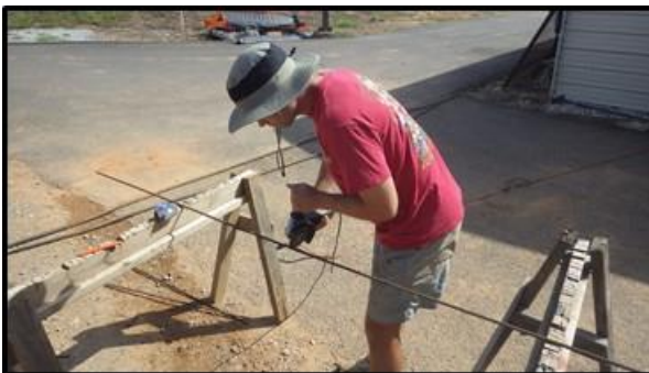
(c) cutting rebar for footings
