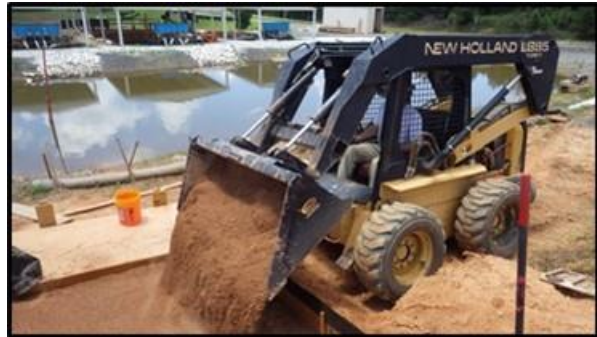
(d) backfilling test plot with screened soil
