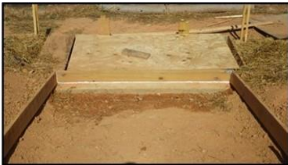
(c) border joints sealed with caulk
