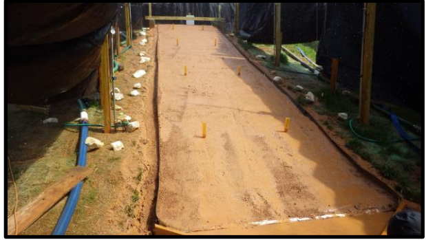
(b) slope erosion after interval 1
