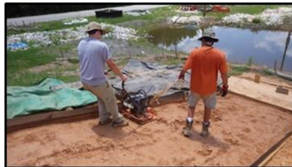
(g) compacting slope with a plate compactor
