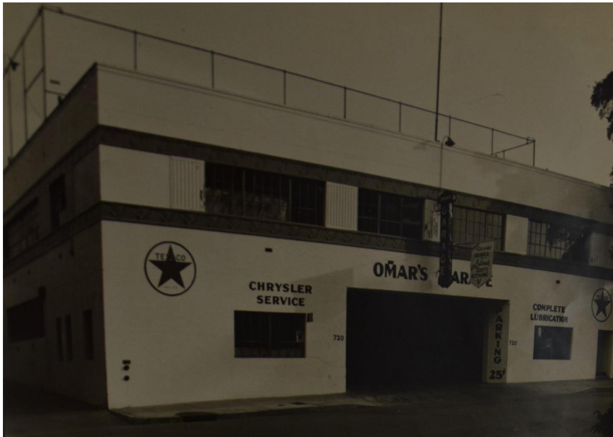
Figure 26: Omar's Garage before Airfloat 40
