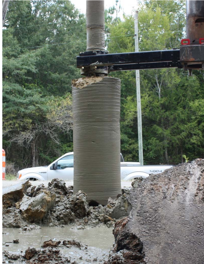
Figure 74: Extracted Column of Soil from Deep Mix Column
