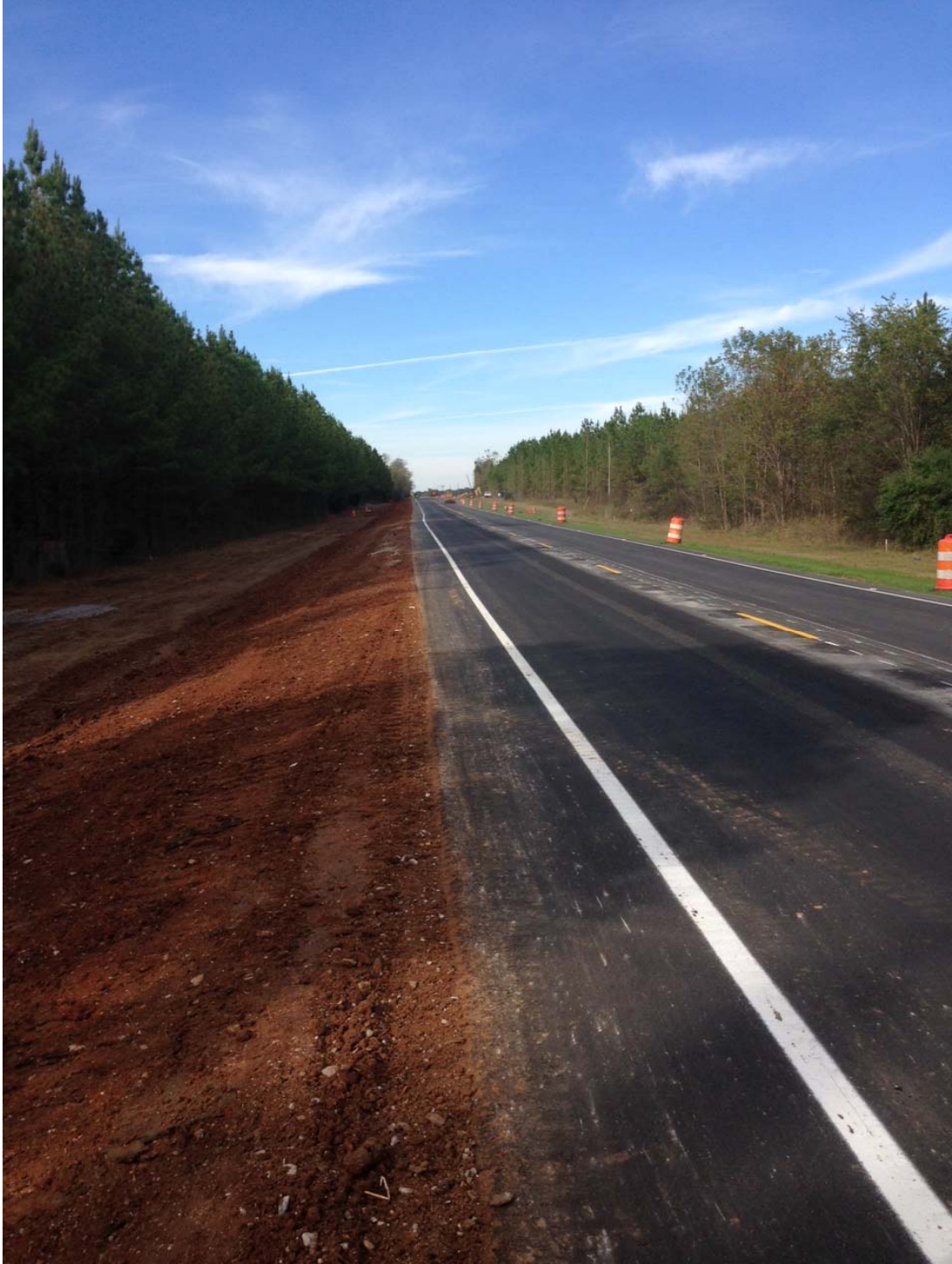
Figure 41: Completed Sand Blanket Test Section
