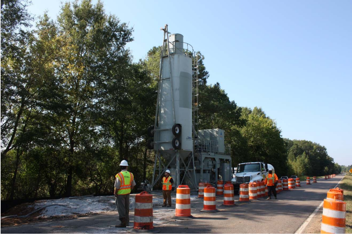
Figure 72: Deep Mix Column Batch Plant
