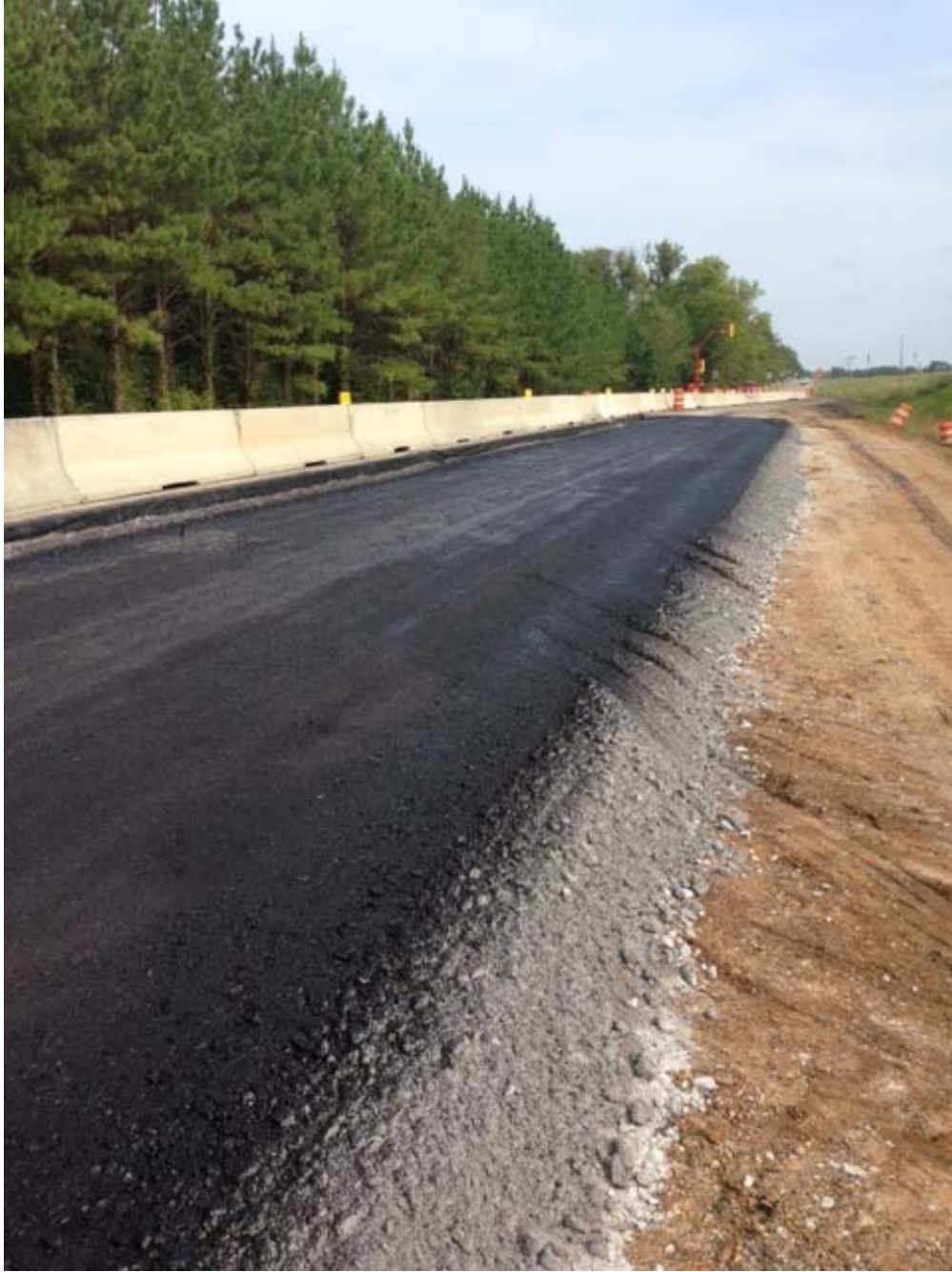
Figure 39: North Bound Lane – Placement of Tack Coat on Granular Base
