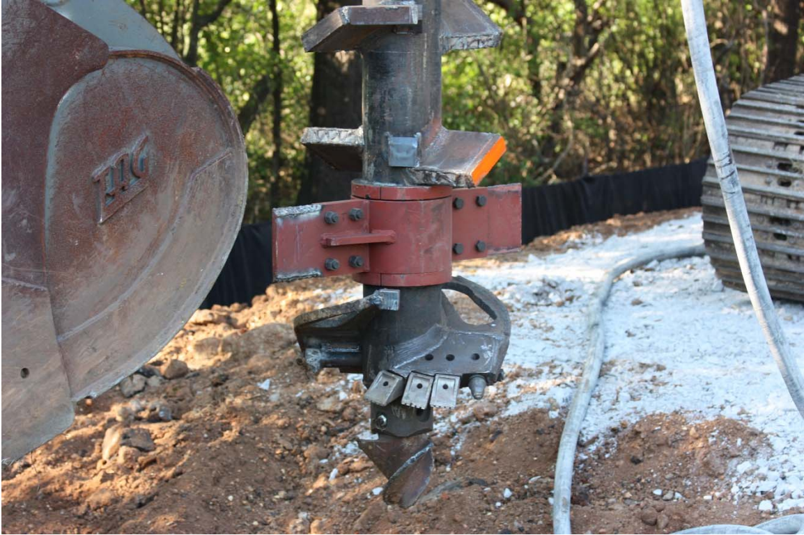
Figure 73: Drill Bit used for Deep Mix Column Installation
