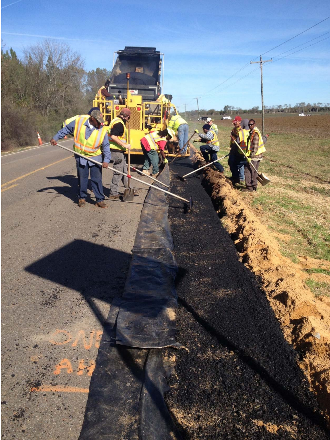
Figure 48: Leveling Asphalt over Vertical Barriers
