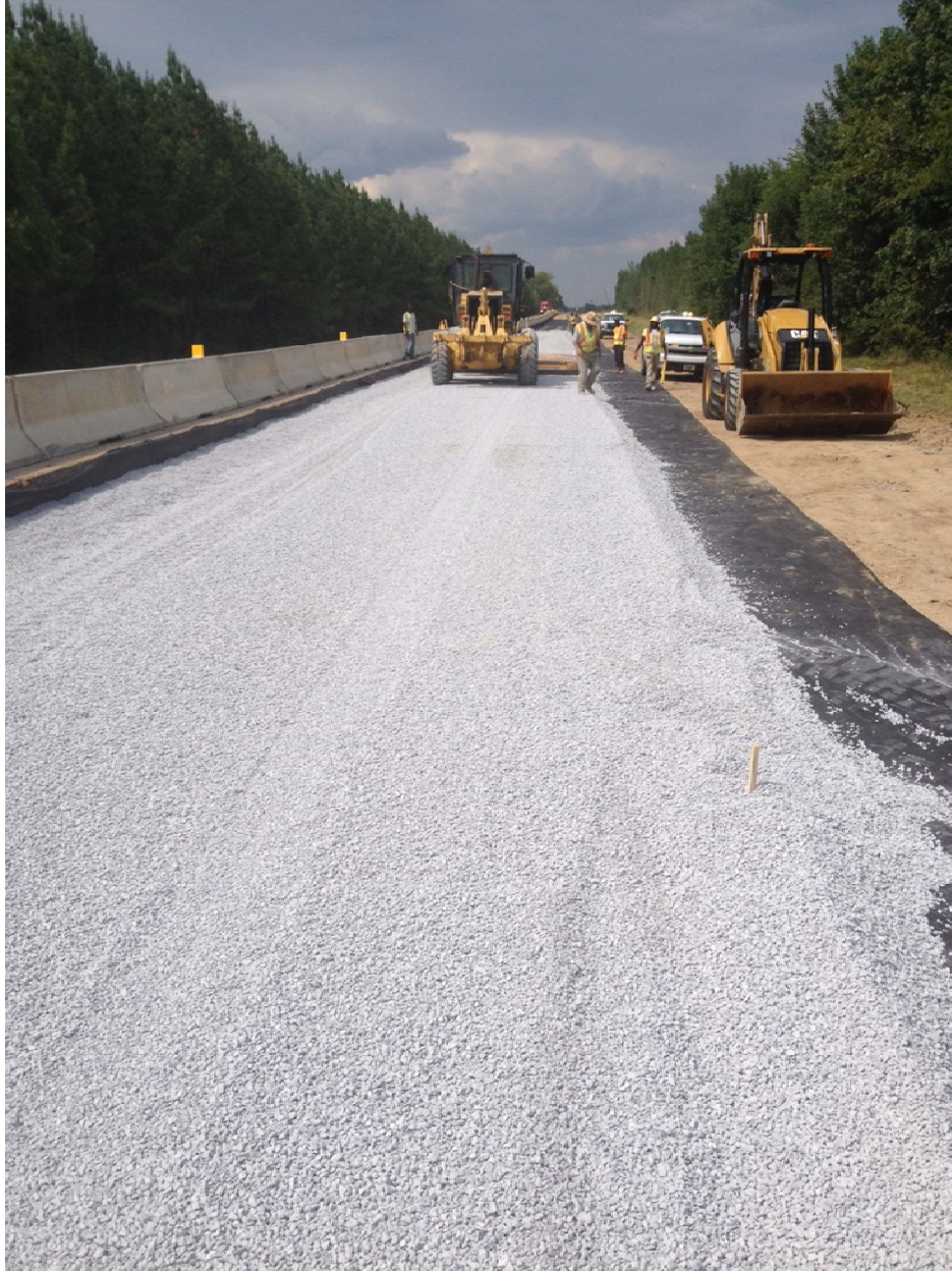
Figure 38: North Bound Lane – Application of Sand Blanket
