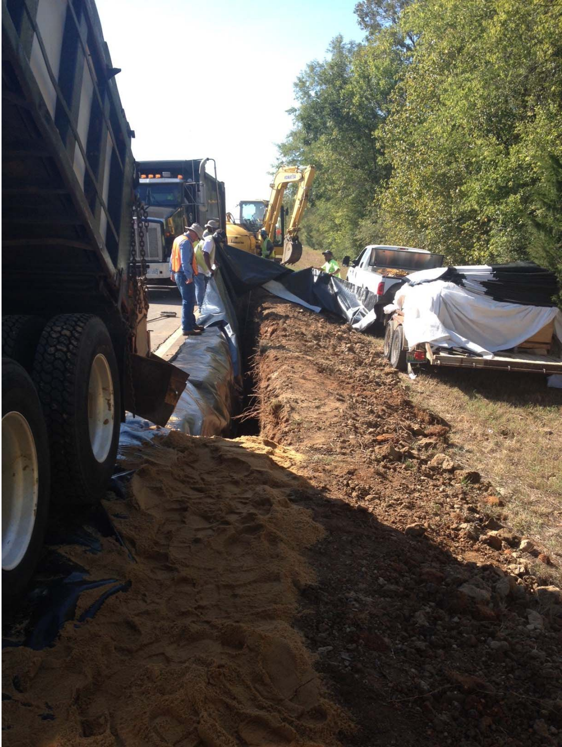
Figure 45: Backfilling of Vertical Barriers
