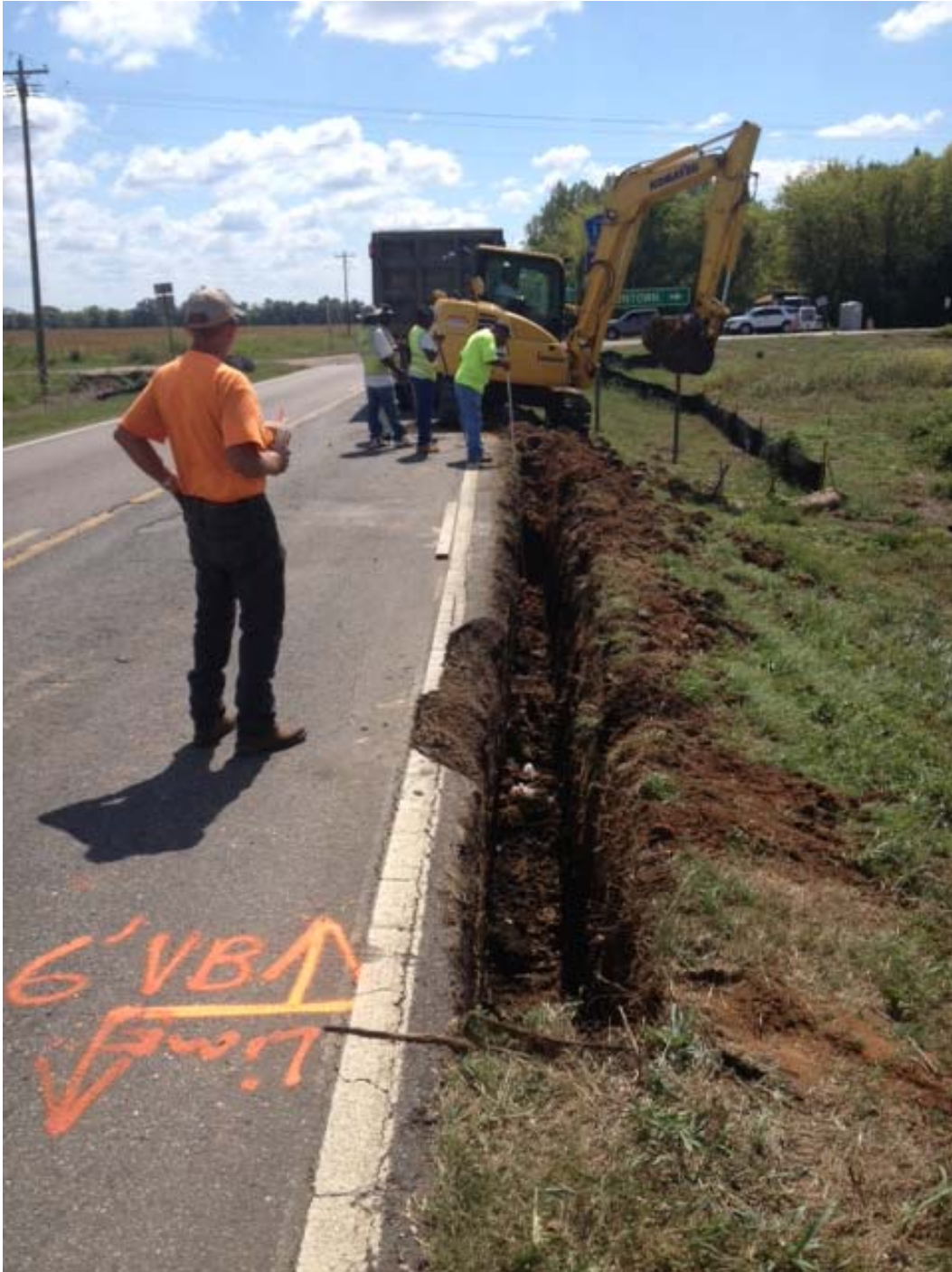
Figure 44: Vertical Barrier Trench
