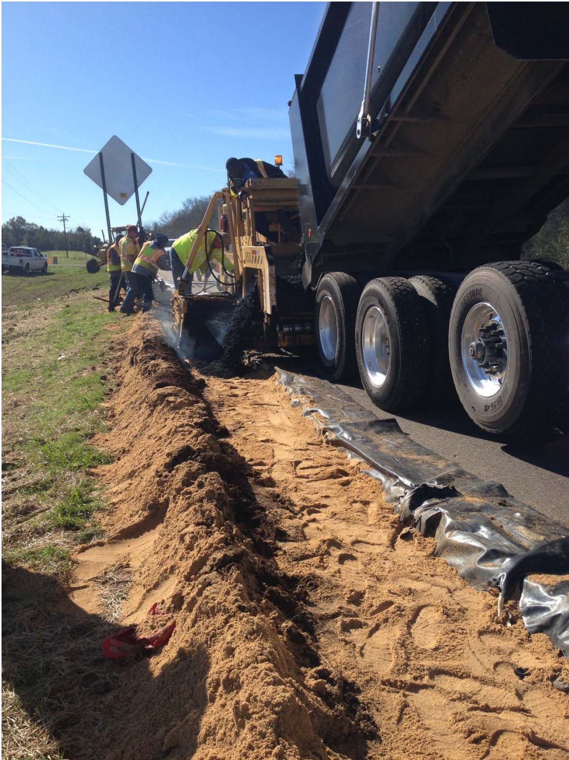
Figure 47: Paving over Vertical Barrier Trench
