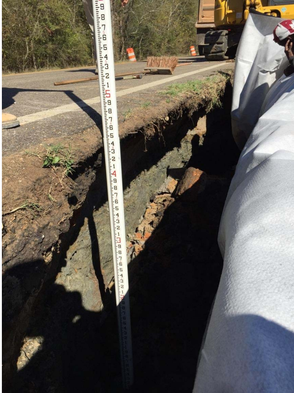
Figure 43: Trench Cave-in – Vertical Barriers
