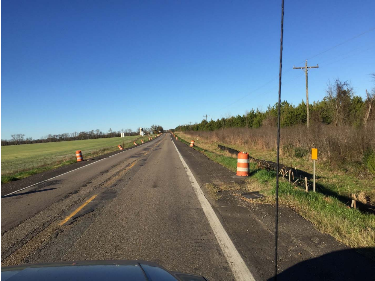
Figure 66: Paved Shoulder prior to Leveling Course
