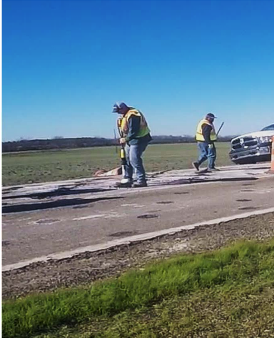
Figure 60: Compacting asphalt in Lime Column
