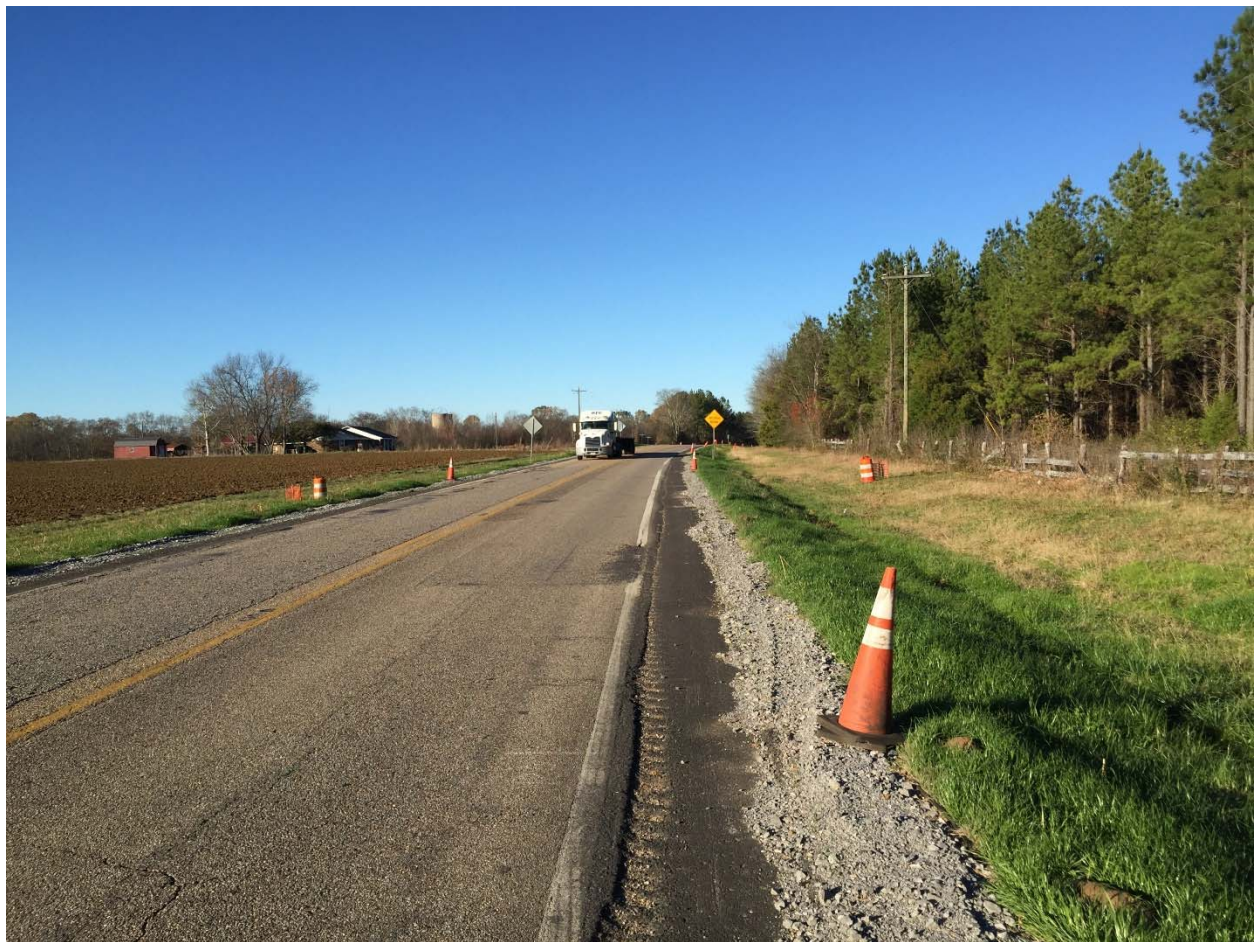
Figure 68: Edge Drains after Backfilling with Stone
