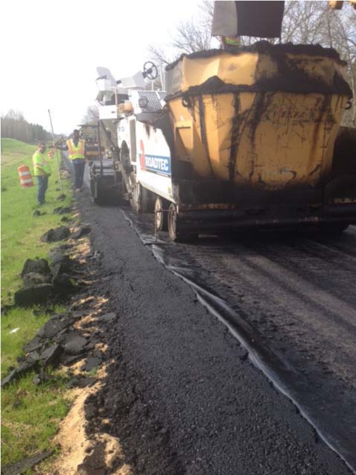
Figure 49: Leveling of Pavement over Vertical Barriers
