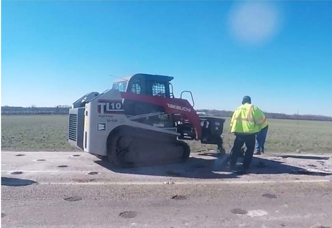
Figure 59: Pouring Asphalt into Lime Column Holes
