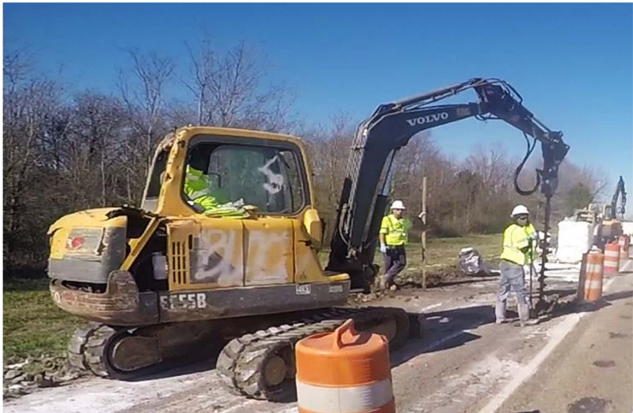
Figure 56: Drill Used for Lime Column Installation
