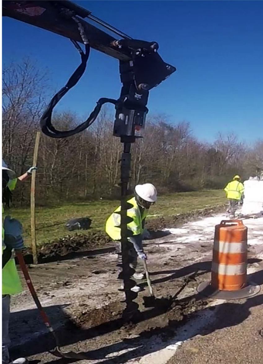
Figure 57: Auger used for Lime Column Installation
