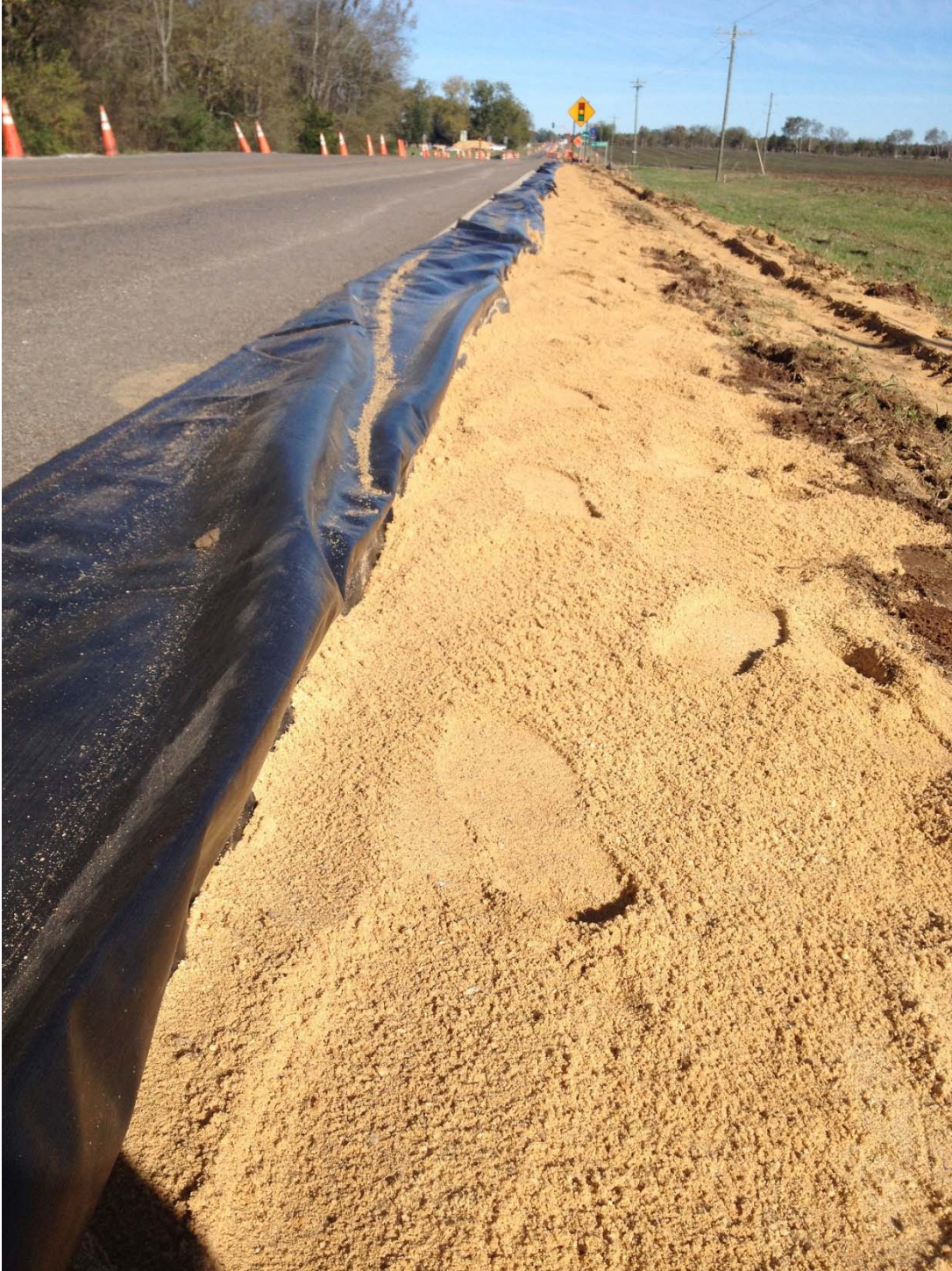
Figure 46: Sand Backfill of Vertical Barriers
