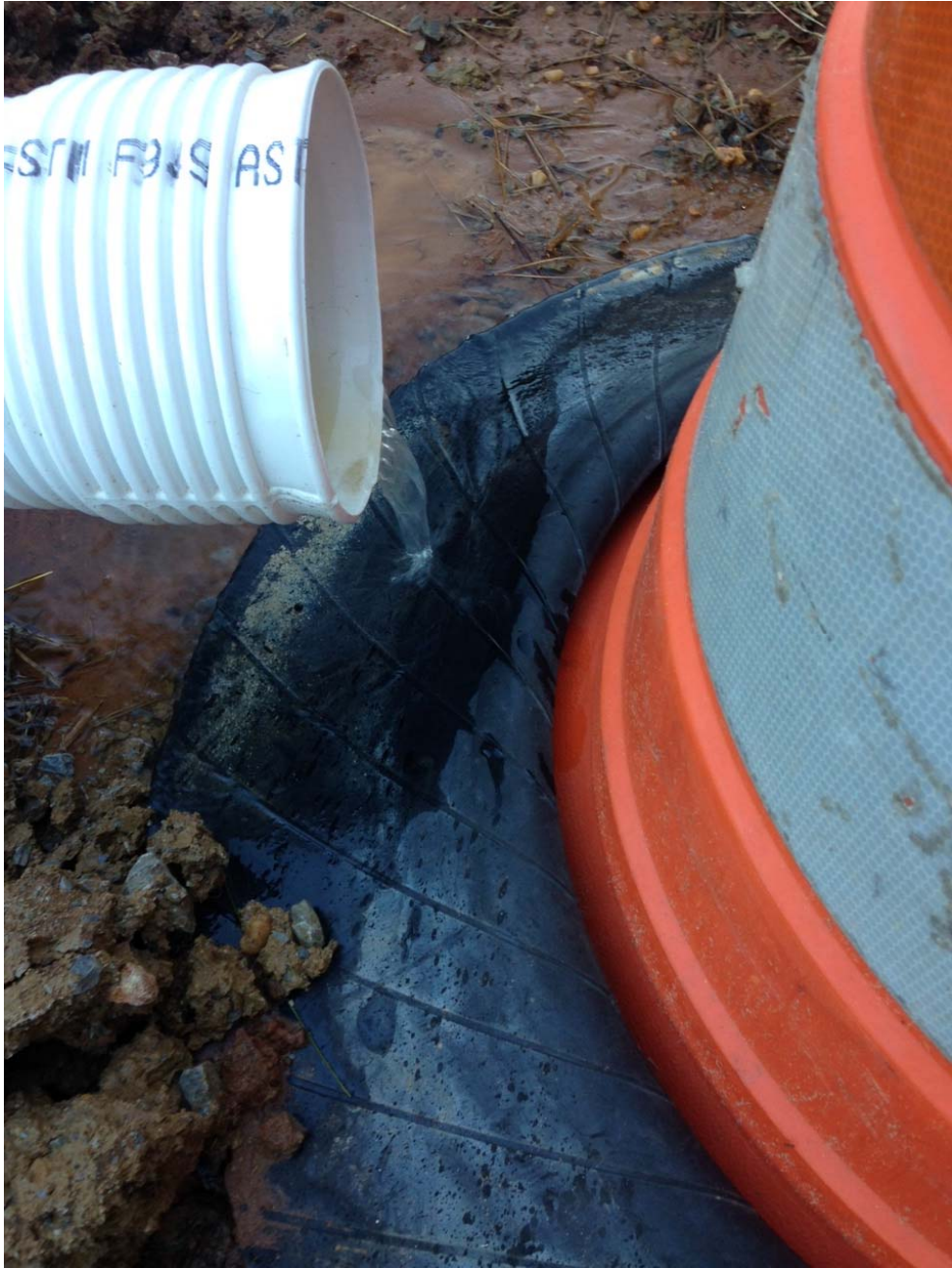
Figure 40: Rainwater flowing out of Sand Blanket
