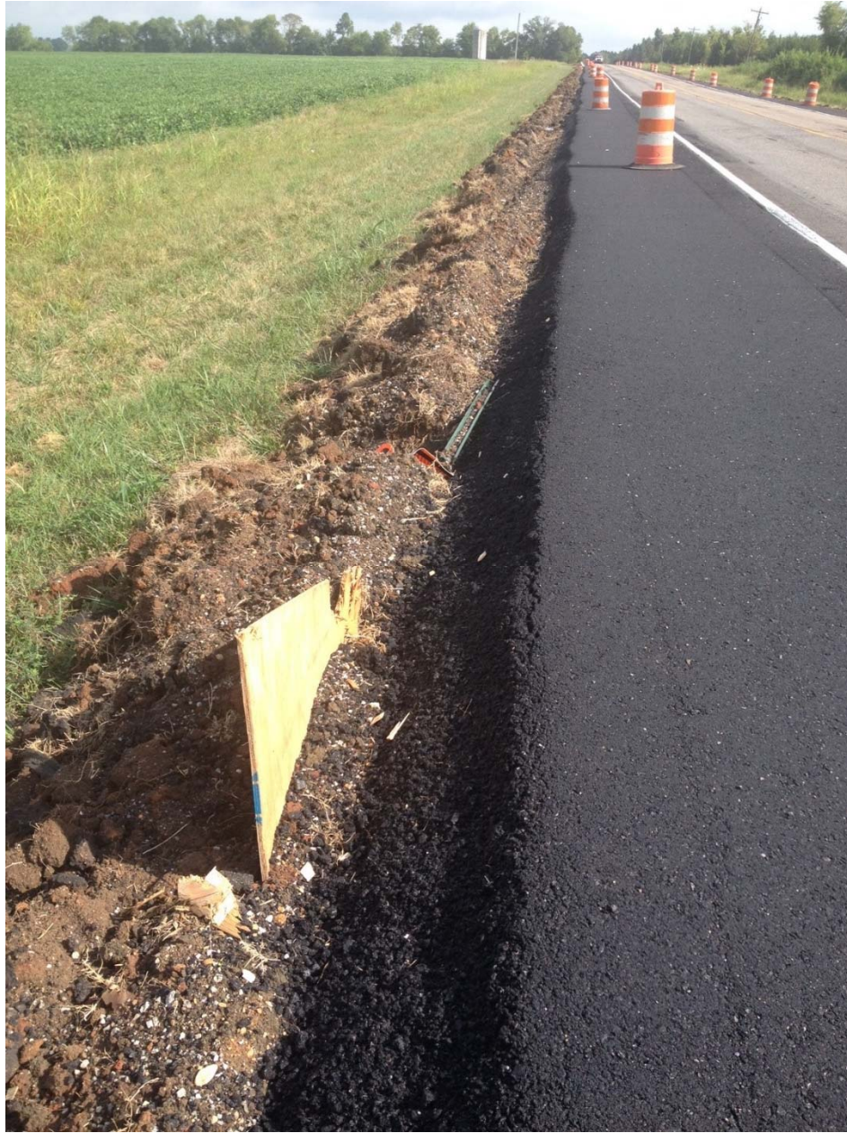
Figure 65: After paving of Paved Shoulders
