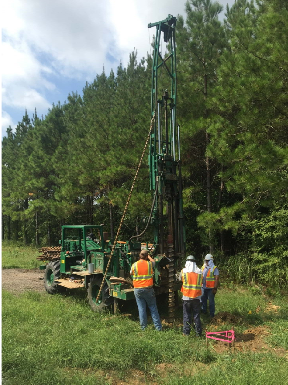
Figure 78: ATV Drill Rig used for Hydroprobe Installation
