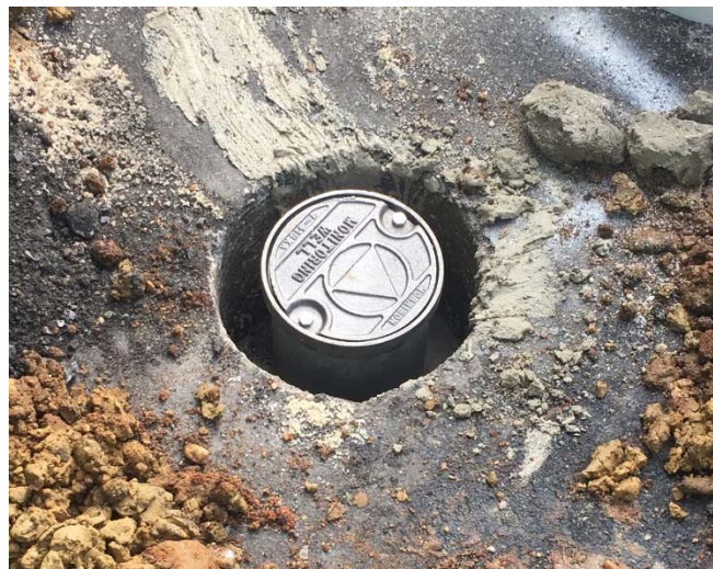
Figure 80: Waterproof Manhole Cover before grouted in place
