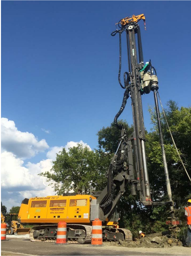
Figure 71: Deep Mix Column Drill Rig
