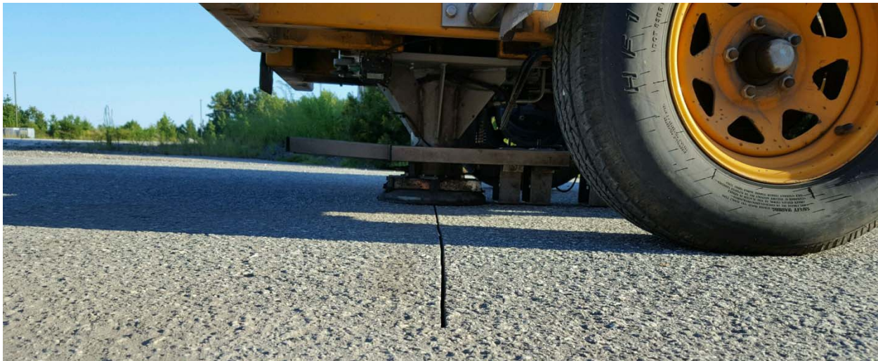
Figure 3.17 – FWD testing over saw-cut discontinuity.
