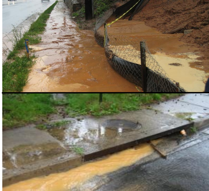
Figure 5 - Sediment-laden water from site with overwhelmed silt fence draining to sewer. Reference: environment.arlington.us/2014/07/see
