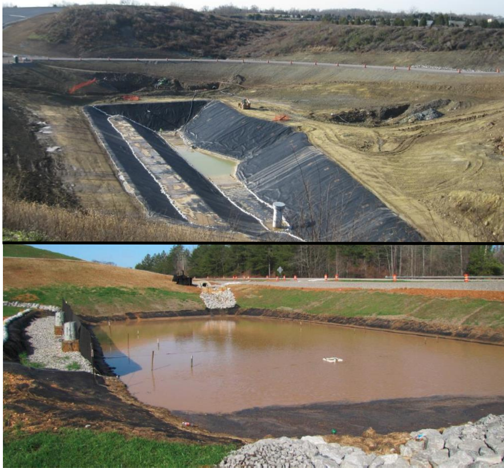
Figure 7 – Sediment basin in large construction site (top). Reference: thewalkercompany.com. Sediment basin full of turbid water (bottom). Reference: mdpi.com/water
