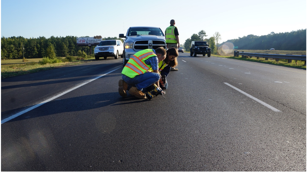
Figure C-3: Installation of NC-350 on I-59/I-20 Veronica Ramirez and Dr. Rod Turochy
