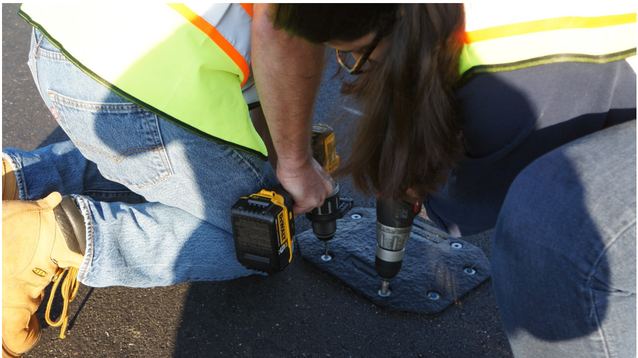
Figure C-6: Installation of NC-350 on I-59/I-20 Veronica Ramirez and Dr. Rod Turochy
