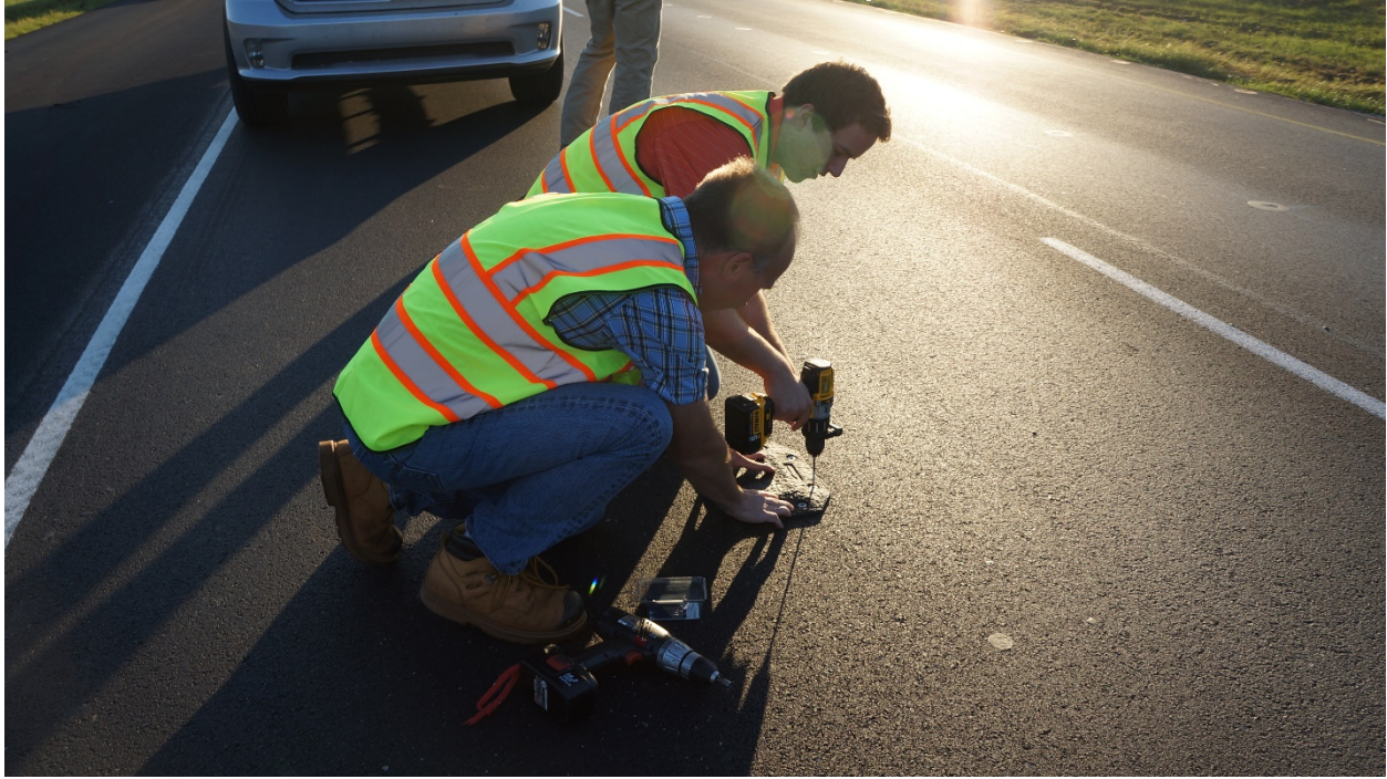
Figure C-1: Installation of NC-350 on I-59/I-20 Nick Jehn and Dr. Rod Turochy
