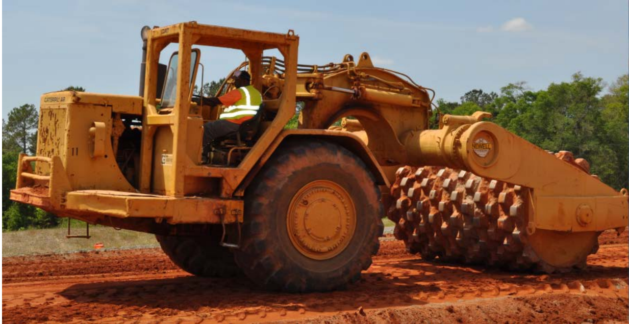
Figure 2.13: Sheepfoot roller used to compact fine-grained soil-cement base
