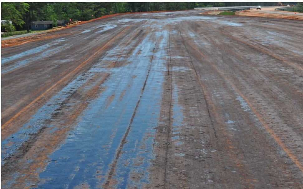
Figure 2.16: Asphalt emulsion placed on the soil-cement base
