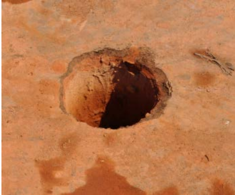
Figure 3.34: Core hole on U.S. Highway 84 bypass project in Elba, Alabama
