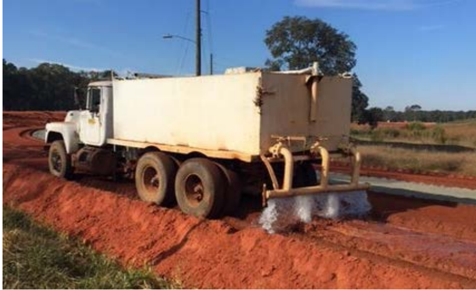
Figure 2.8: Water truck used in mixed-in-place construction
