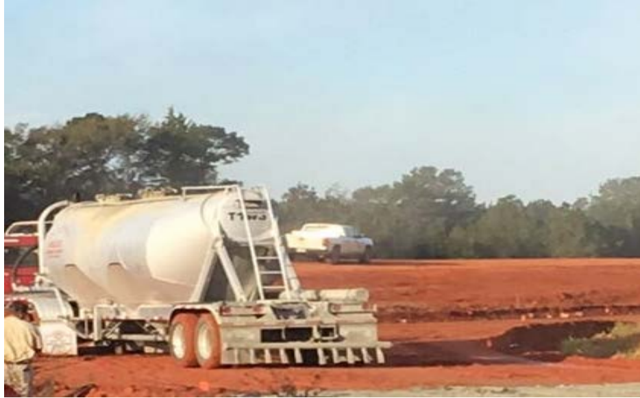
Figure 2.6: Bulk-cement truck with mechanical spreader used to place cement
