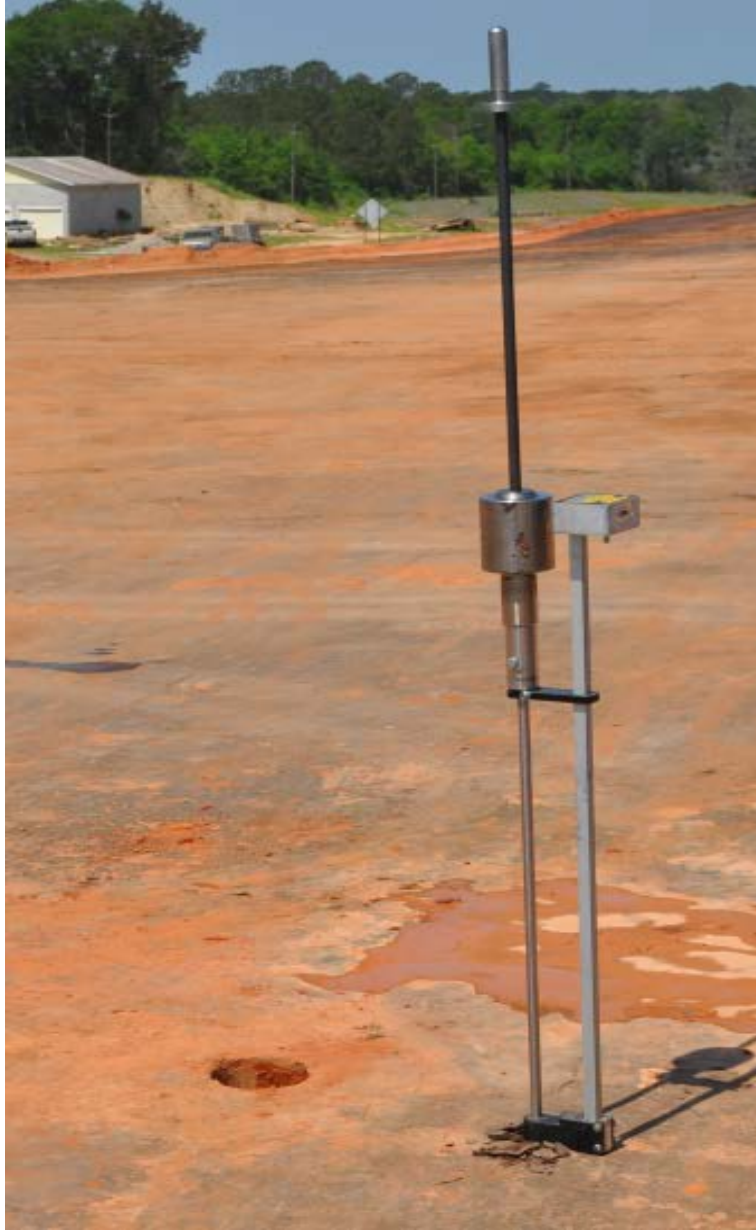
Figure 3.33: DCP tested conducted at a core hole location equipped with a magnetic ruler
