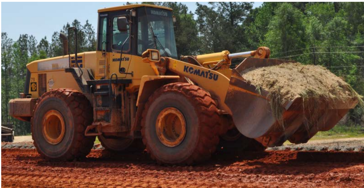
Figure 2.12: Front-end loader used for initial compaction
