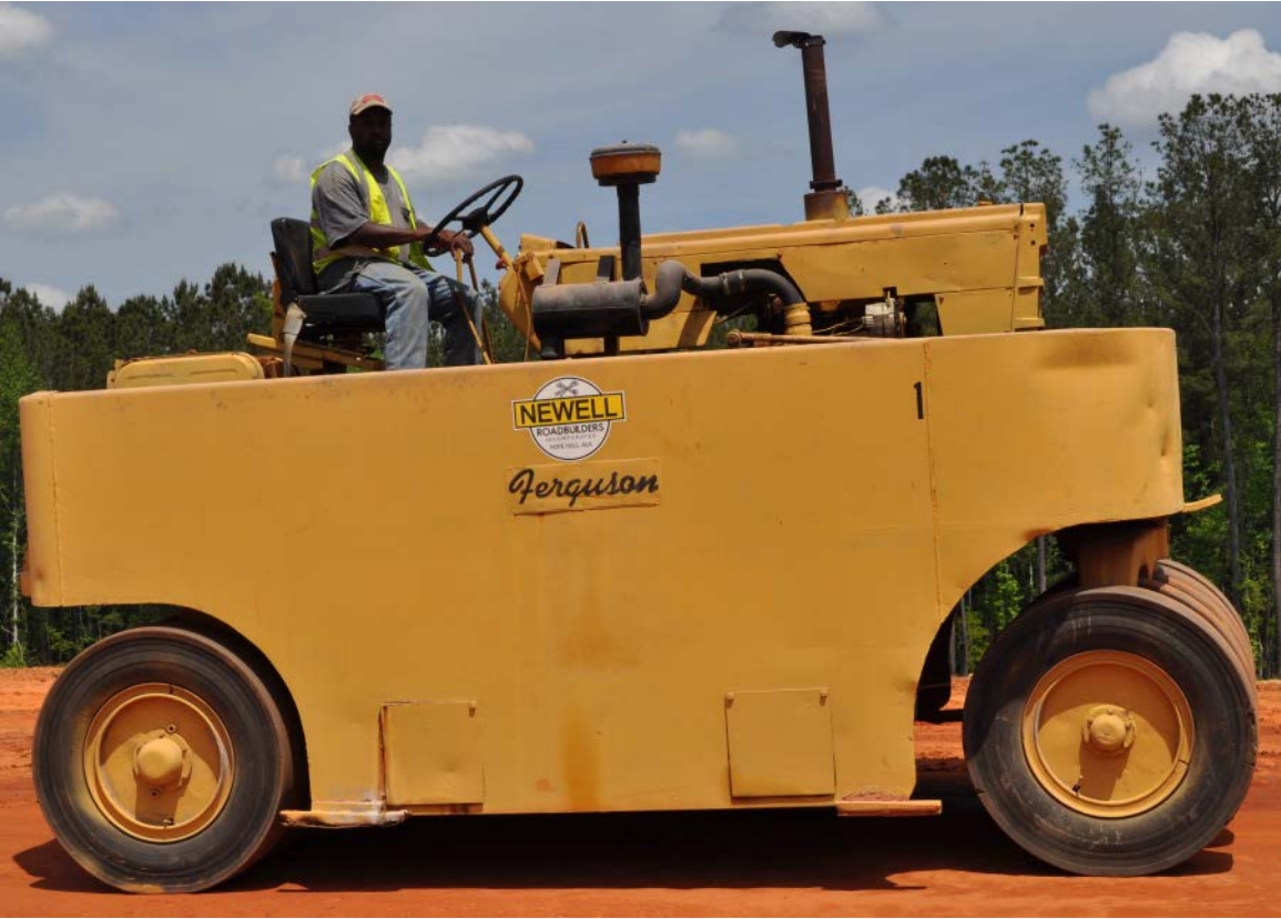
Figure 2.14: Multiple-wheel, rubber-tire roller used to compact soil-cement base
