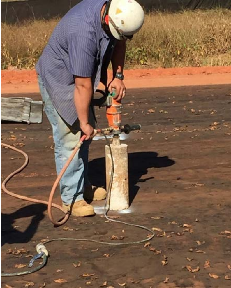
Figure 2.19: Coring operation on U.S. Highway 84 in Elba, Alabama
