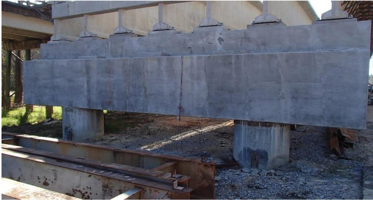
Figure 5-39: Brewton bent cap during bridge construction
