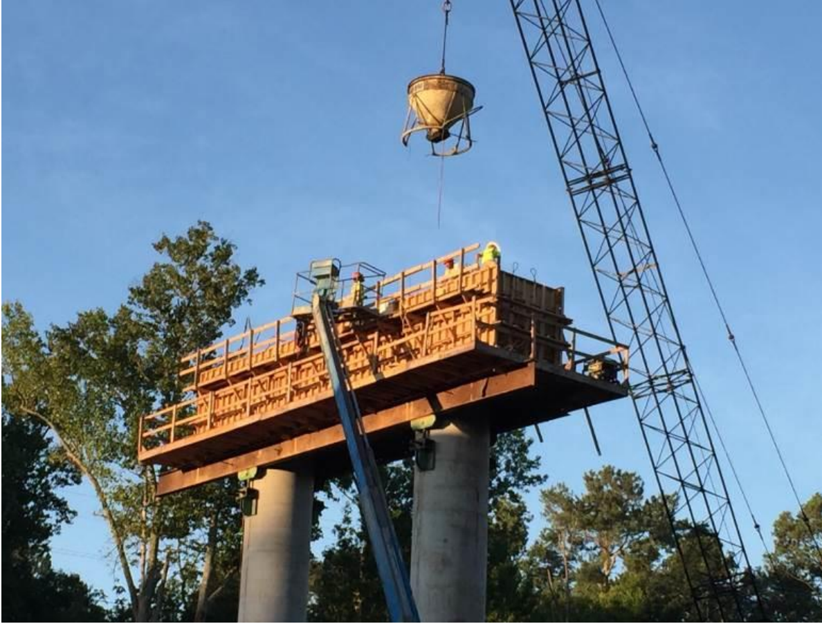
Figure 5-1: Albertville bent cap (Eiland 2015)
