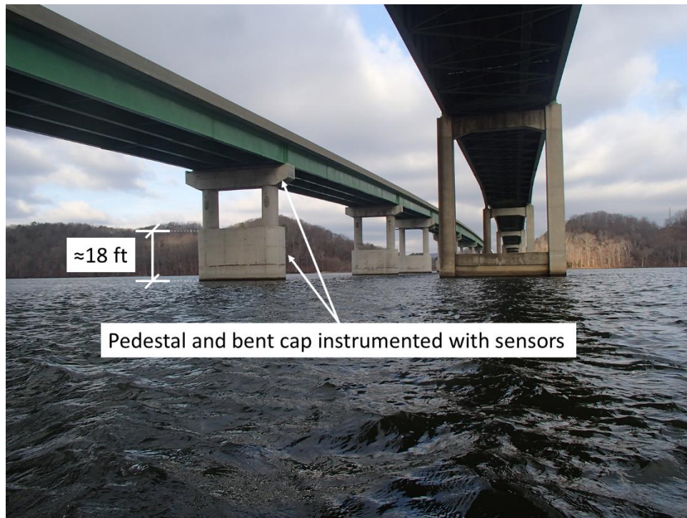
Figure 5-18: Scottsboro pedestal and bent cap on day of inspection on 2/9/2017
