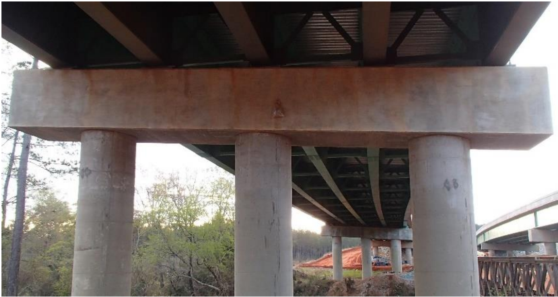
Figure 5-29: Elba bent cap during construction (top) and post construction (bottom)
