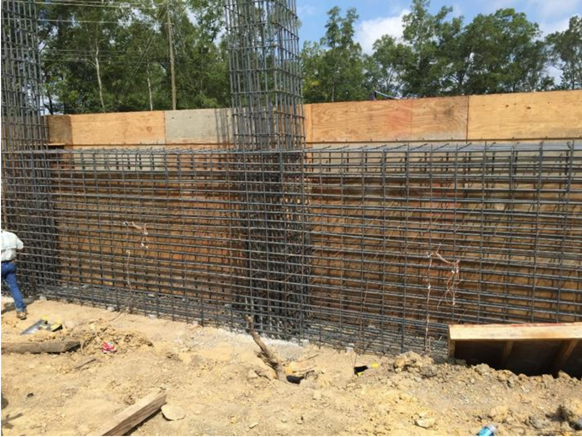
Figure 5-6: Harpersville crashwall under construction
