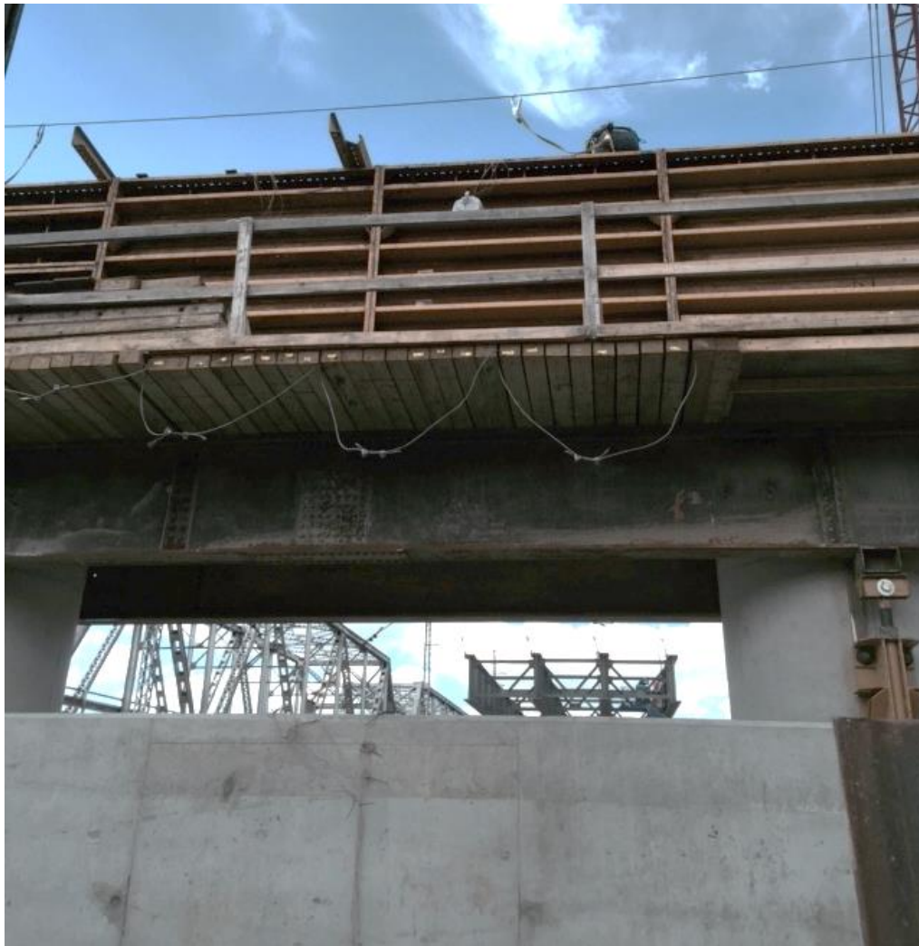
Figure 5-25: Scottsboro bent cap under construction
