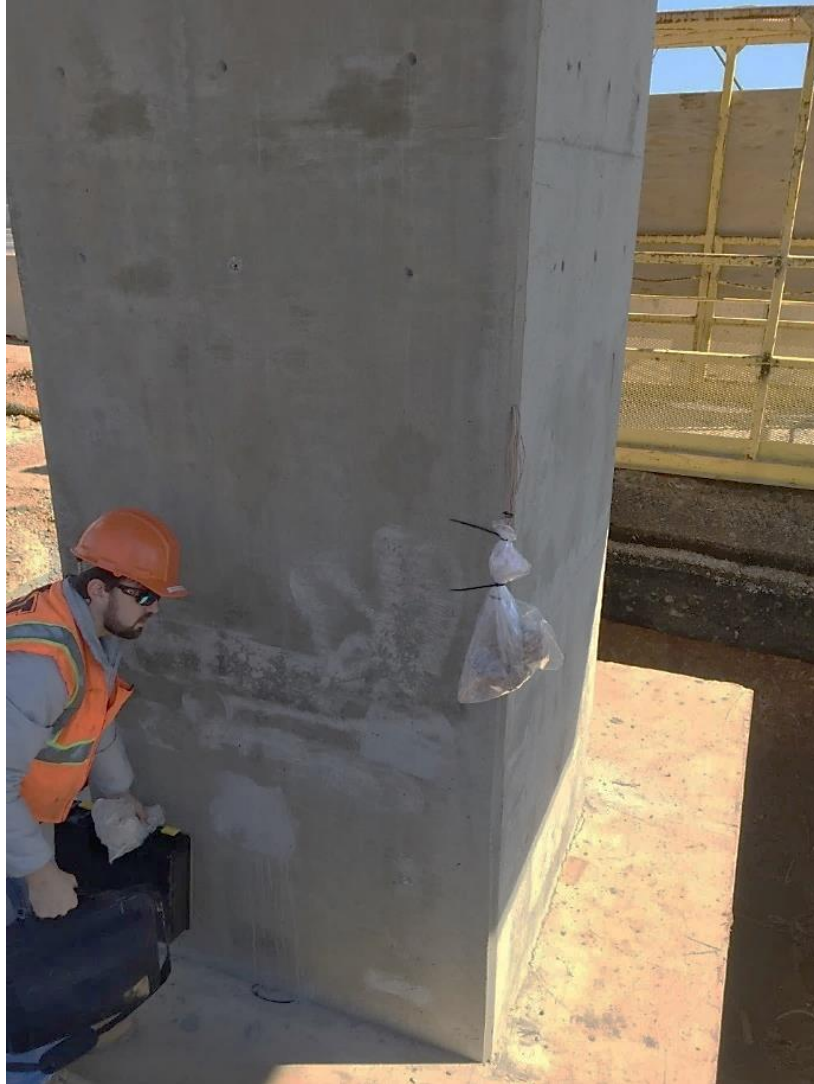
Figure 5-34: Birmingham column post construction with sensor lead wires visible
