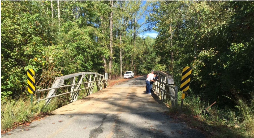
Figure 3-10: Replaced Bridge in Lee County
