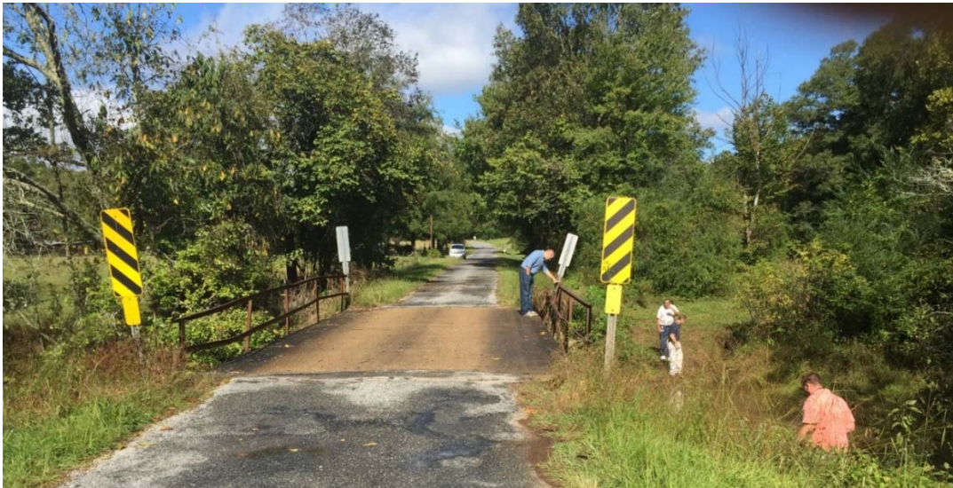
Figure 3-19: Replaced Bridge in Coosa County
