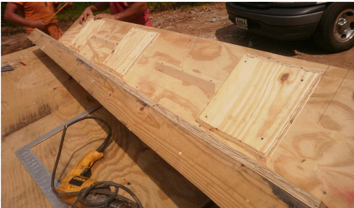
Figure 4-5: Formwork with block-outs for post installation
