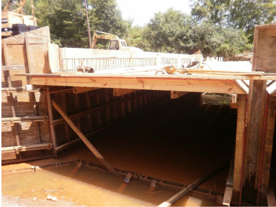
Figure 3-6: Formwork for northern half of elevated mat
