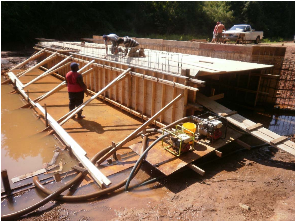
Figure 3-3: Workers construct formwork for southern end of culvert
