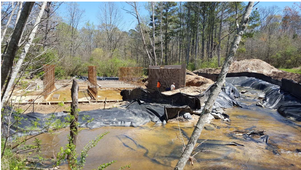
Figure 3-21: Workers construct formwork for barrels
