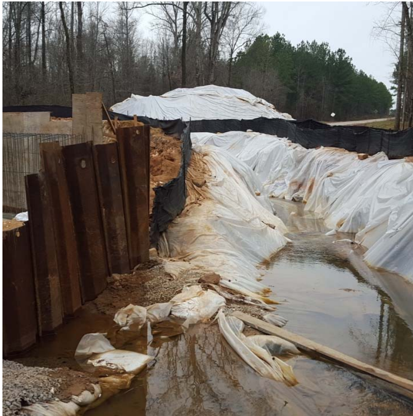
Figure 3-12: Water flow redirected
