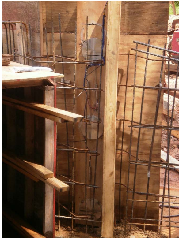
Figure 3-4: Formwork for embedded pressure cells
