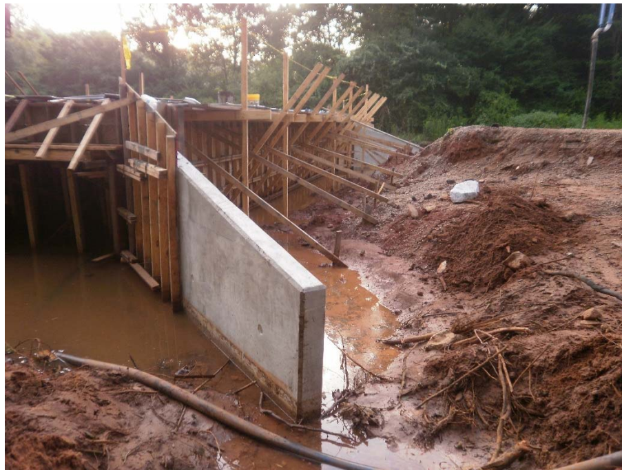
Figure 3-5: Southern wing wall formwork removed
