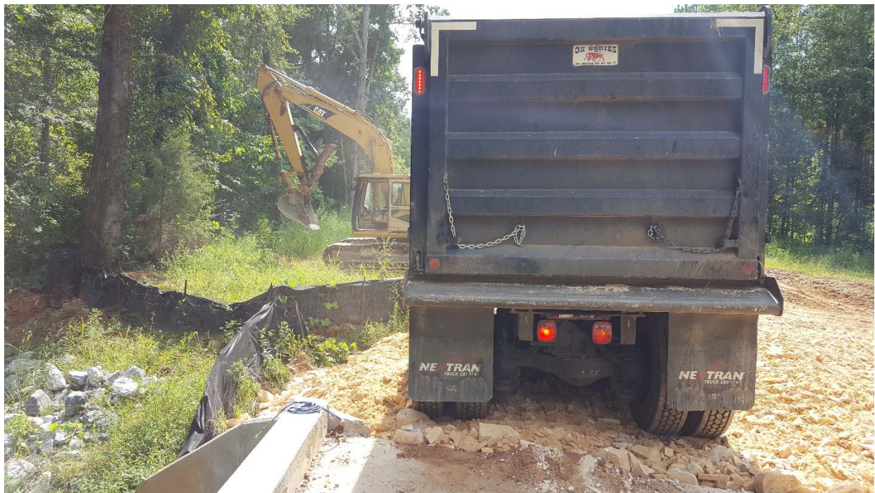
Figure 3-16: 40 ton truck placed near tab
