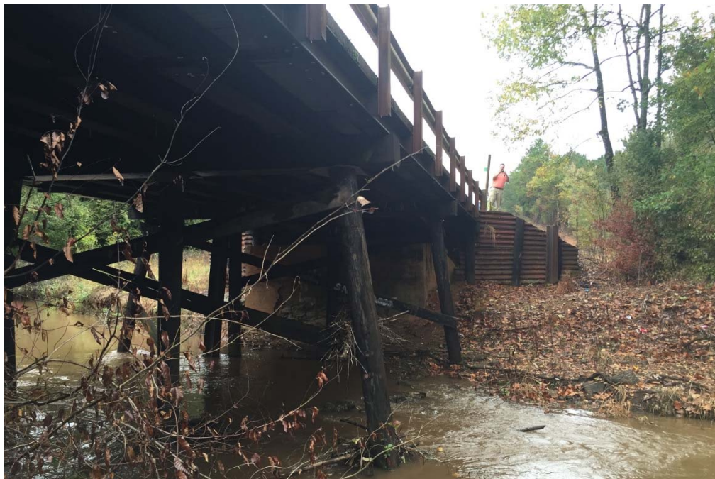
Figure 3-1: Replaced Bridge in Chambers County
