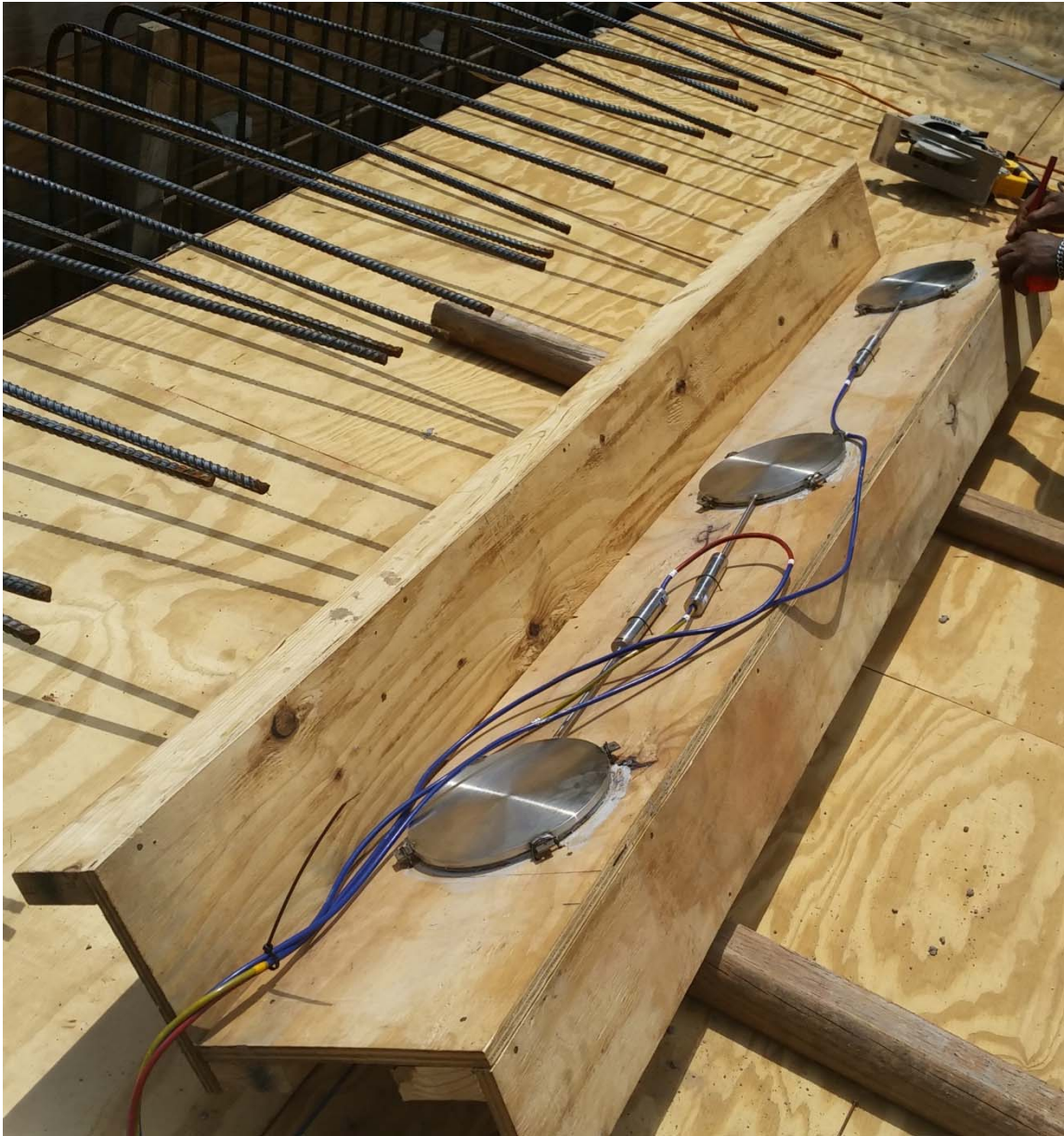
Figure 4-3: Formwork prepared for embedded installation of pressure cells
