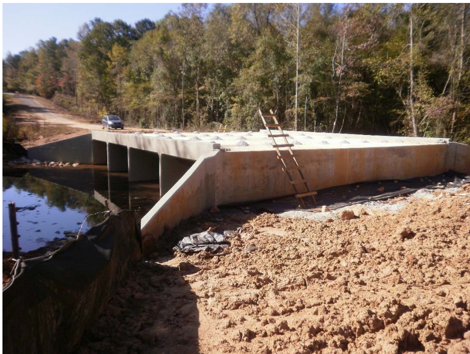
Figure 3-7: All formwork removed
