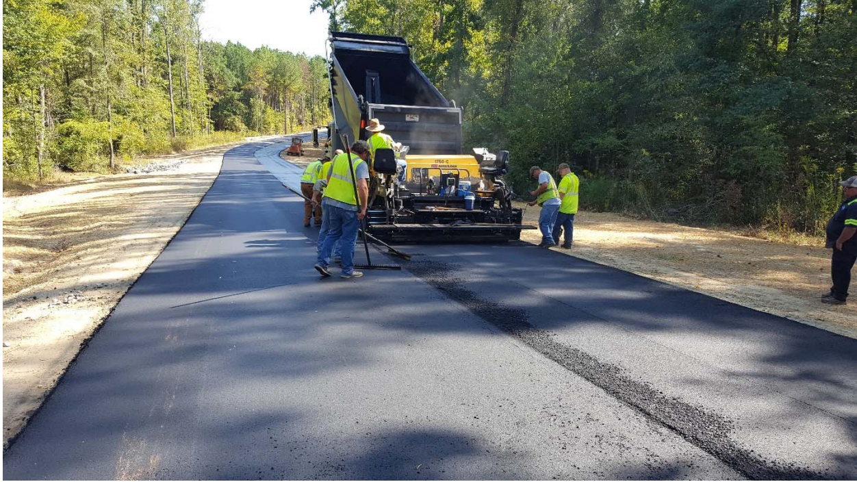
Figure 3-17: Culvert in process of being paved
