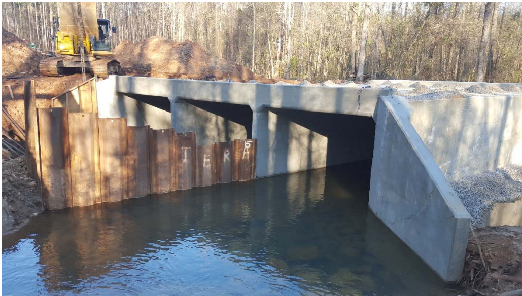
Figure 3-14: Water flow redirected to construct western wing walls
