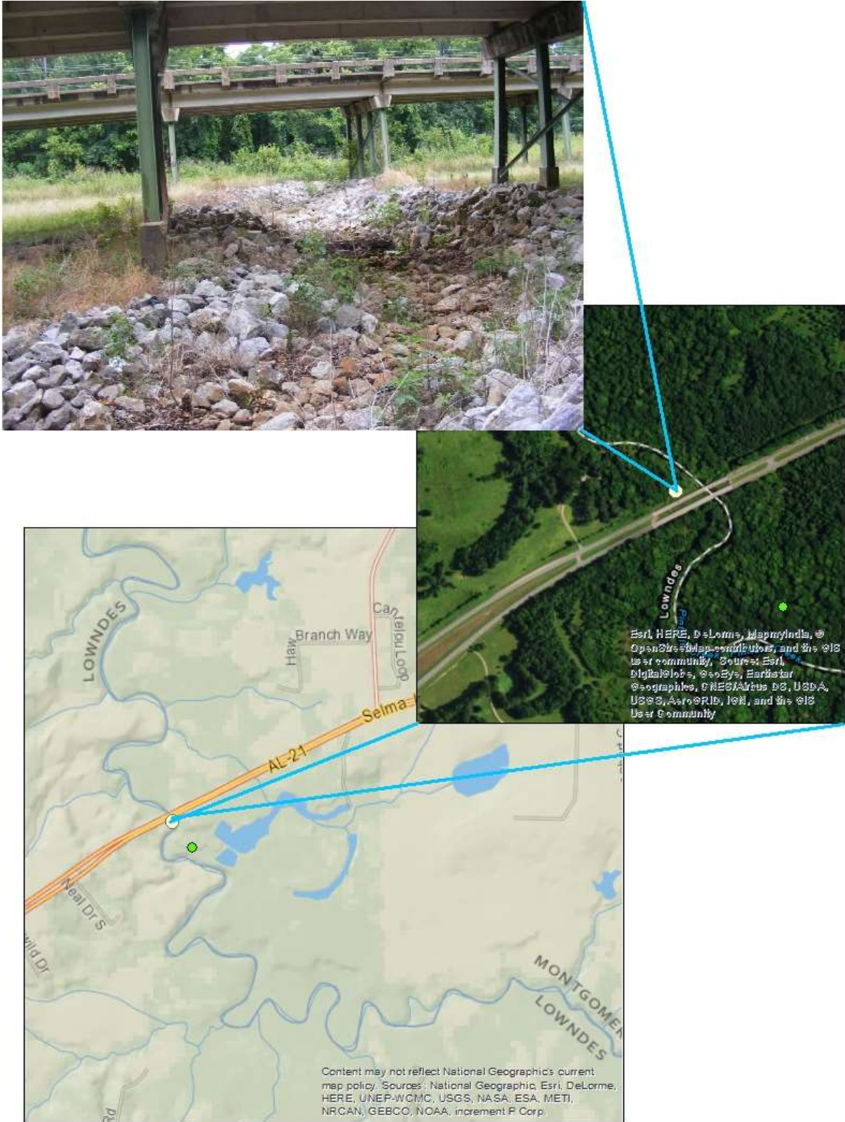
Figure 4.3 Location of Pintalla Creek and bridge site characteristics.
