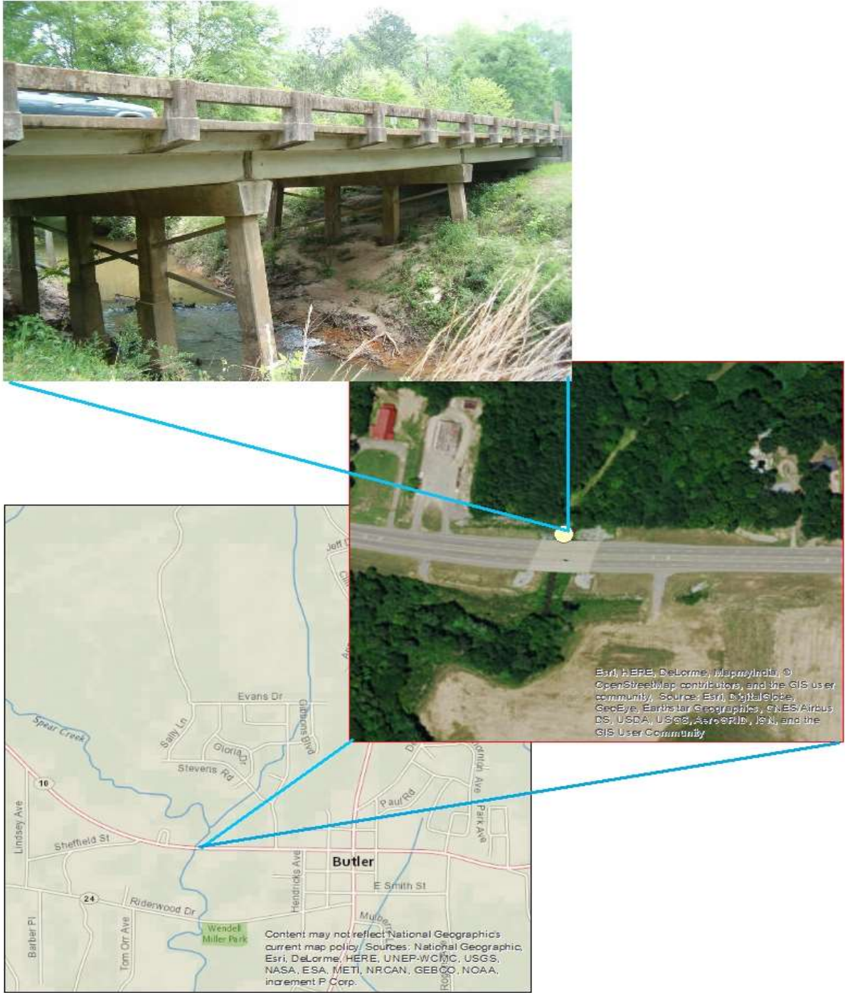
Figure 4.1 Location of Spear Creek and bridge site characteristics.
