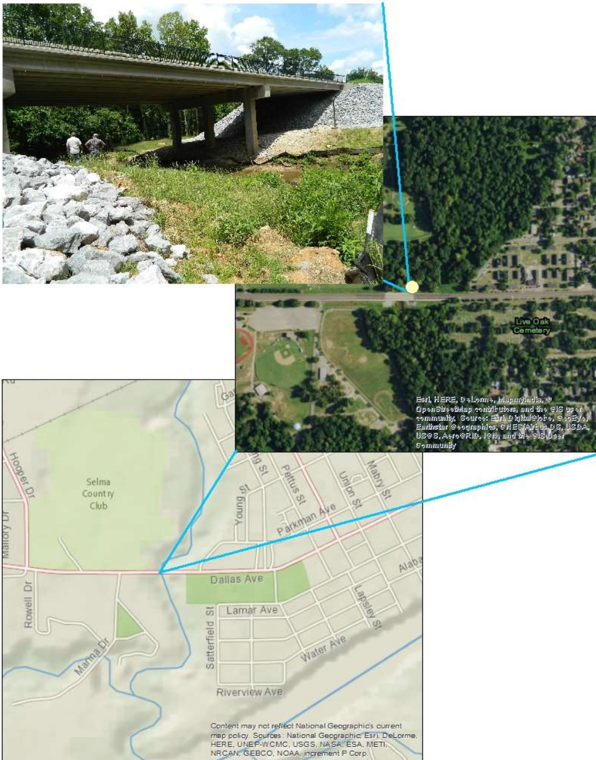
Figure 4.2 Location of Valley Creek and bridge site characteristics.
