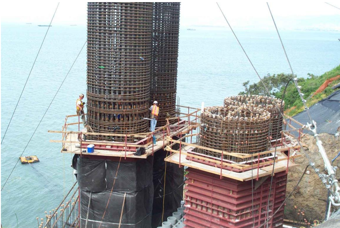
Figure 1-1: Mass concrete column under construction (Courtesy: PCA 2007)
