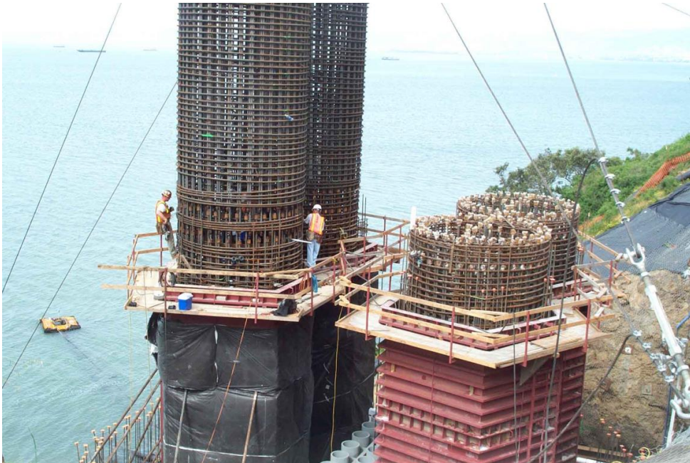
Figure 8-1: Mass concrete column under construction (Courtesy: PCA 2007)
