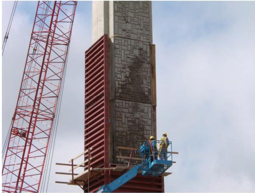
Figure 10-3: Rectangular column formwork removal (Riding et al. 2017)
