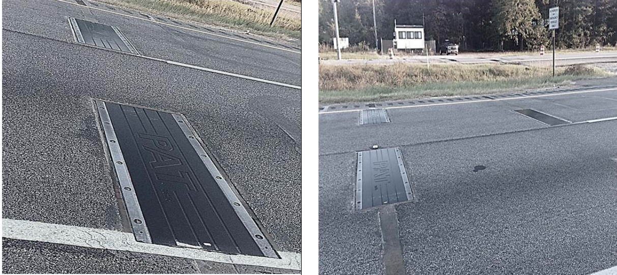
Figure 0-1. Bending Plate Systems in WIM Location 965 (Shorter, I-85)
