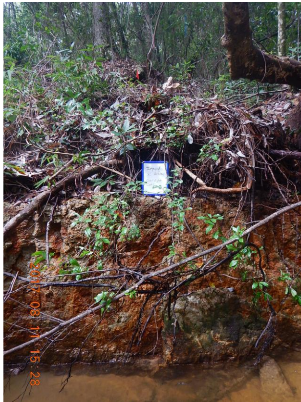
Figure 30: Example of bank incision at the impaired site. This type of incision is common in urban areas and is associated with hydrologic changes related to impervious surfaces (i.e. stream flashiness).
