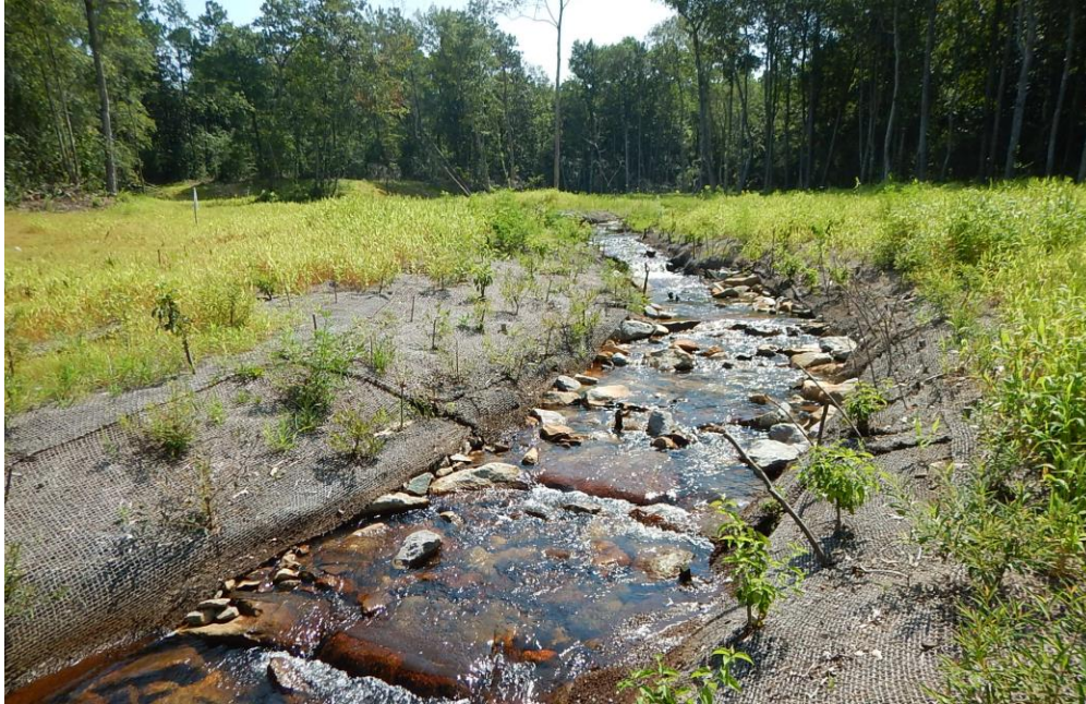
Figure 7: The use of rock material (e.g. boulders) and riparian vegetation to modify flow dynamics at the restored site, following a hybrid natural channel design and modified hydraulic design method (Rosgen, 1994).
