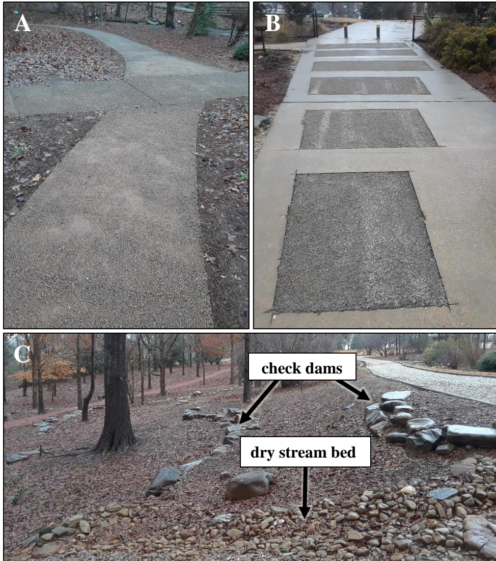
Figure 32 A, B, and C: BMP examples at the Donald E. Davis Arboretum, Auburn University A) Pervious concrete sidewalk; B) Pervious concrete inserted into an impervious concrete sidewalk; C) BMP apparatus installed across the landscape to mitigate runoff before it enters a downhill stream.
