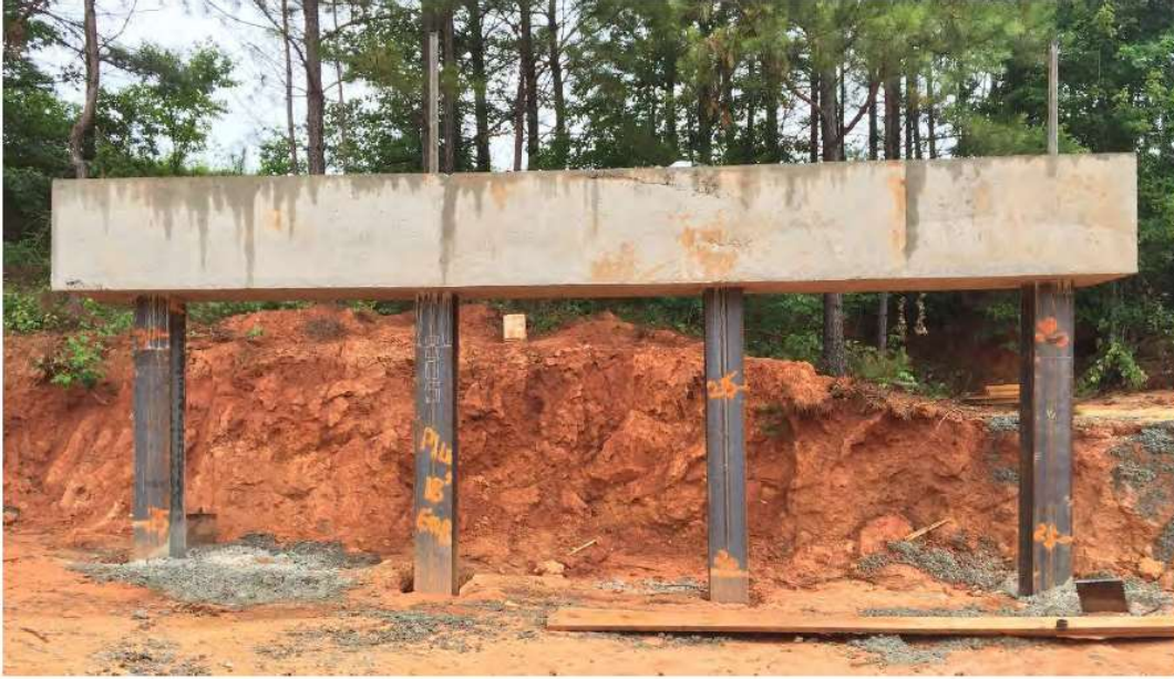
Figure 19. Vertical bent, taken from south to north (Marshall et al. 2017).
