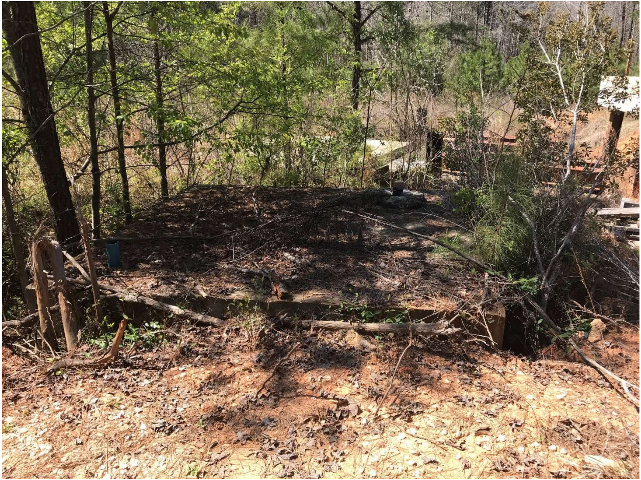
Figure 8. Photo of the 5-pile group looking from east to west taken in March 2018.
