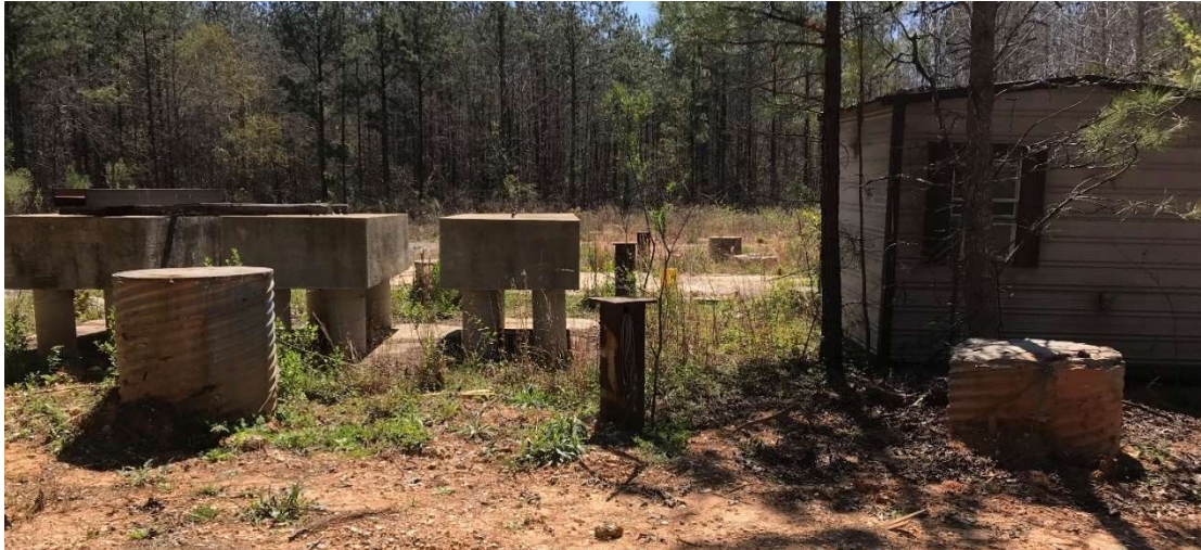
Figure 16. Photo of drilled shafts looking from north to south taken in March 2018.
