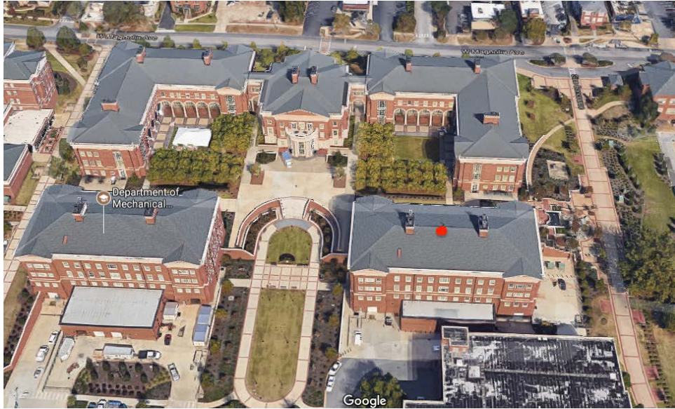
Figure 4.3: Overhead View of Antenna of Roof of Woltosz.
