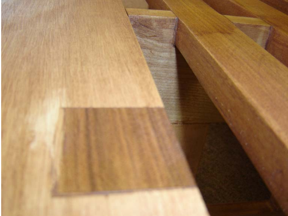
Top of dovetail joint in desktop surface.
