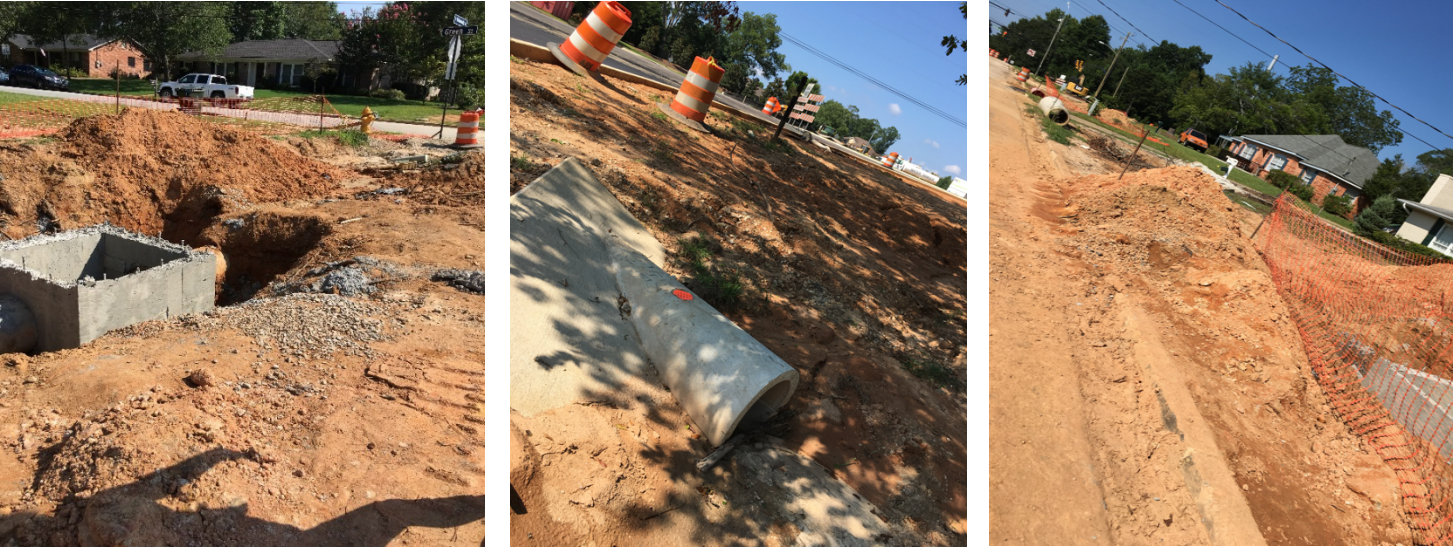
Fig. A1. Construction sites within the Moore's Mill Creek watershed
