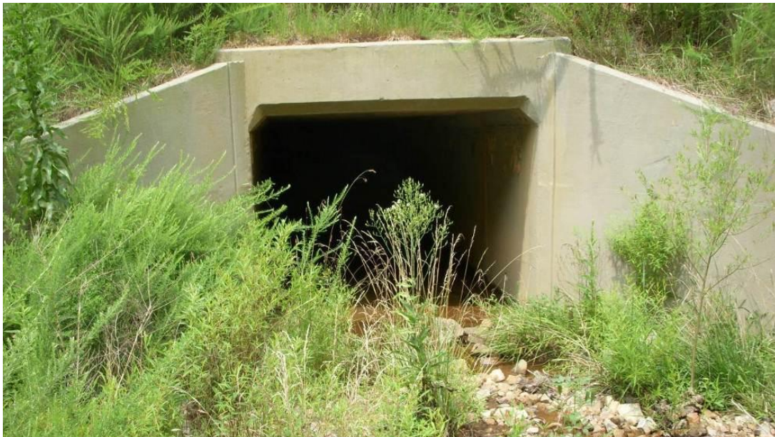
Figure 10-1 AEB Culvert at 175+70 Entrance (Minton 2012)
