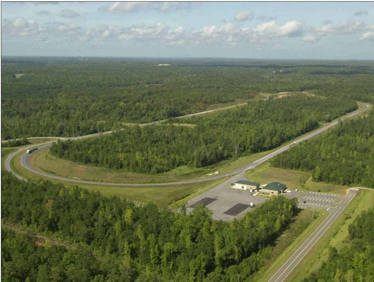
Figure 3.1 NCAT Pavement Test Track
