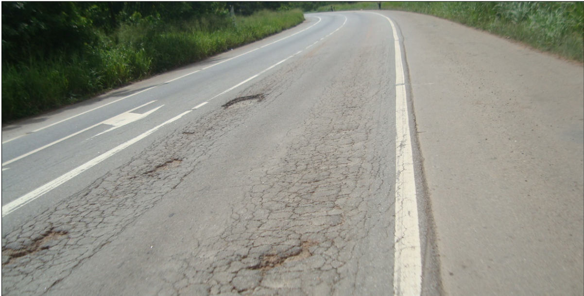
Figure 1.1 Bottom-up Fatigue Cracking
