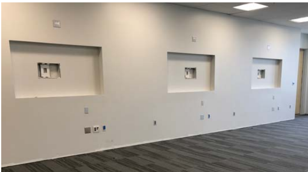
Figure 22. Recess in secondary wall for venting heat load.
