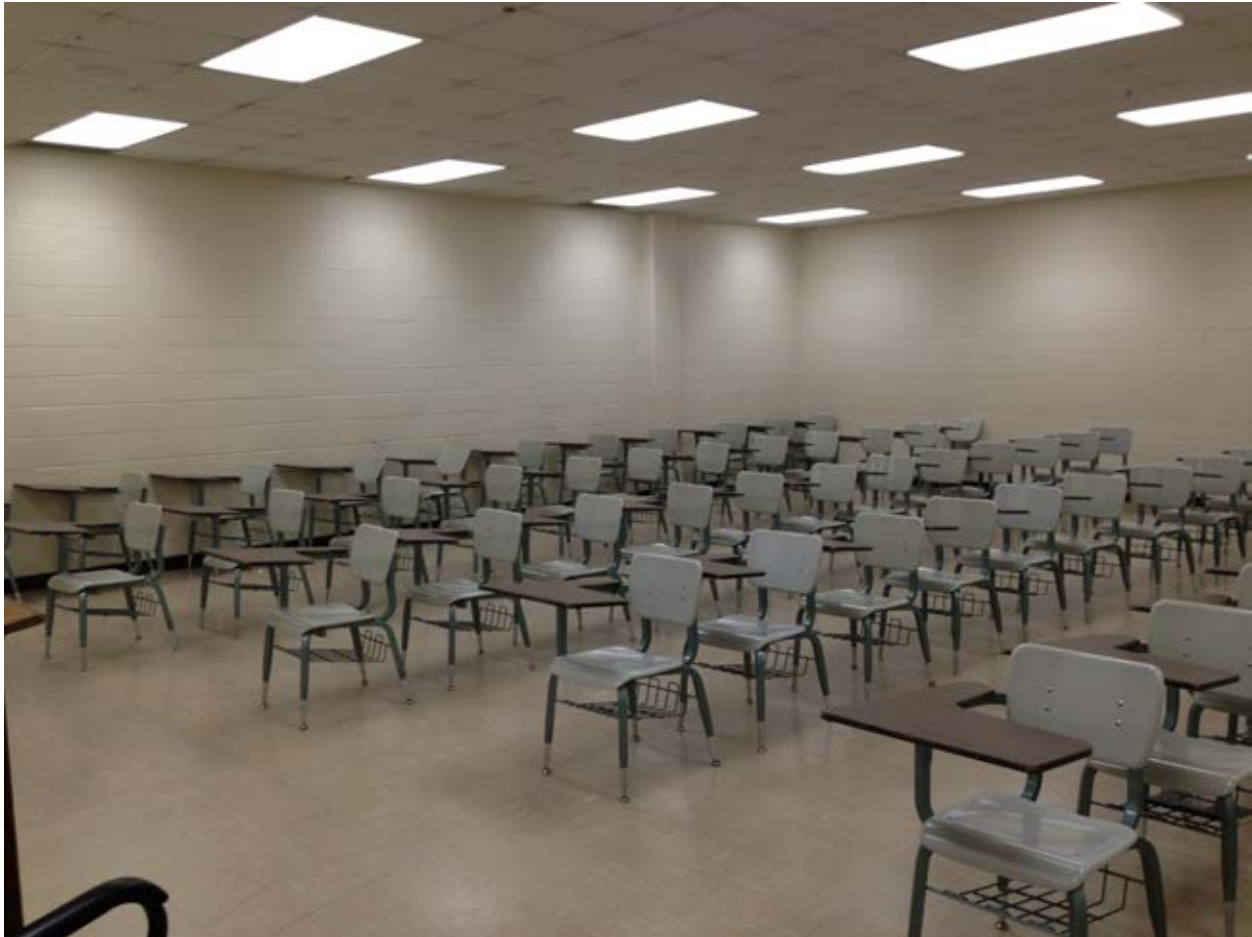
Figure 5. Haley Center 2213 Existing Conditions
