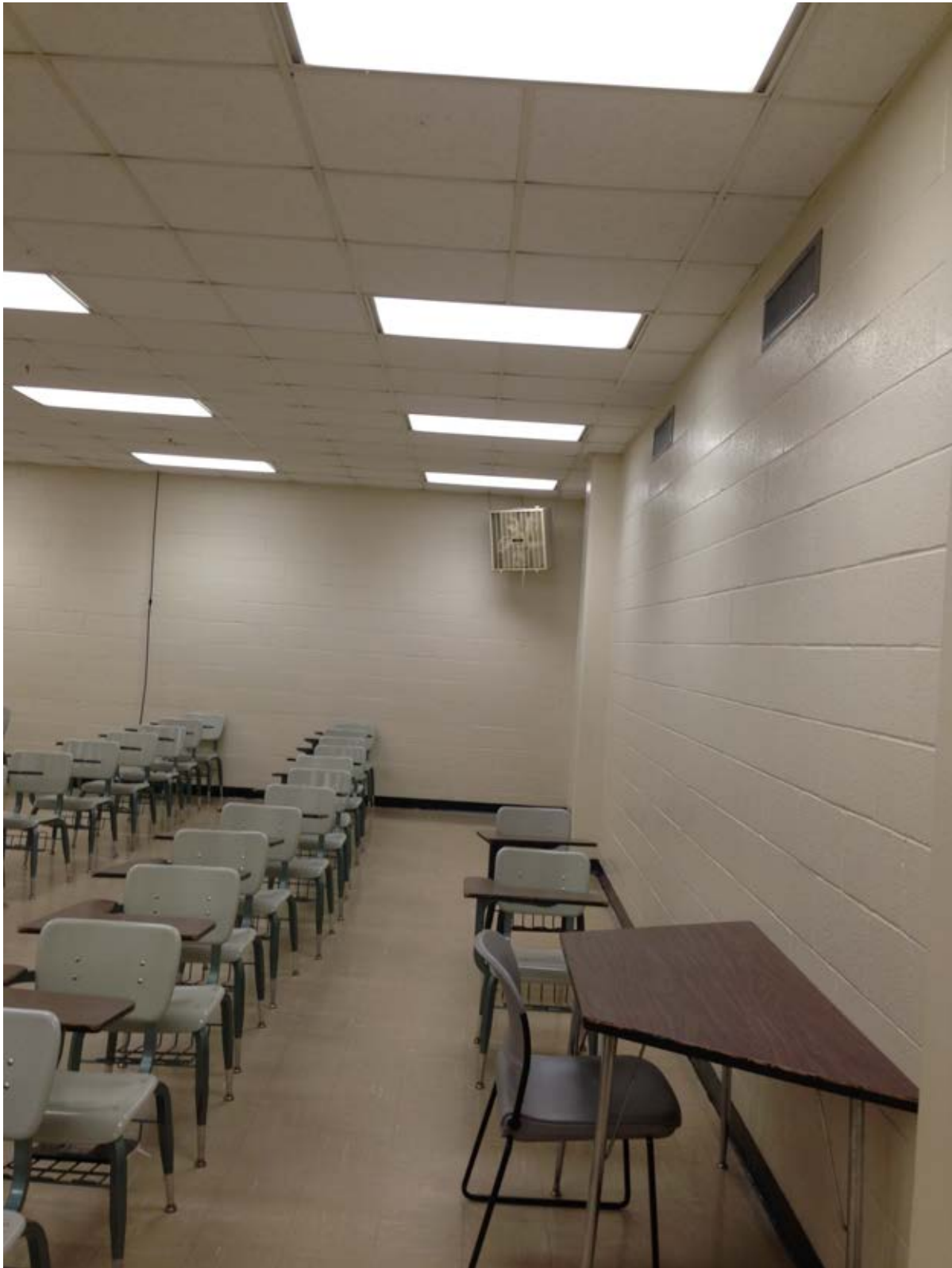
Haley Center 2213 Existing Conditions Photo – 3/20/13
