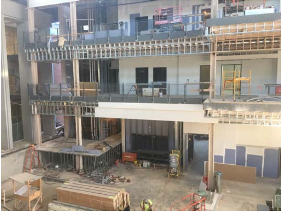
Mell Classroom Building 118 Construction Photo – Public Gathering Space – 3/9/17
