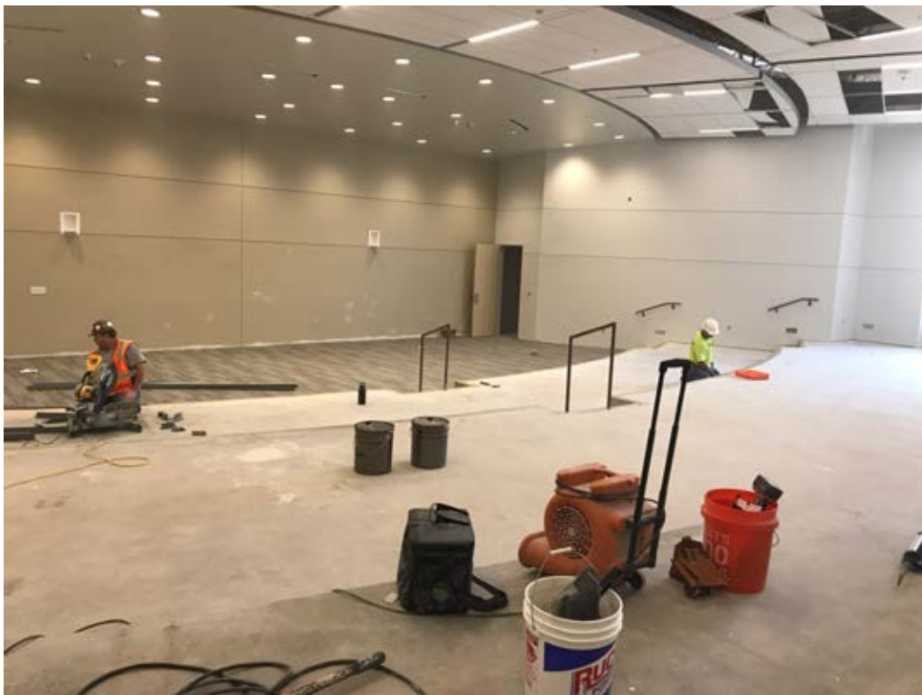
Mell Classroom Building 118 Construction Photo – Lecture Hall – 3/9/17
