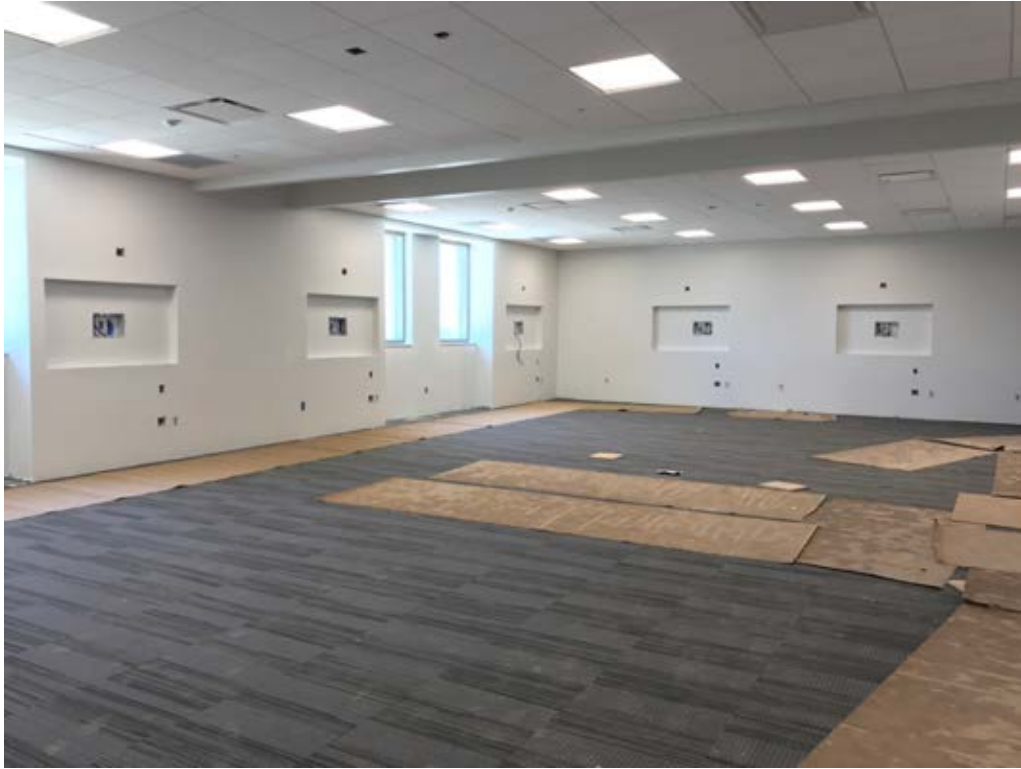
Mell Classroom Building 118 Construction Photo – Classroom – 3/9/17
