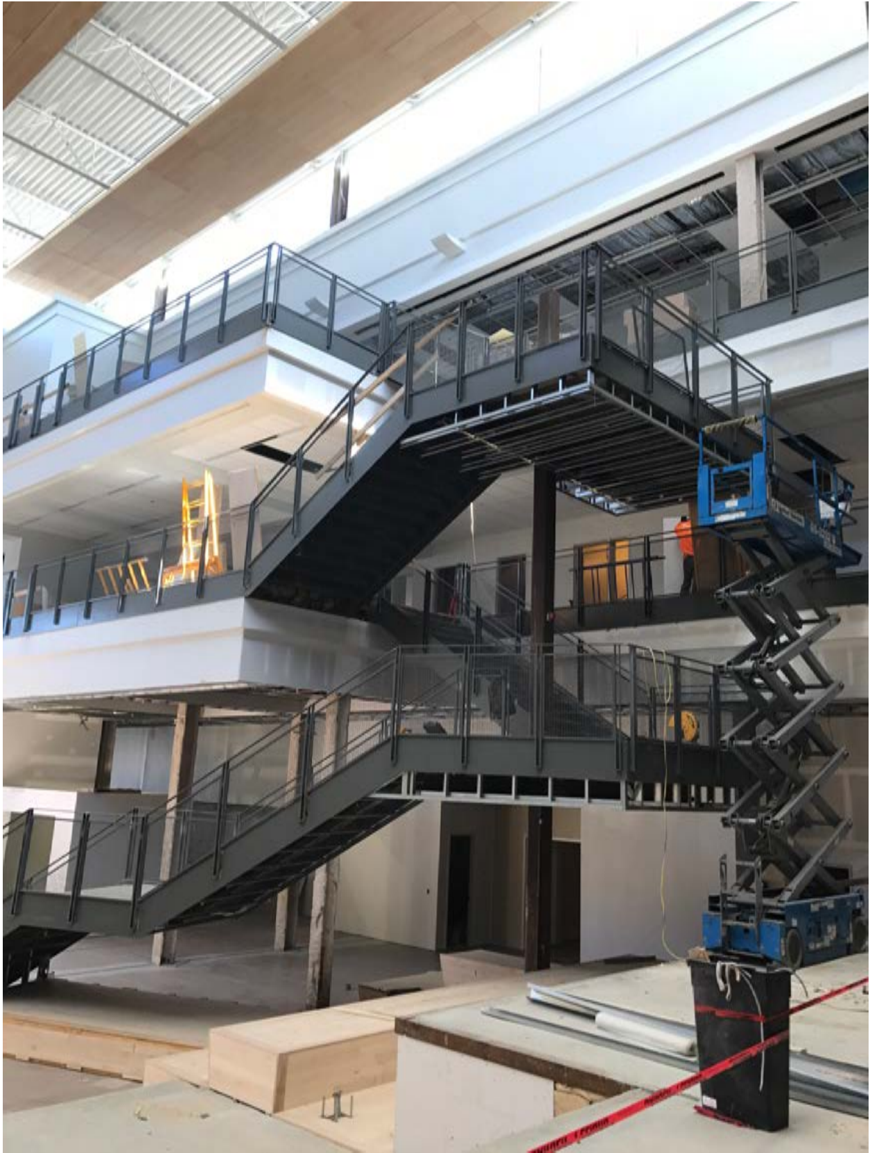
Mell Classroom Building 118 Construction Photo – Public Gathering Space – 3/9/17
