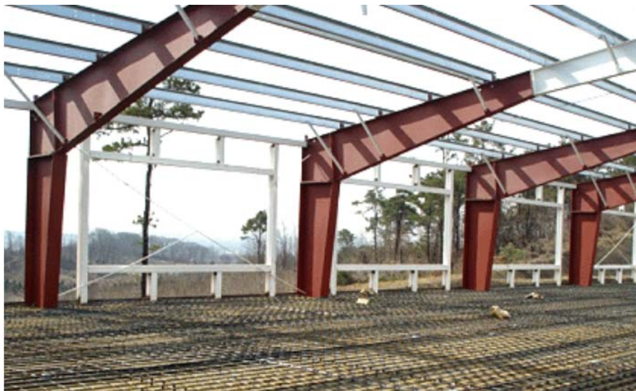
Figure 2-2. Metal Building Frame with tapered webs under construction (Stuart 2013)
