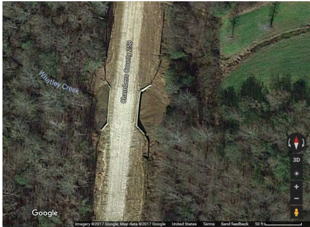
Figure 3-4. Location of Chambers County culvert (“Google Maps” 2017a)
