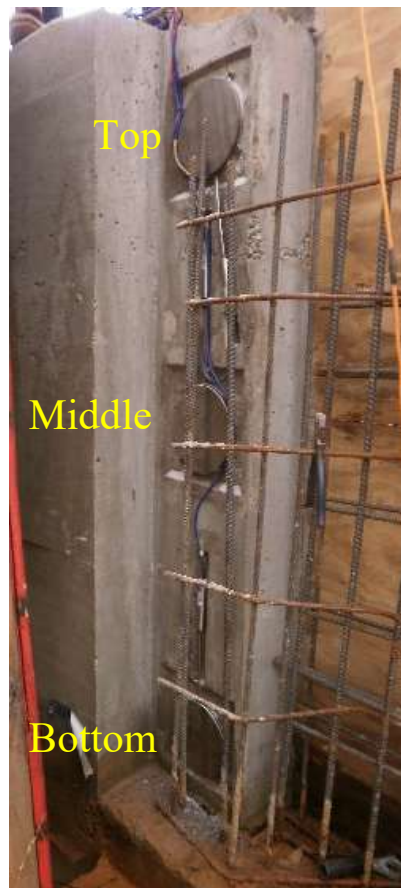
Figure 5-3. Post installed pressure cells (Lee 2017)
