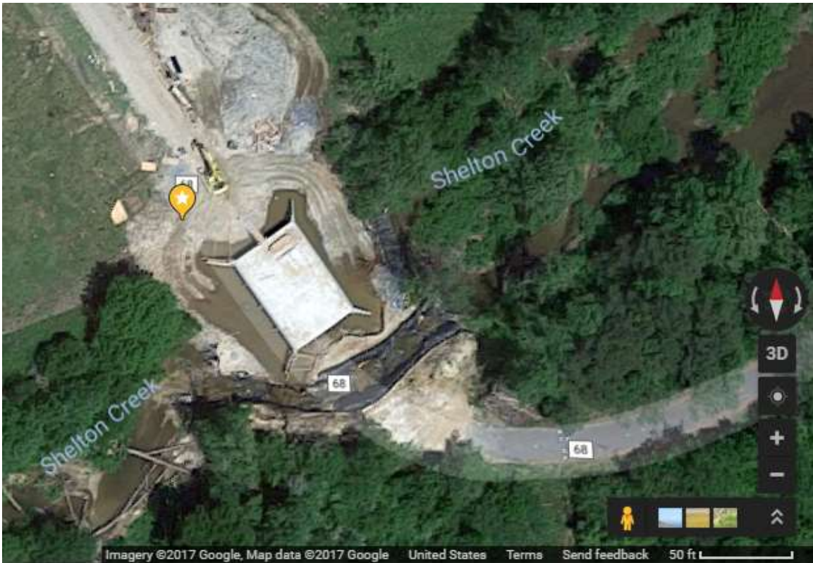
Figure 3-8. Location of Coosa County culvert (“Google Maps” 2017c)
