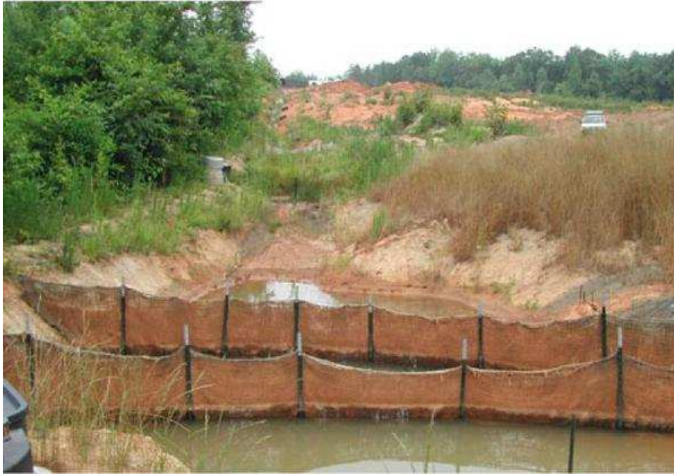
Figure 2.6: Jute/coir baffles in a basin (McLaughlin, 2015b).
