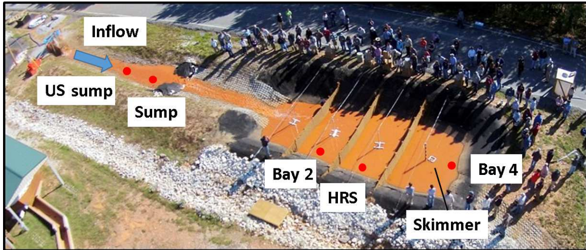
Figure 6.1: Aerial view of the sediment basin facility (Perez et al. 2016).
