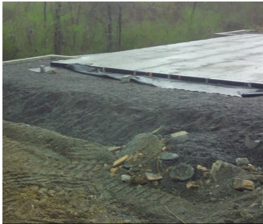
Figure 25: Placed bridge beams and the integrated approach.
