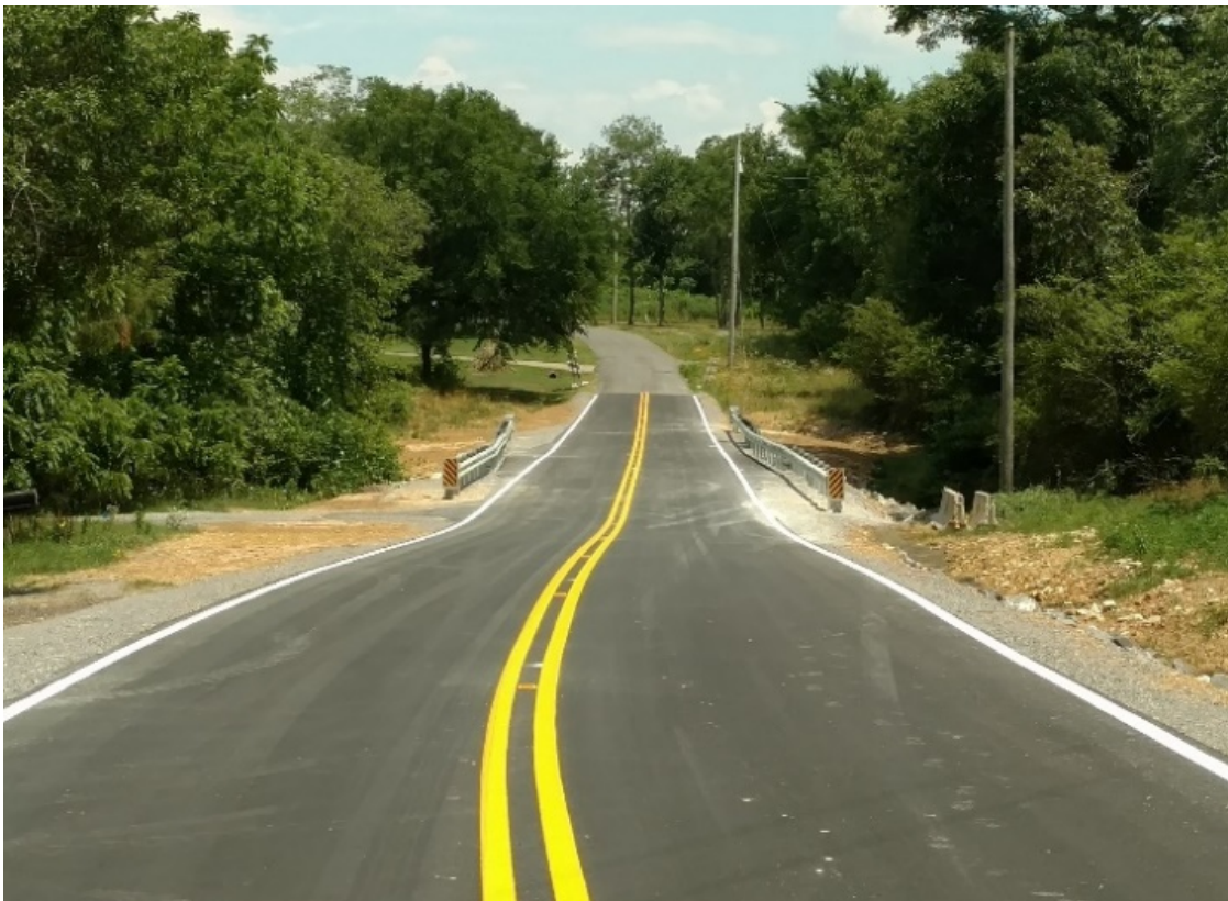
Figure 26: The completed GRS-IBS over Turkey Creek in Marshall County, AL.
