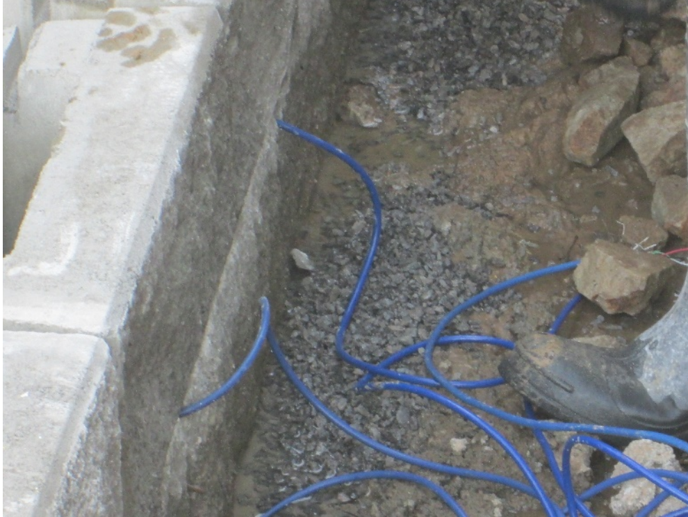
Figure 31: Sensor cables routed through chiseled openings in the SRW units.
