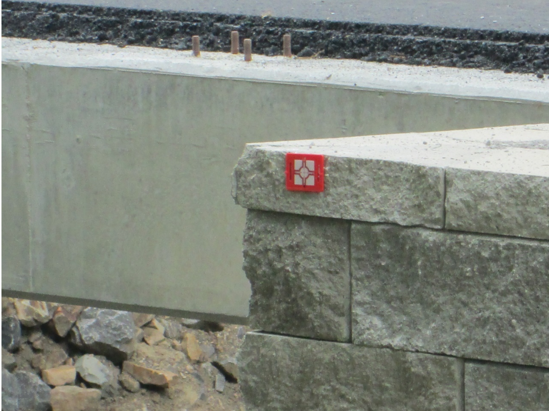
Figure 36: RS60 survey target mounted onto a GRS abutment.
