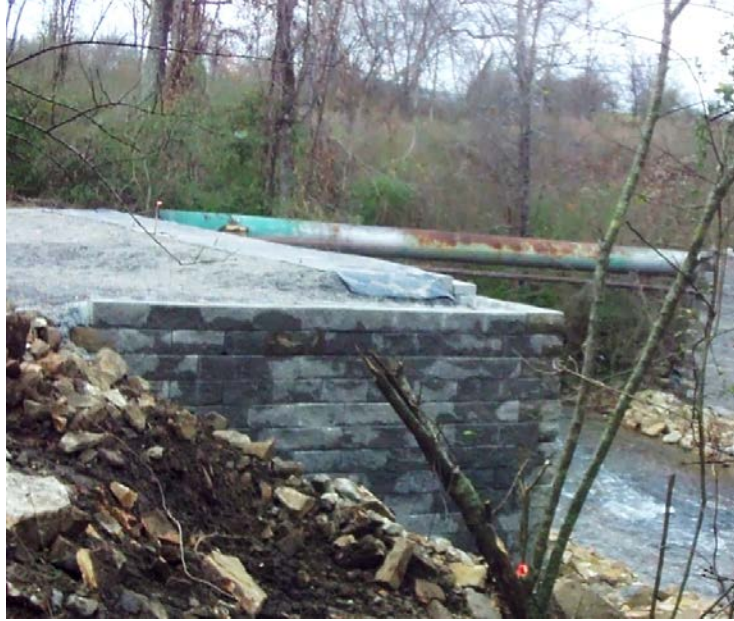
Figure 23: The finished GRS abutment prior to placement of the bridge beams.
