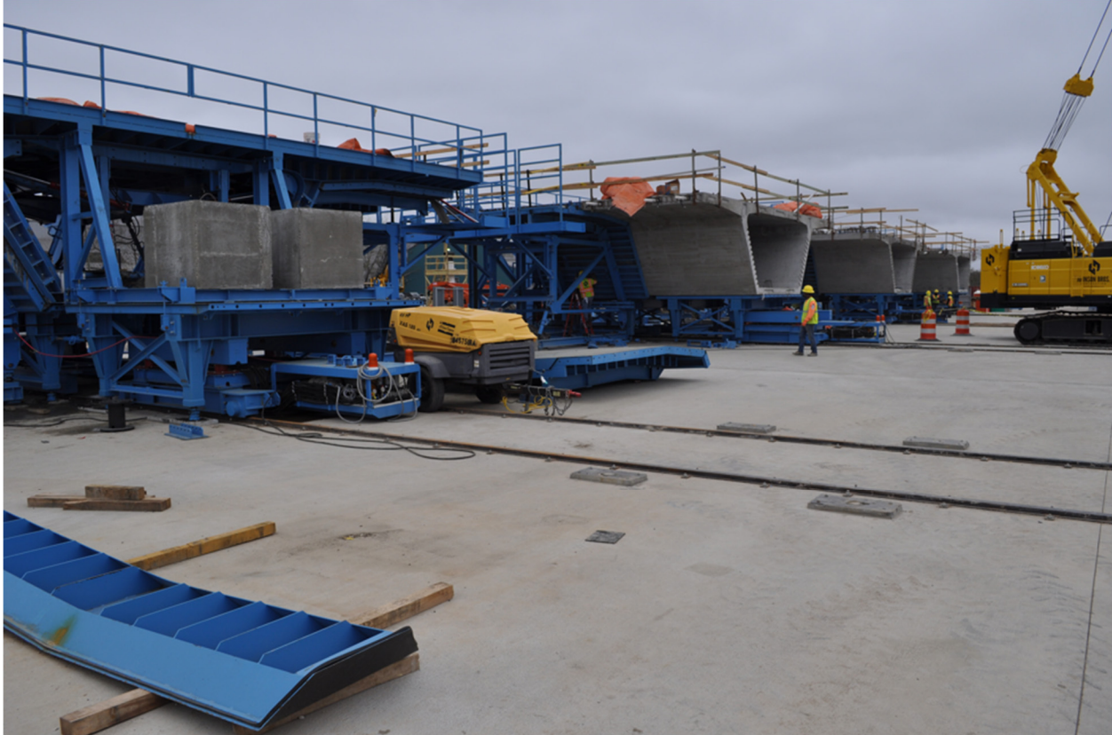
Figure 1-3: Formwork used during casting of concrete segments
