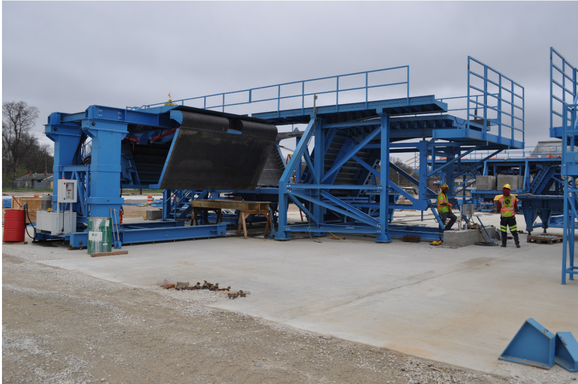
Figure 4-4: Hydraulic conveyor system used to slide each segment from the formwork
