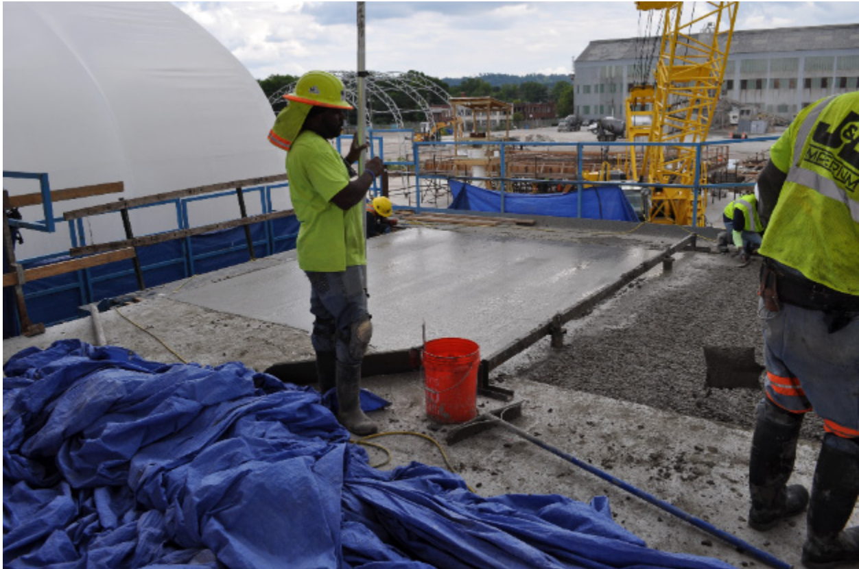
Figure 4-12: Float finishing of a concrete segment
