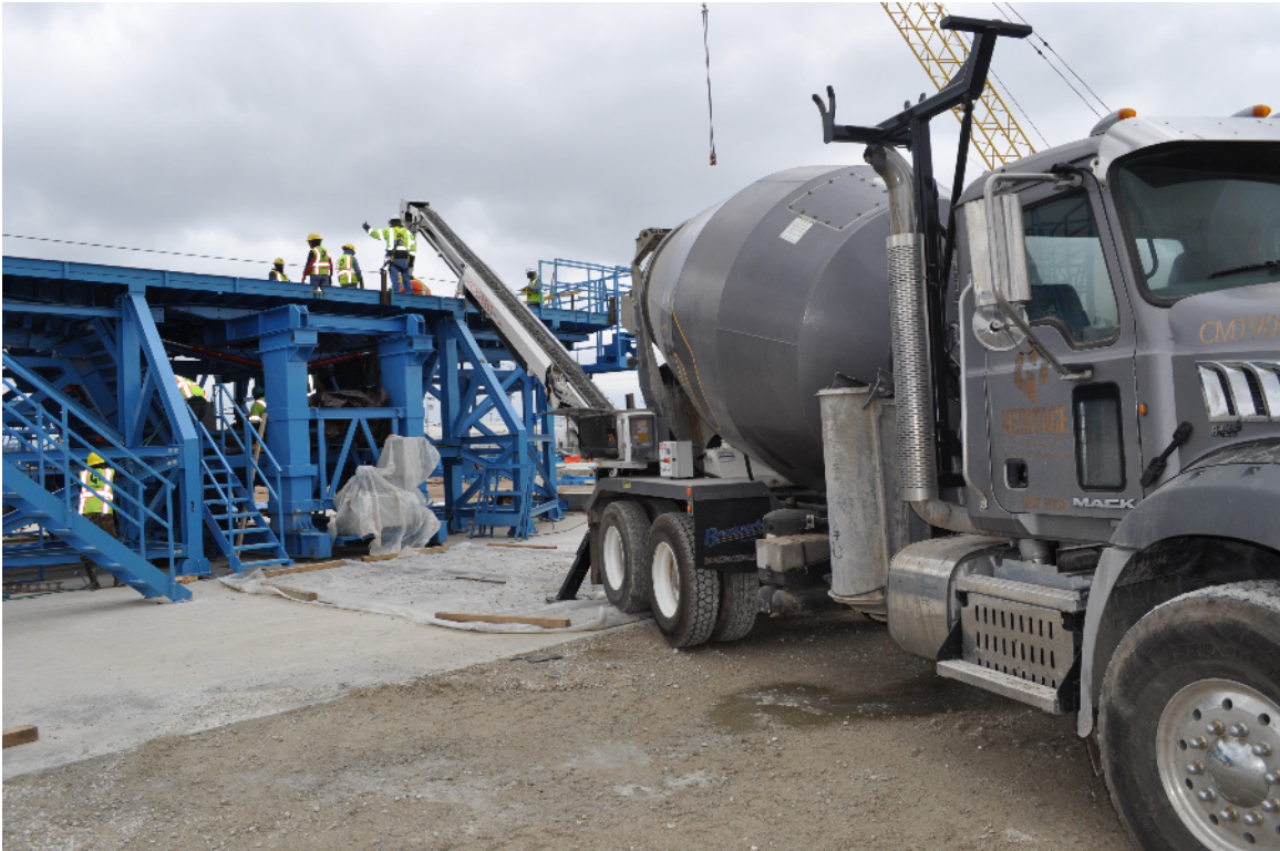
Figure 4-7: Ready-mixed concrete truck equipped with belt conveyor
