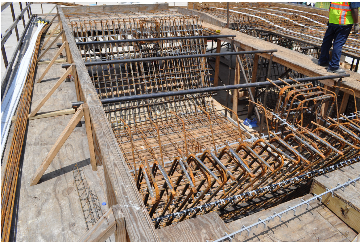
Figure 4-3: Pre-fabrication of steel reinforcement cage prior to being placed in formwork
