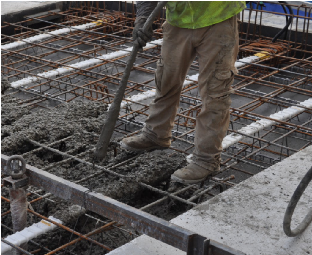
Figure 4-11: Portable vibrator used to achieve the desired consolidation
