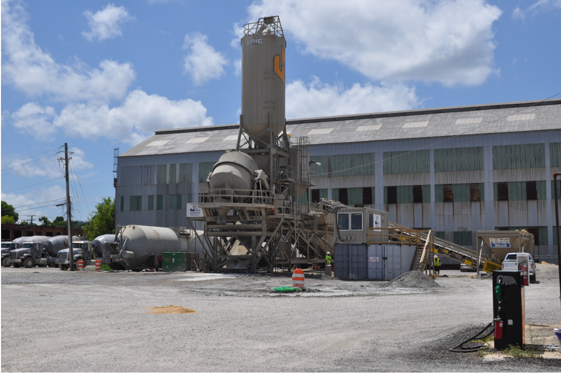
Figure 4-5: On-site batch plant for all mixing of concrete
