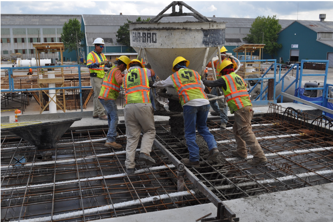
Figure 4-10: Placement of concrete by use of the concrete bucket
