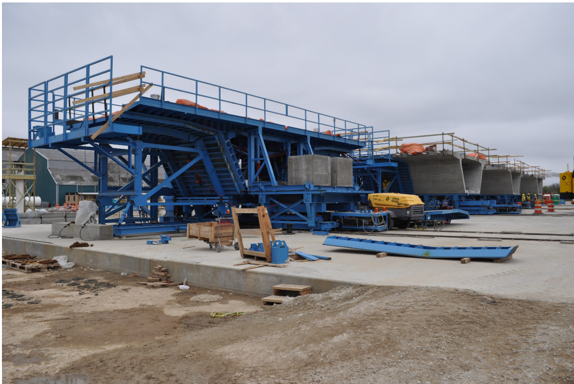
Figure 4-2: Segmental formwork used during casting
