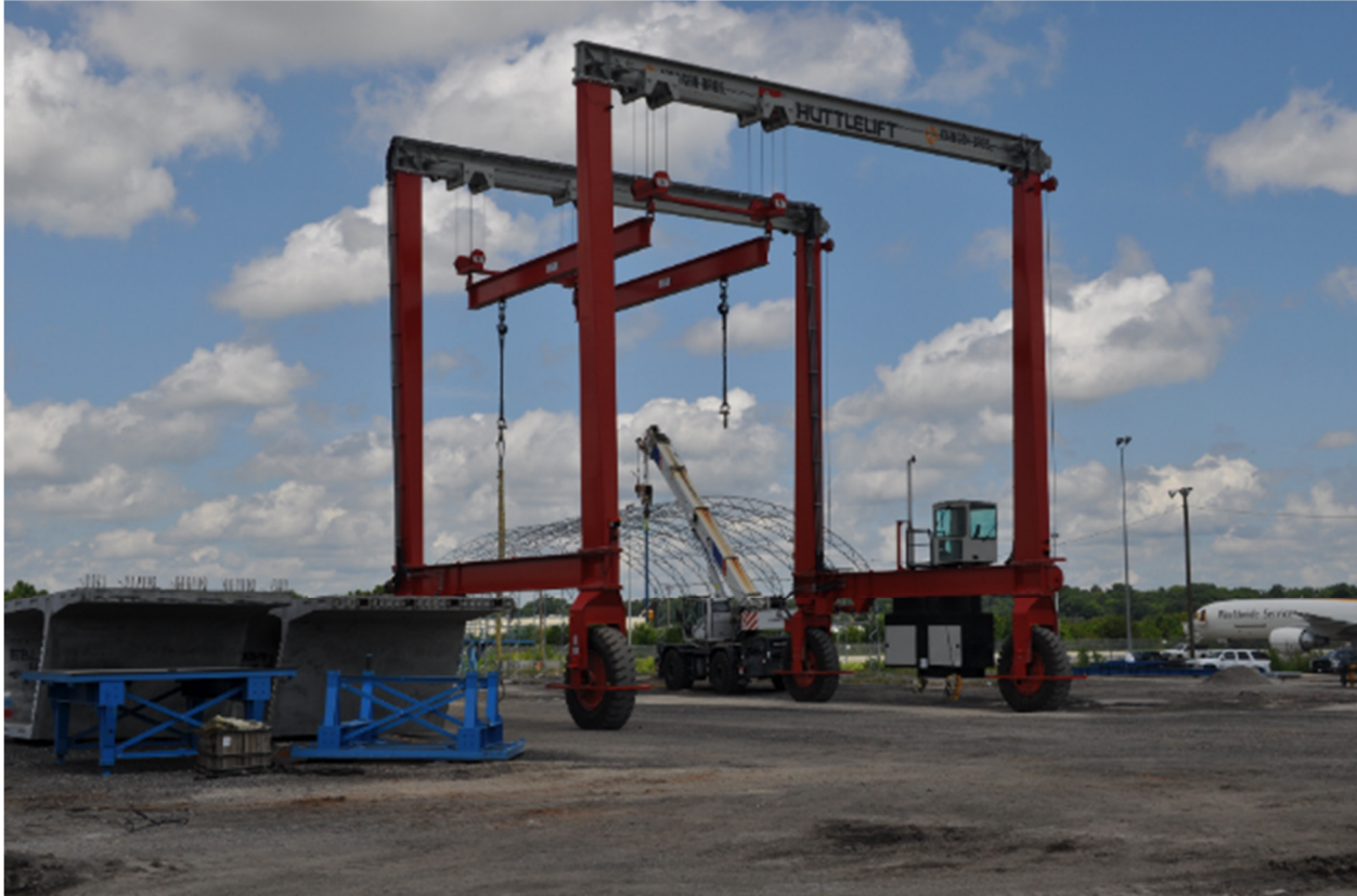
Figure 4-13: Crane used to transport segments to the storage yard
