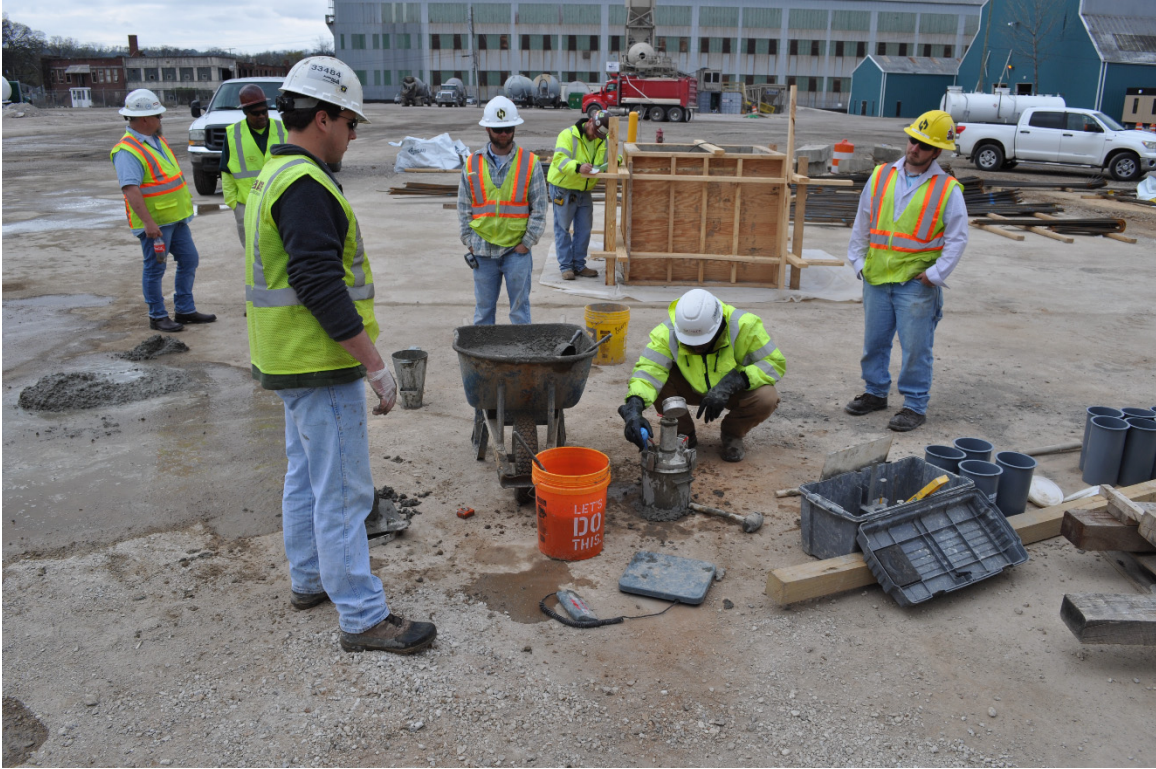
Figure 4-6: Quality control testing prior to placement of the concrete
