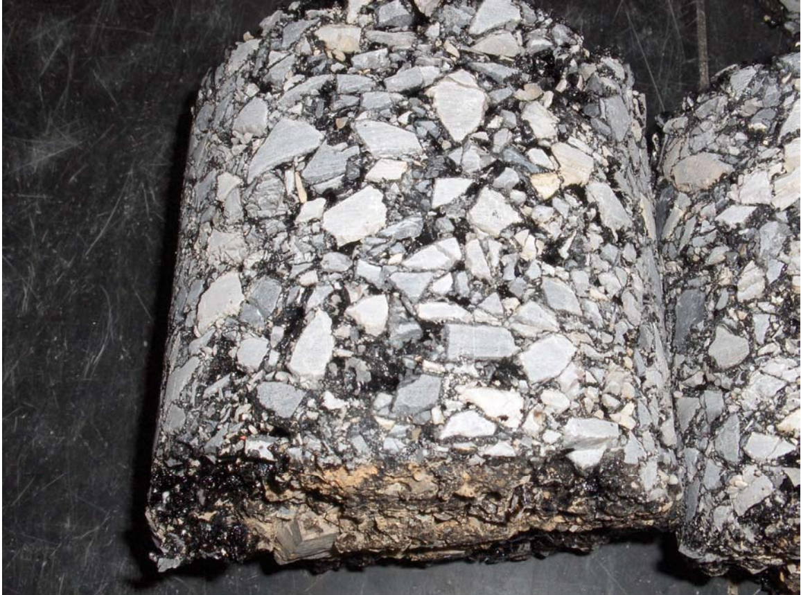
Figure 4.3. Core Obtained from Interstate 20 Construction Site.
