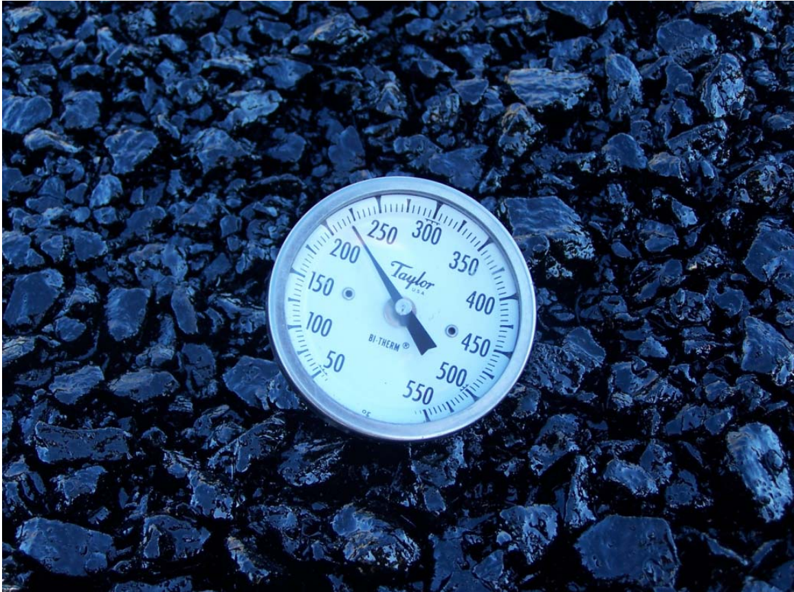
Figure 4.1. Temperature of Freshly Paved PATB on US 280.
