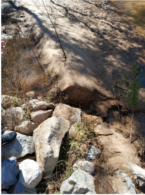
Figure 5.26: Aggradation signs on the east side of Soapstone Branch, downstream from temporary steel bridge
