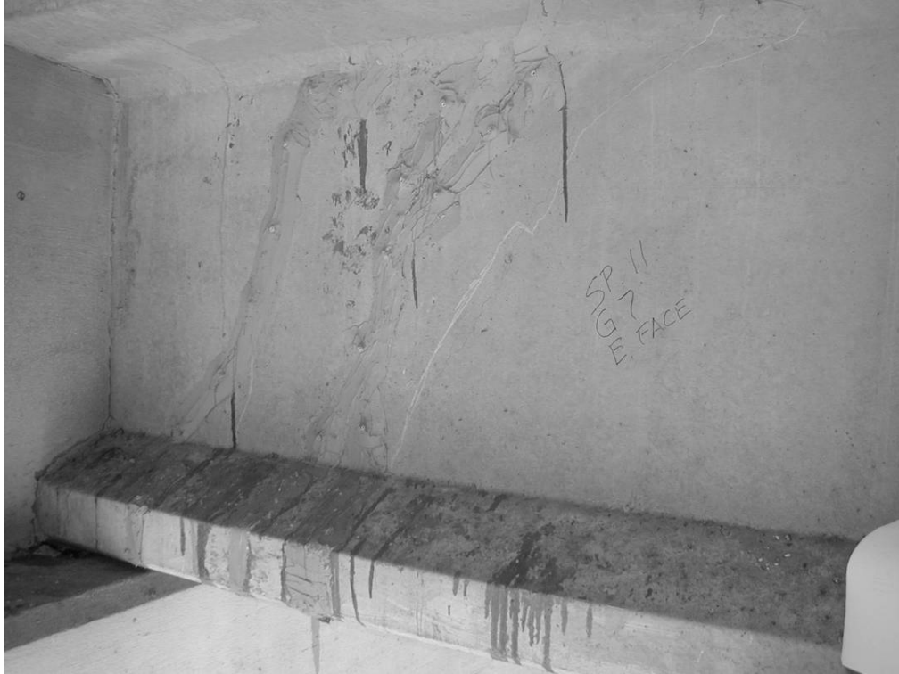
Figure 4.14 Girder 7 Span 11 East Face
