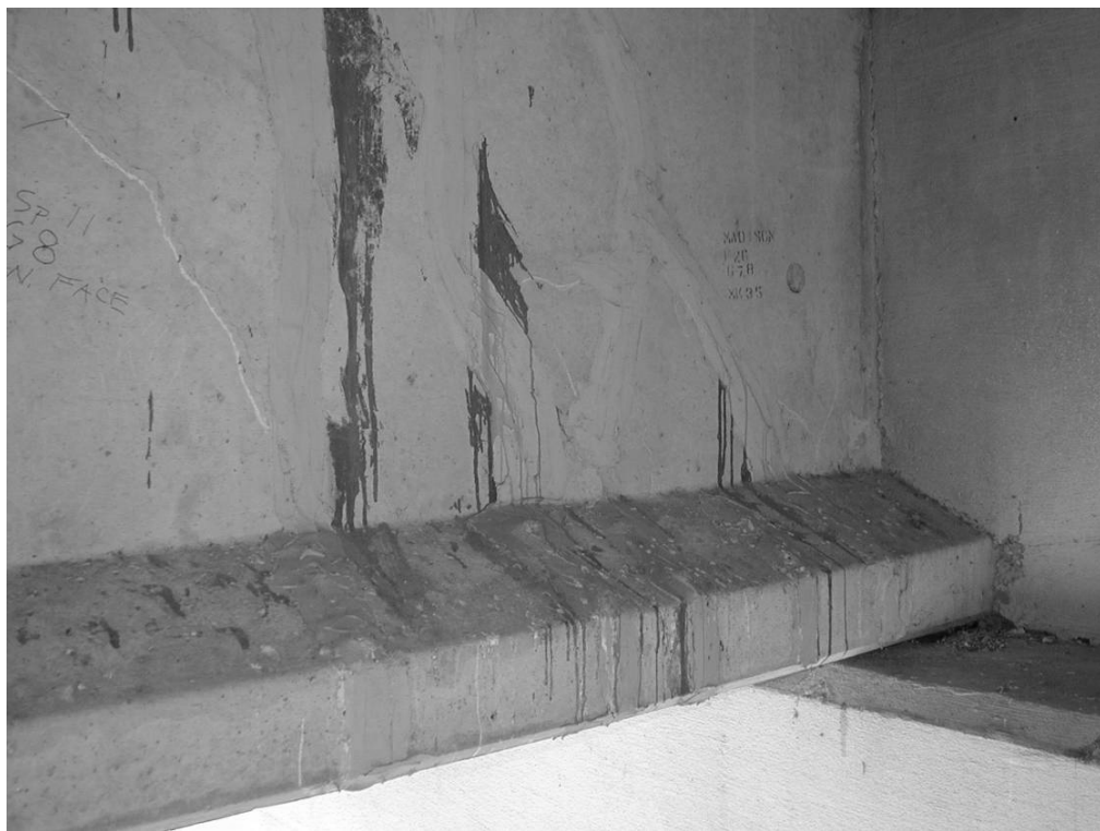
Figure 4.19 Girder 8 Span 11 West Face
