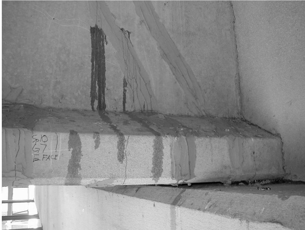
Figure 4.12 Girder 7 Span 10 East Face
