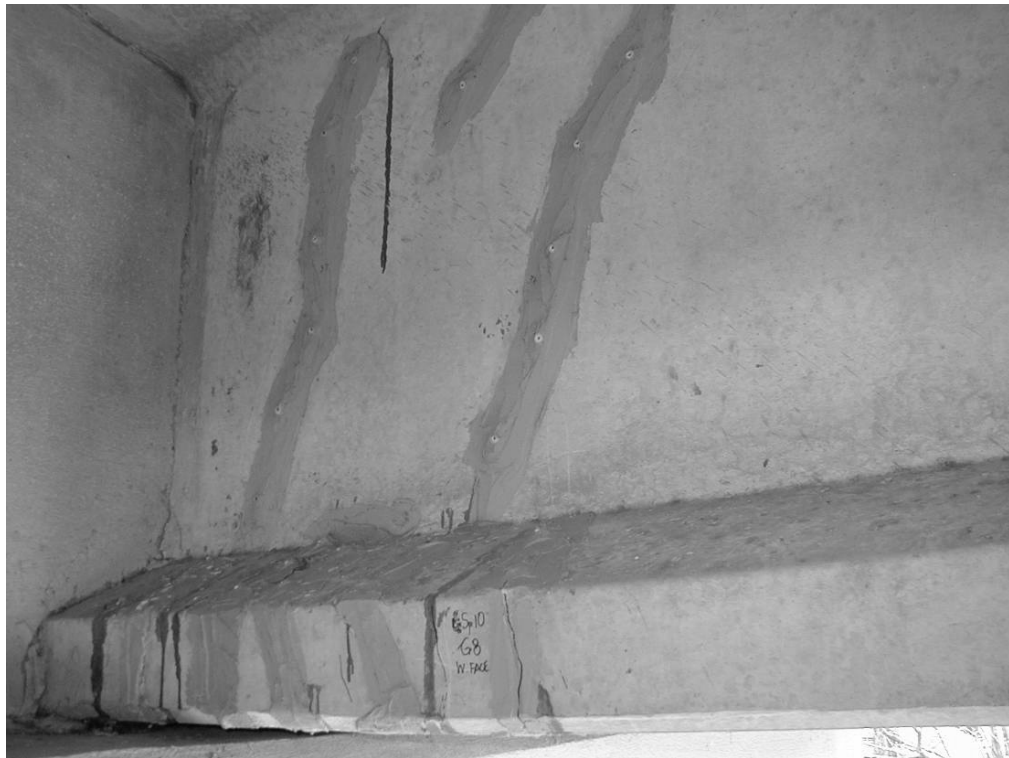
Figure 4.17 Girder 8 Span 10 West Face
