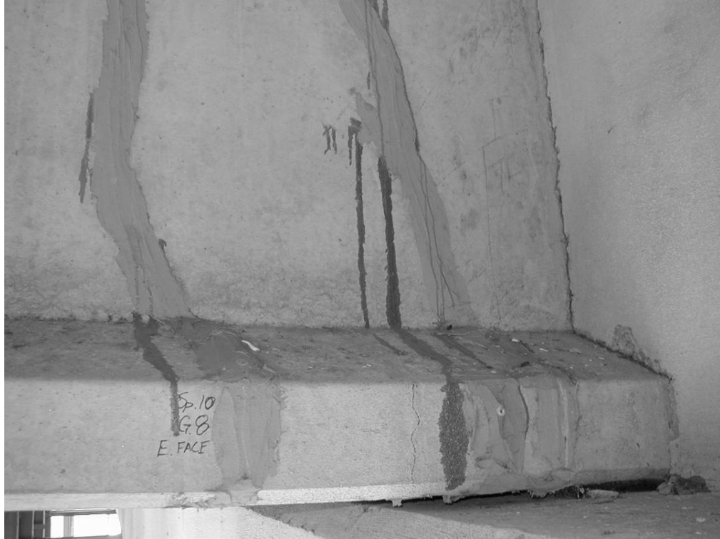
Figure 4.16 Girder 8 Span 10 East Face
