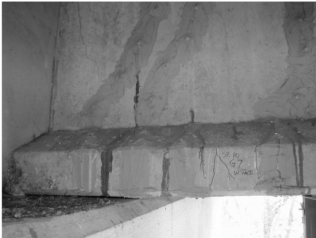
Figure 4.13 Girder 7 Span 10 West Face
