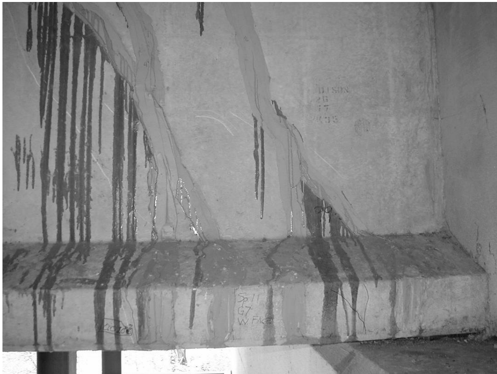
Figure 4.15 Girder 7 Span 11 West Face
