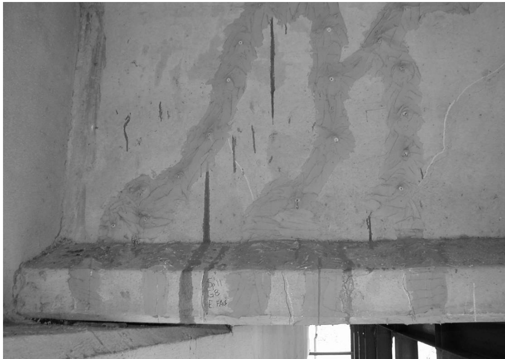
Figure 4.18 Girder 8 Span 11 East Face
