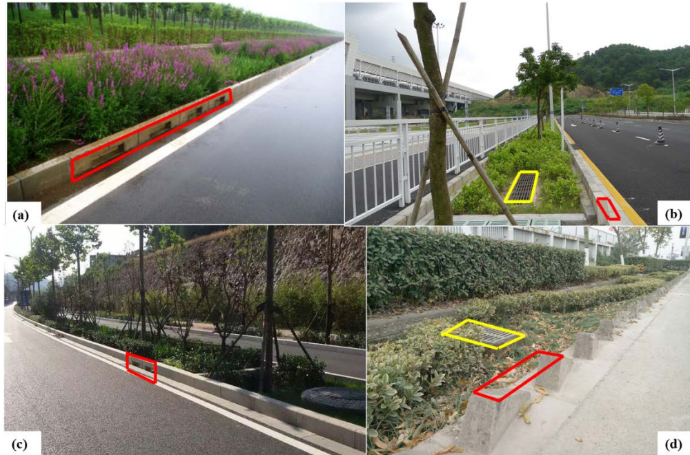
Figure 4.2. Continuous road-bioretention strip in (a) Beijing (curb inlet length L_{ci} = 0.5 m) taken by Yongwei Gong, (b) Shenzhen ( L_{ci} = 0.4 m) taken by Yongwei Gong, (c) Jinan ( L_{ci} = 0.4 m) taken by Xiaoning Li, and (d) Ningbo ( L_{ci} = 0.3 m) taken by Jianlong Wang. Red boxes show curb inlets and yellow boxes show overflow grate inlets in the bioretention cells.
