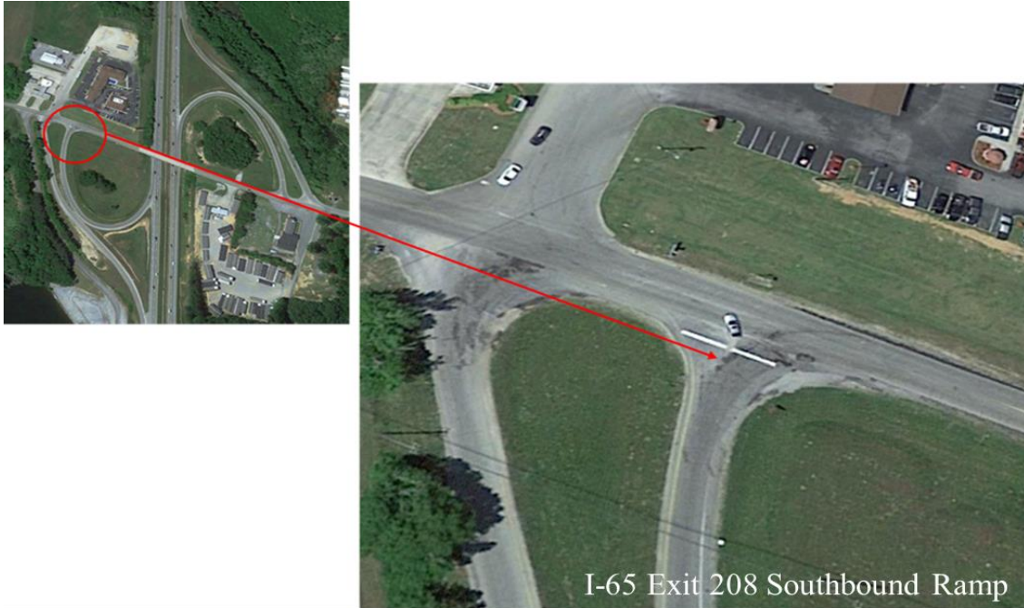
Figure C.4 High-risk exit ramp terminal of parclo interchange
