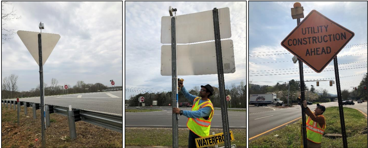
Figure 3.9 Installing cameras at the high-risk exit ramp terminals
