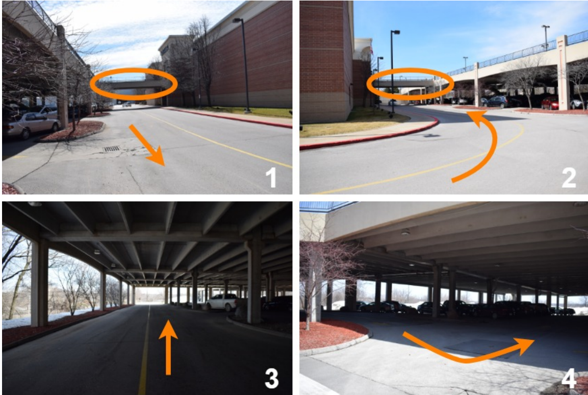
Figure 6.40: Pictures of Parking Deck Trajectory in West Des Moines, IA
