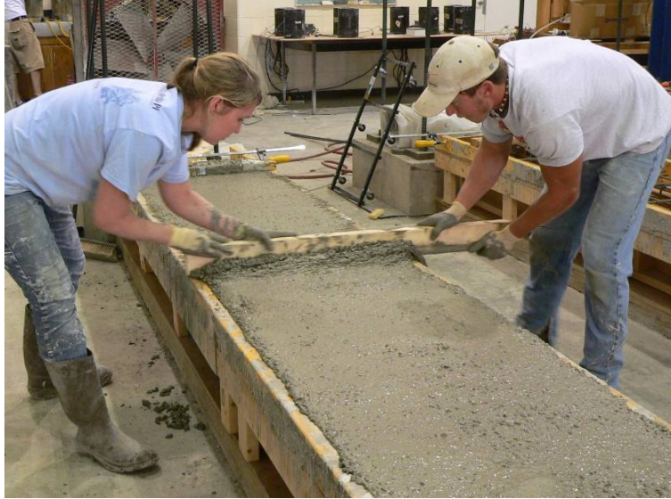
Figure 3-22: Screeding of Excess Concrete
