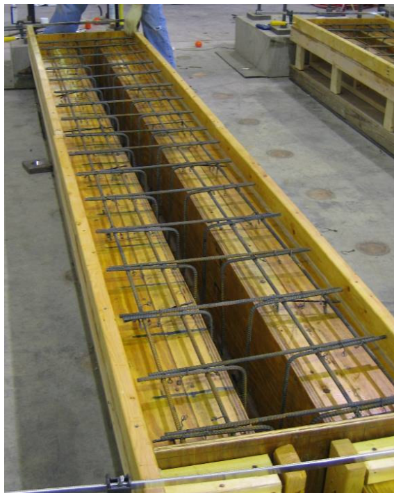
Figure 3-19: Finished Reinforcement Cage
