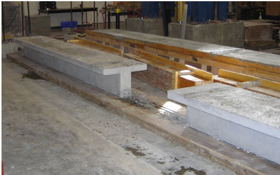
Figure 3-26: Removal of Side Forms
