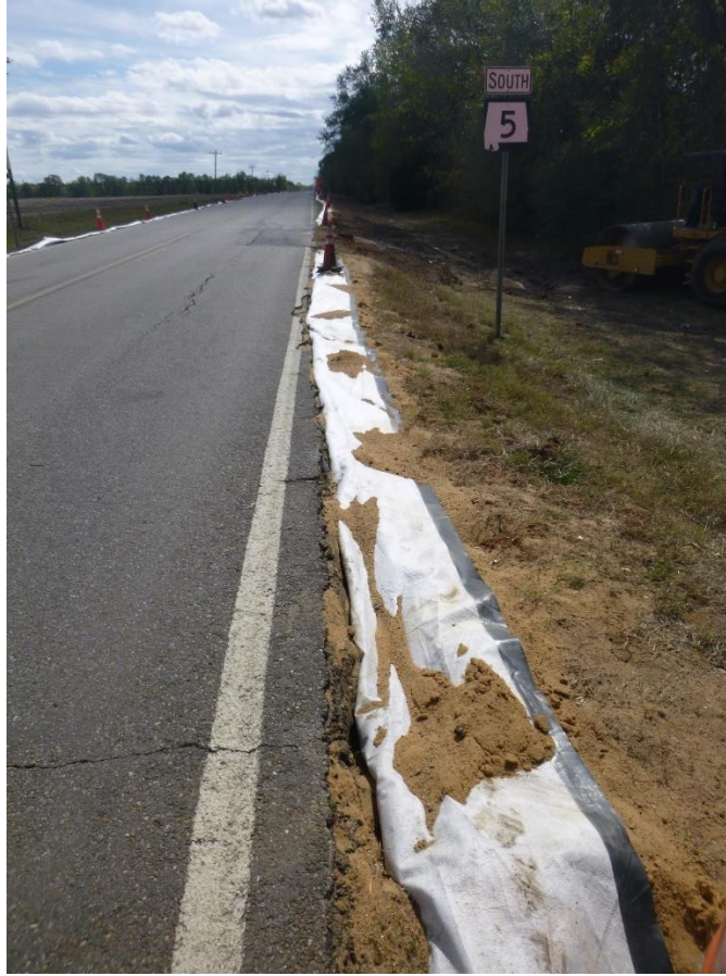
Figure 30: Construction of Vertical Barriers
