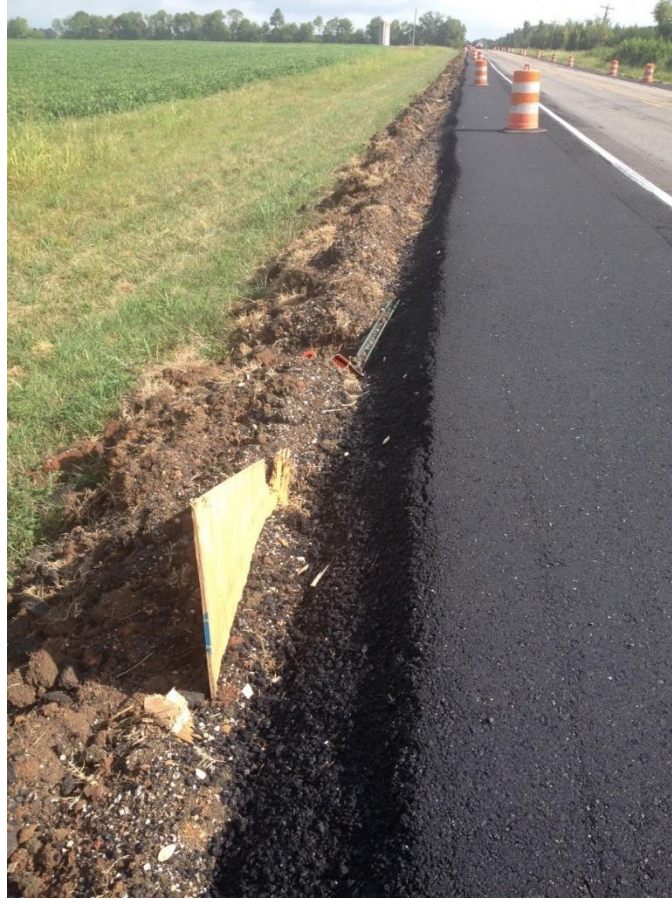
Figure 40: Paved Shoulders After Paving
