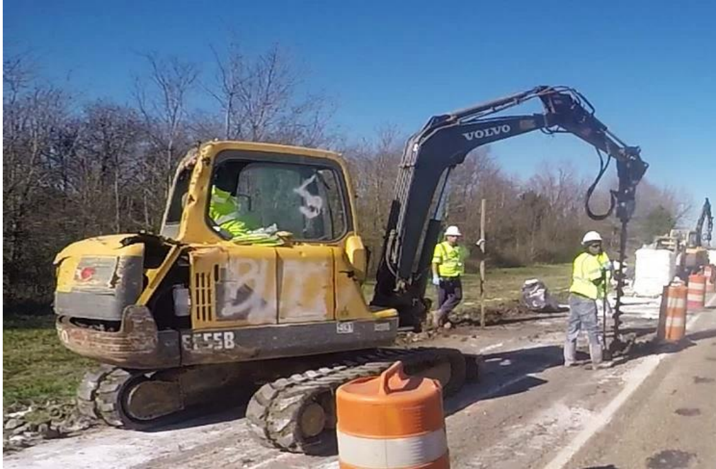
Figure 35: Drill Used for Lime Column Installation
