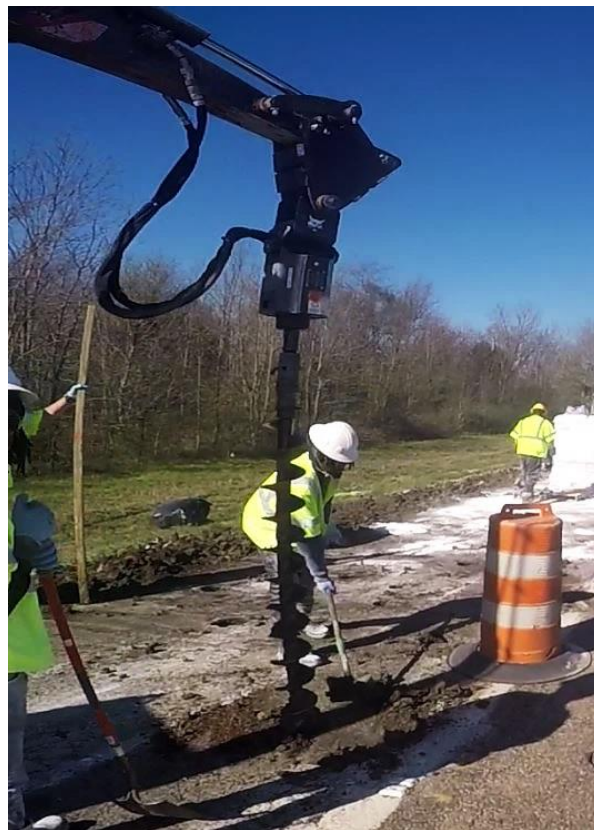
Figure 36: Auger used for Lime Column Installation
