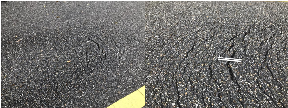
Figure 110: Paved Shoulder Test Section Travel Lane November 2018
