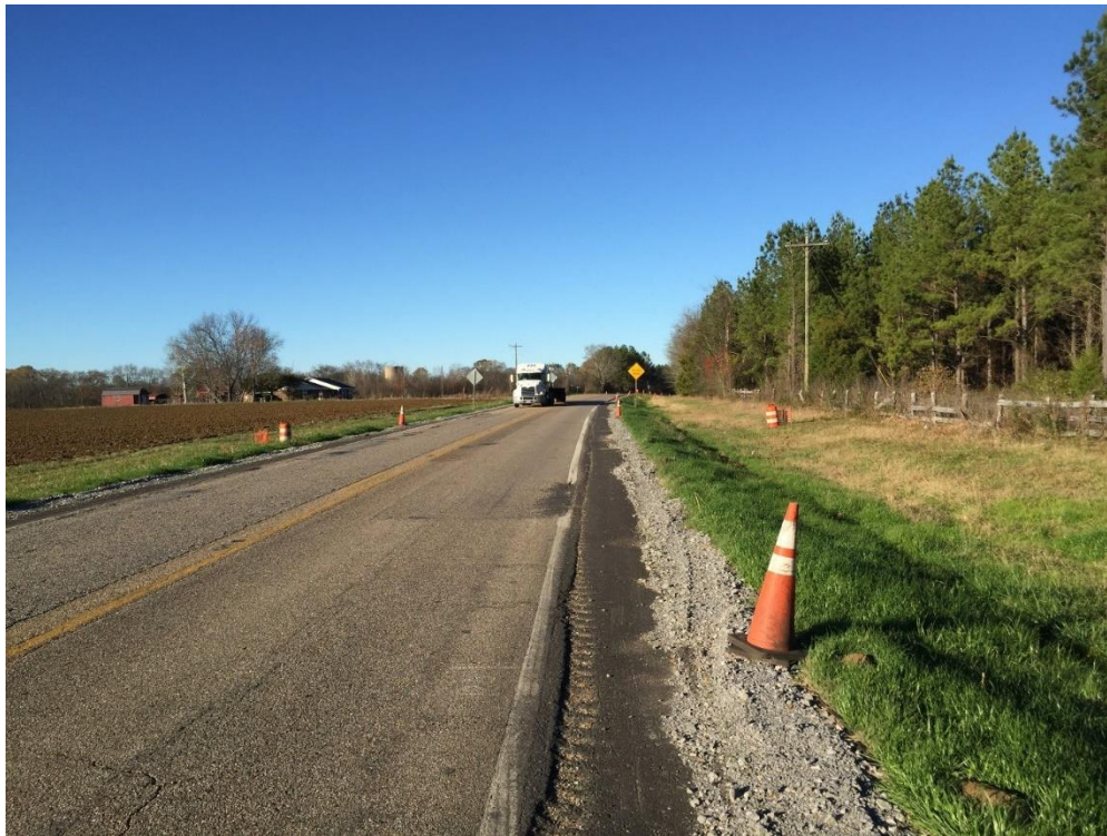
Figure 42: Edge Drains after Backfilling with Stone
