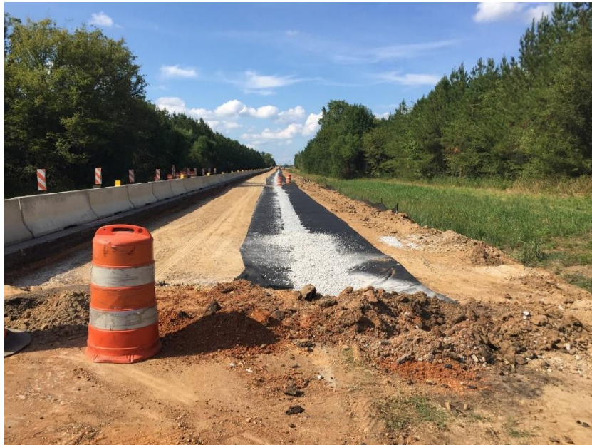
Figure 28: Sand Blanket Construction
