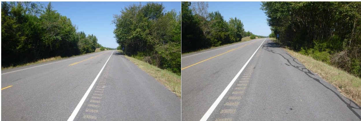
Figure 108: Paved Shoulder Section of AL-5 in Dallas County December 2017
