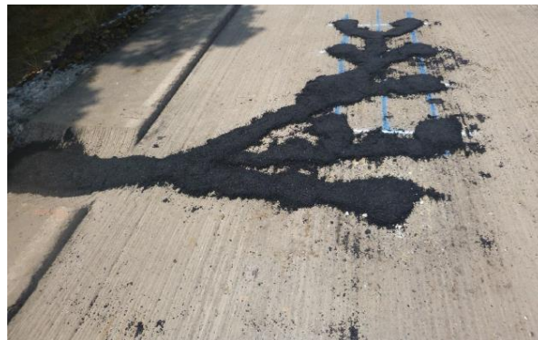
Figure 62: Gage Array on Milled Surface Covered with Screened Asphalt (Jackson 2016)
