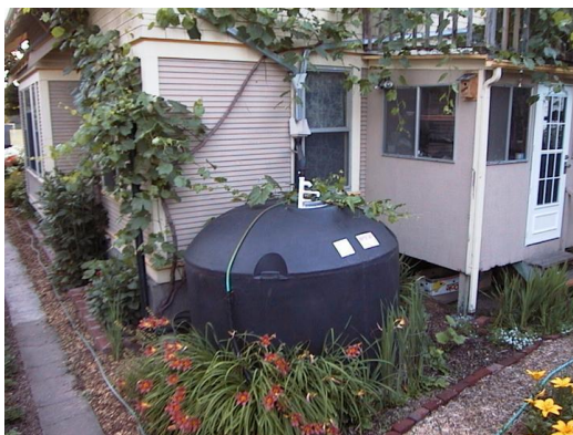
Figure 2.3: Rainwater Harvesting Tank
