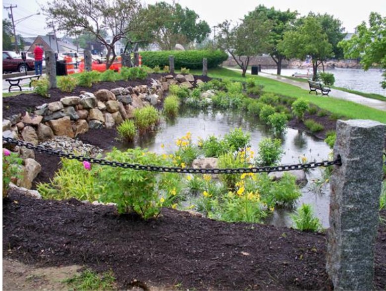
Figure 2.5: Bioretention at Water Street in Plymouth Center, Massachusetts (Source: Hall, 2015).
