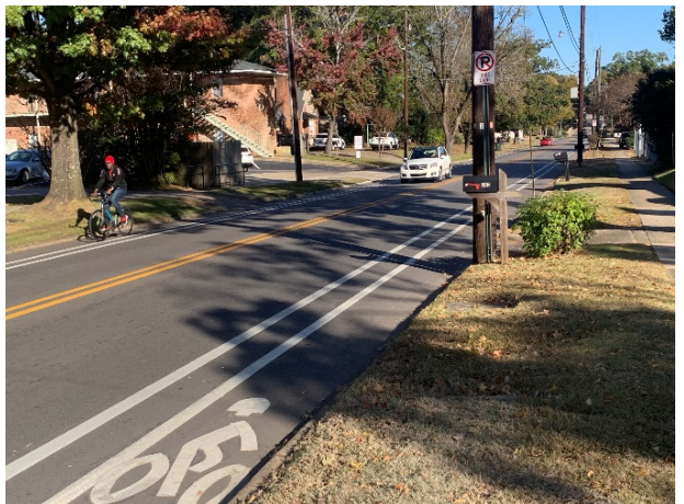
Figure 22: Location 6 - Thach Ave
