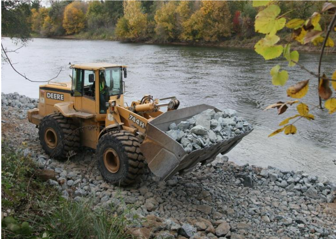
Figure 2.3: Sacramento Riverbank Protection(Nevins 2011)
