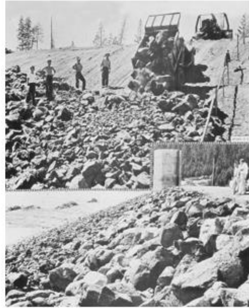
b. Dumped riprap
