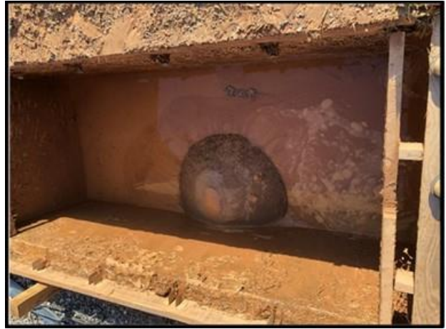
(b) Catch basin
