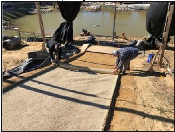
(c) Installing ECB
