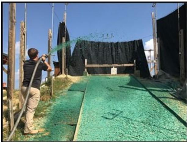
(a) Bottom install
