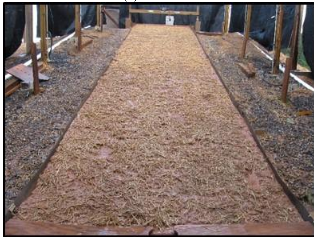
(c) Loose straw with Tacking Agent 3
