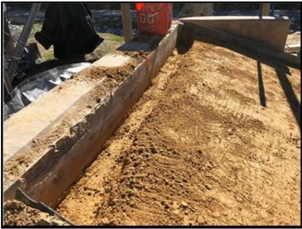
(a) 6" by 6" trench
