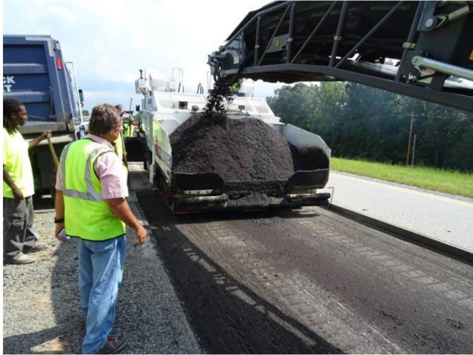
Figure 16. Recycled material loaded into the paver
