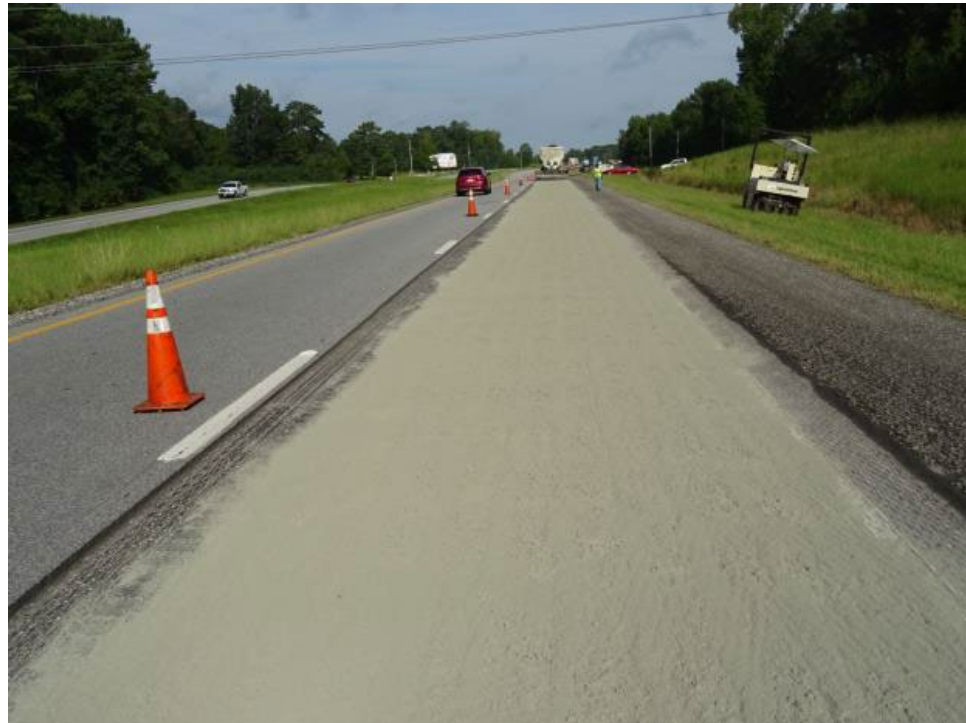
Figure 15. Pre-milling of the CIR sections
