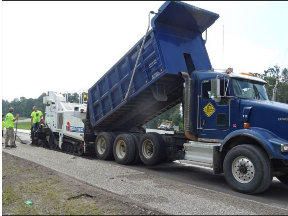
Figure 13. Paving of the CCPR foam section
