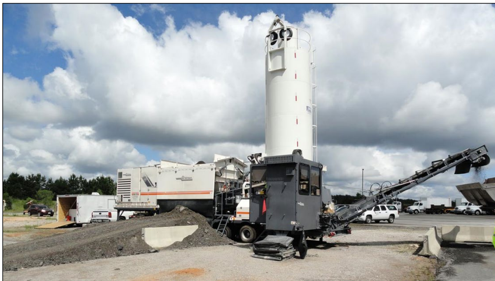
Figure 6. Cold Central Plant Recycling
