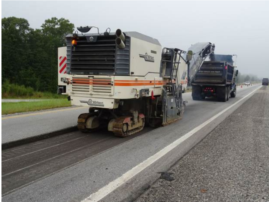
Figure 11. Milling of the CCPR sections
