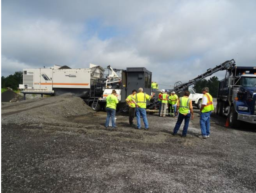
Figure 12. Production of CCPR at NCAT test track
