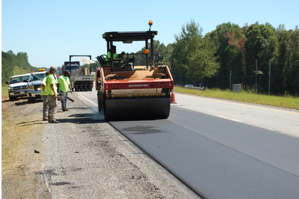
Figure 17. Compaction of the thin overlay
