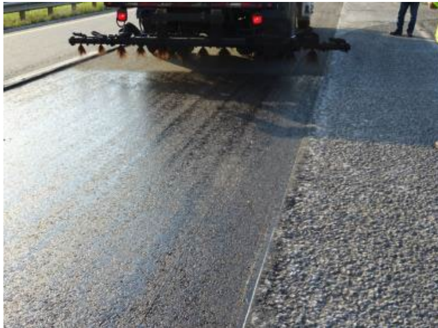
Figure 14. Tack coat application for both sections
