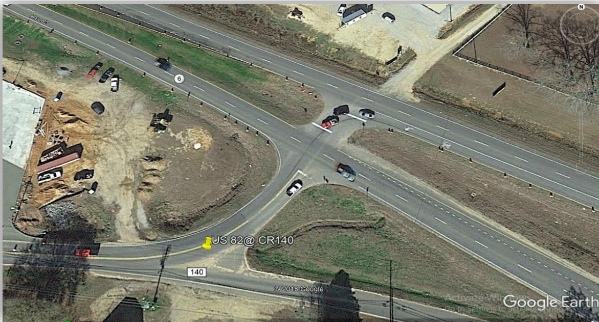
Figure 4- 5: US 82 at County Road 140 Before Condition (Google Earth)
