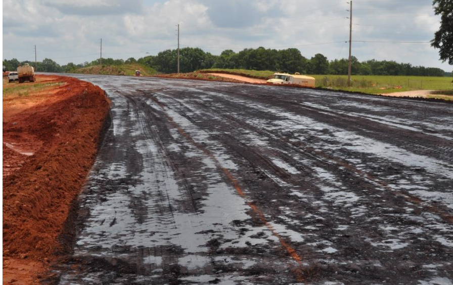
Figure 2.18: Emulsified asphalt coating the compacted soil cement
