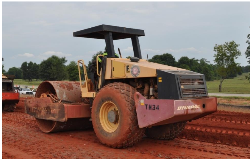
Figure 2.17: Vibratory steel-wheeled roller
