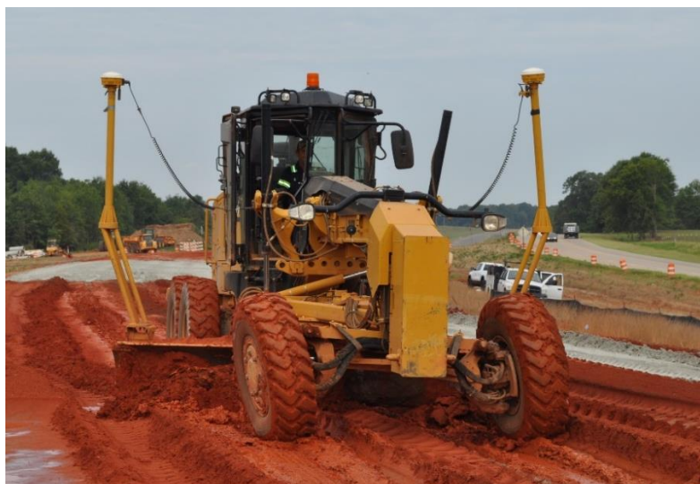
Figure 2.15: Motor grader spreading soil cement
