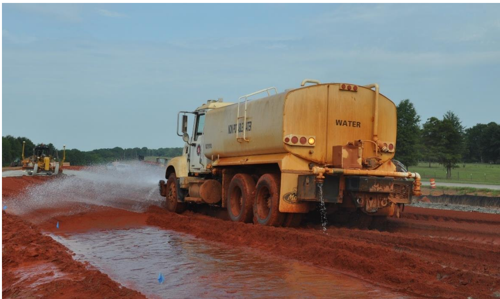
Figure 2.13: Water truck applying water to soil cement
