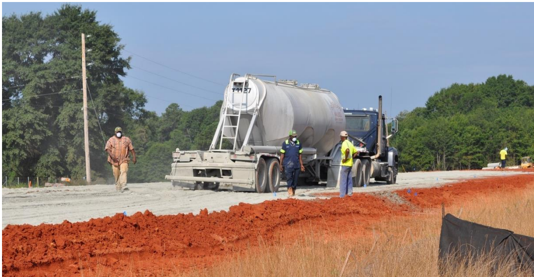
Figure 2.11: Cement being spread by mechanical spreader
