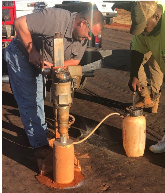
Figure 2.23: Core removal process
