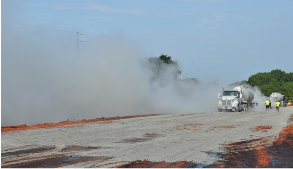
Figure 2.12: Cement dusting into the air
