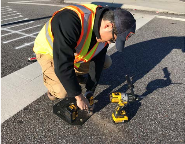
(a) Installing the Protective Cover
