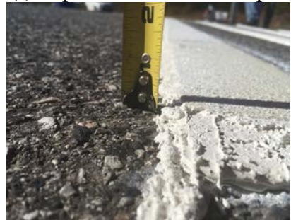
(i) Inspection after installation
