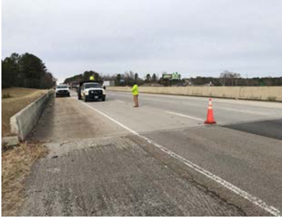
(a) Traffic control (ramp closed)
