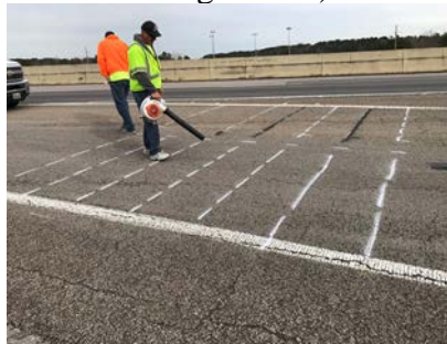
(e) Clean the surface
