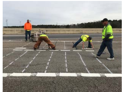
(f) Tape the ends of the strips
