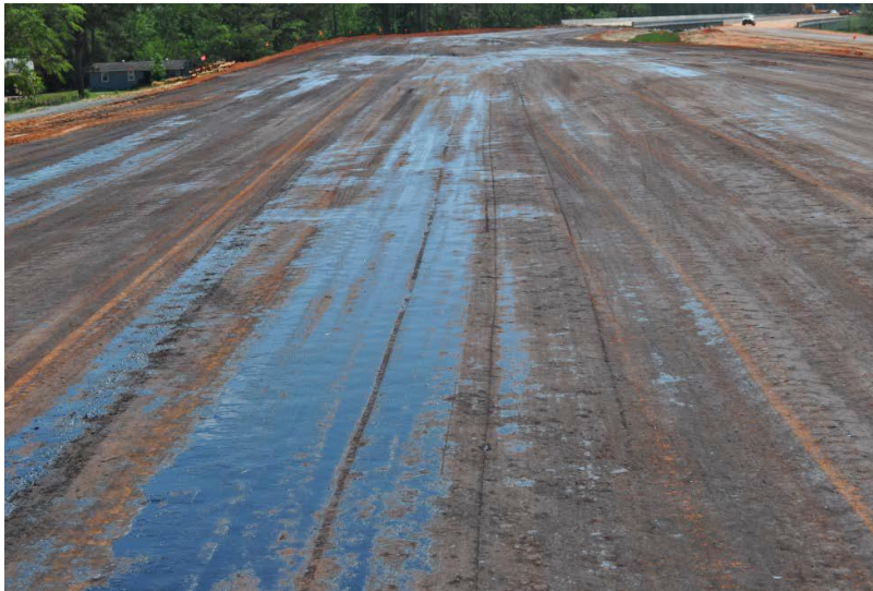
Figure 0.20: Asphalt emulsion placed on the soil cement base (McLaughlin 2017)
