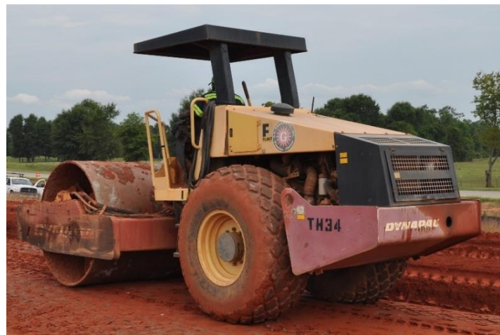
Figure 0.18: Vibratory steel-wheeled roller compacting soil cement (Scales 2020)
