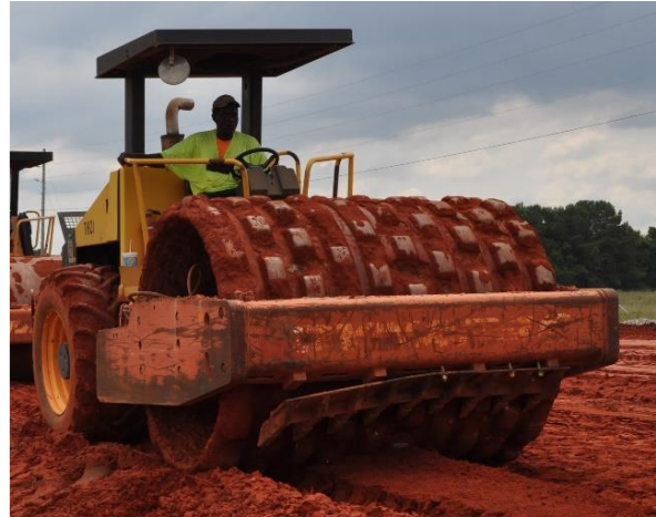
Figure 0.17: Pad foot roller compacting soil cement (Scales 2020)
