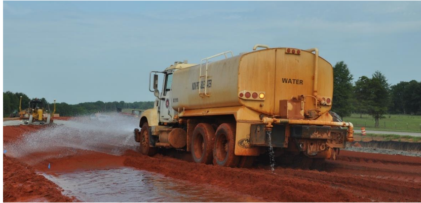
Figure 0.13: Water truck applying water to soil cement (Scales 2020)
