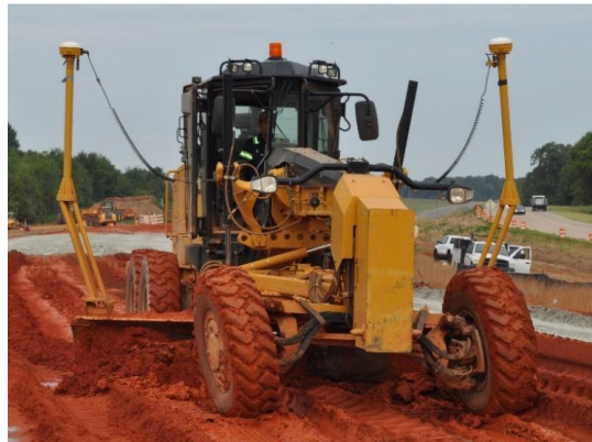
Figure 0.16: Motor grader spreading soil cement (Scales 2020)
