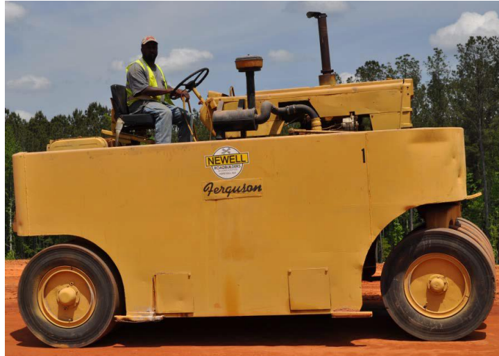
Figure 0.19: Multiple-wheel rubber-tire roller used to finish soil cement base (McLaughlin 2017)
