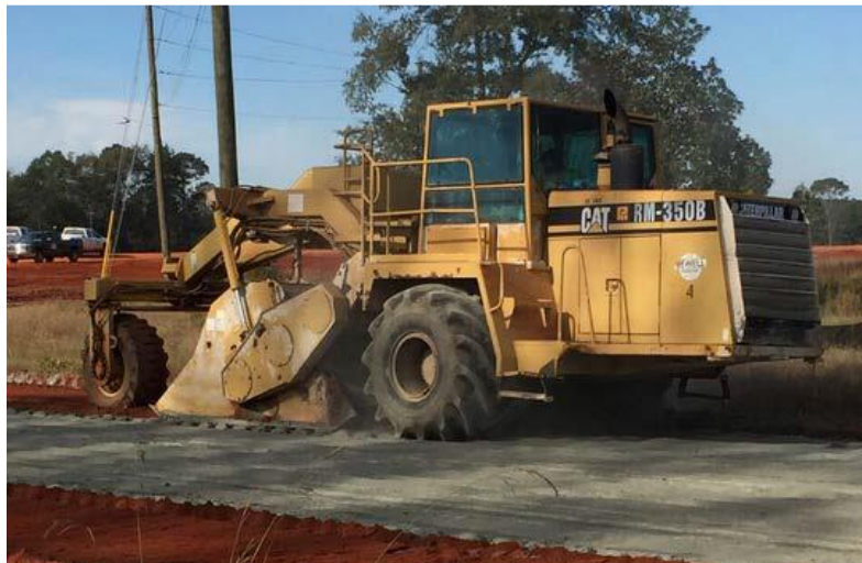
Figure 0.12: Single-shaft mixer used in mixed-in-place construction (McLaughlin 2017)
