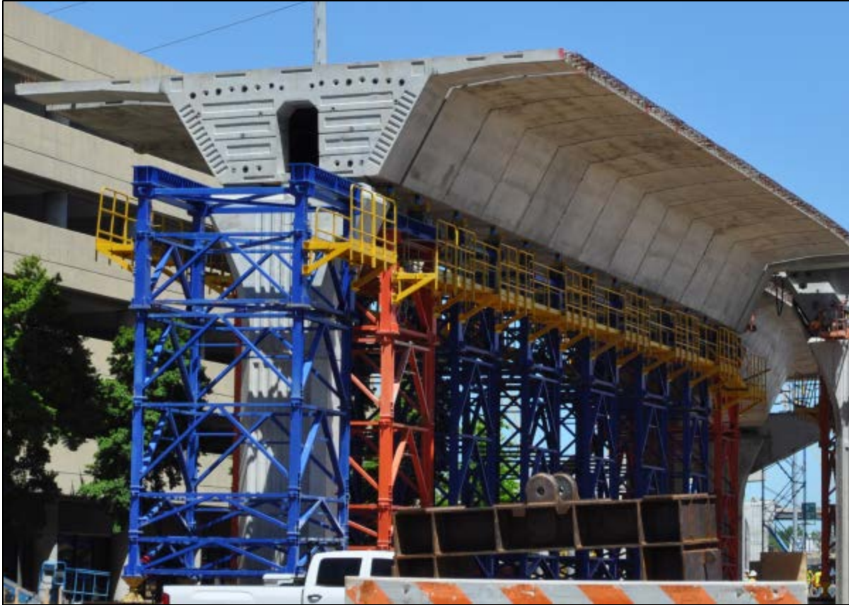
Figure 4-15: Falsework used to erect each span
