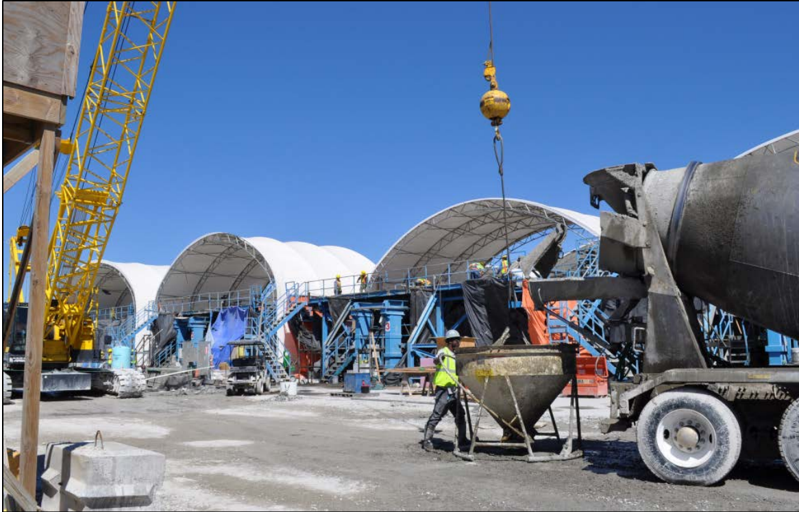
Figure 4-9: Concrete bucket being filled by ready-mixed concrete truck
