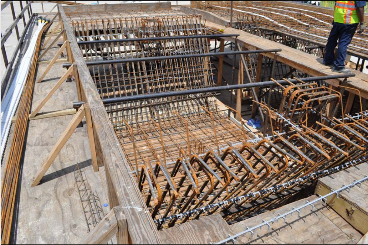
Figure 4-3: Reinforcement fabrication box for increased construction efficiency
