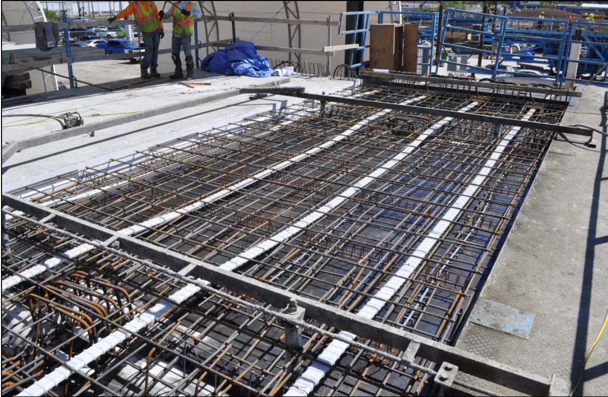
Figure 4-5: Formwork for a segment ready for concrete placement
