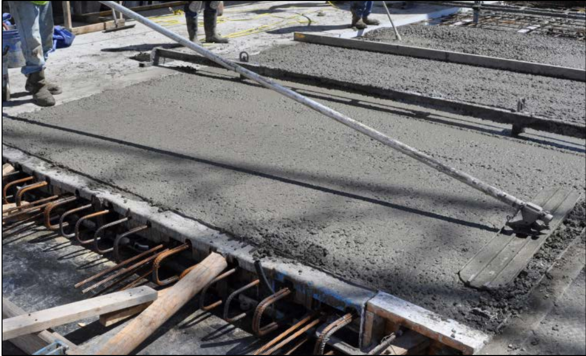
Figure 4-12: Concrete being floated using a bull float
