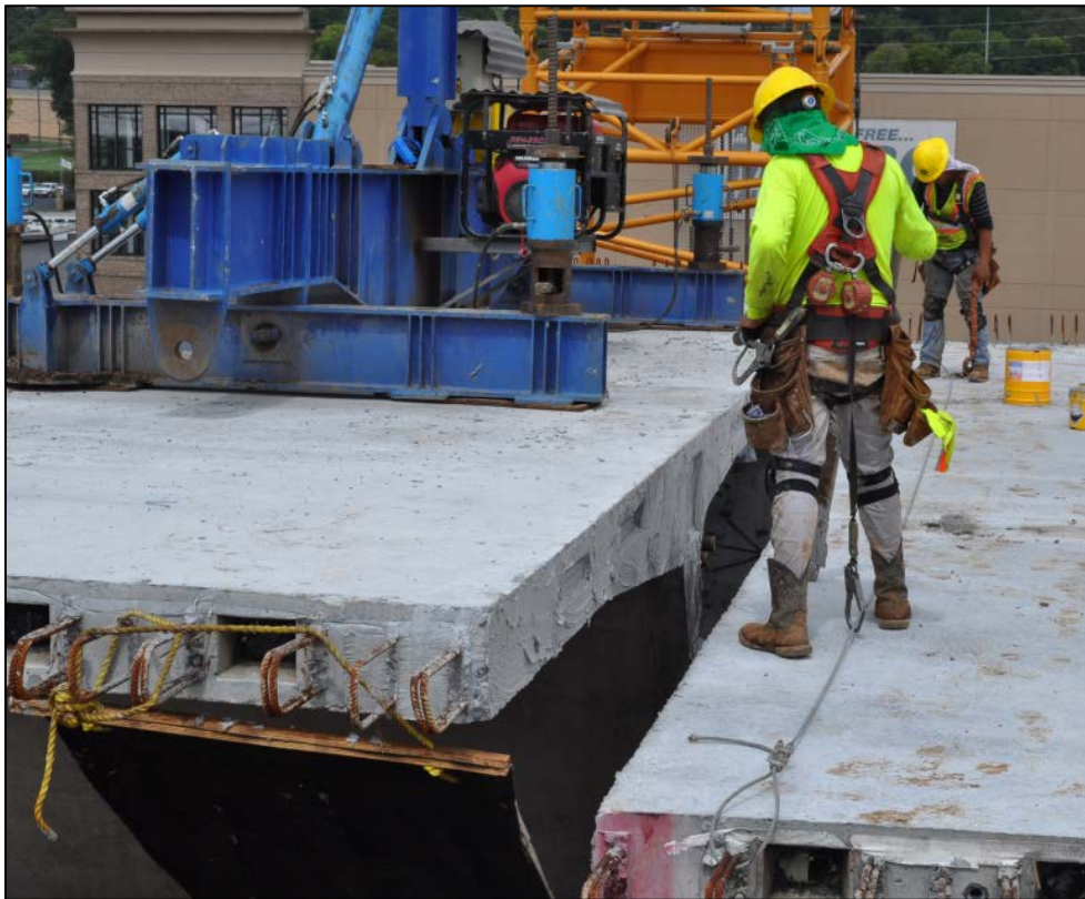
Figure 4-17: Segment being guided into place on falsework
