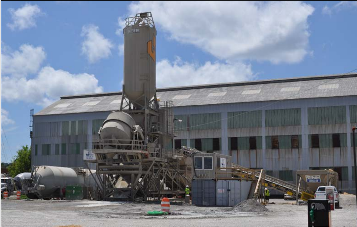
Figure 4-6: On-site batching plant for concrete production
