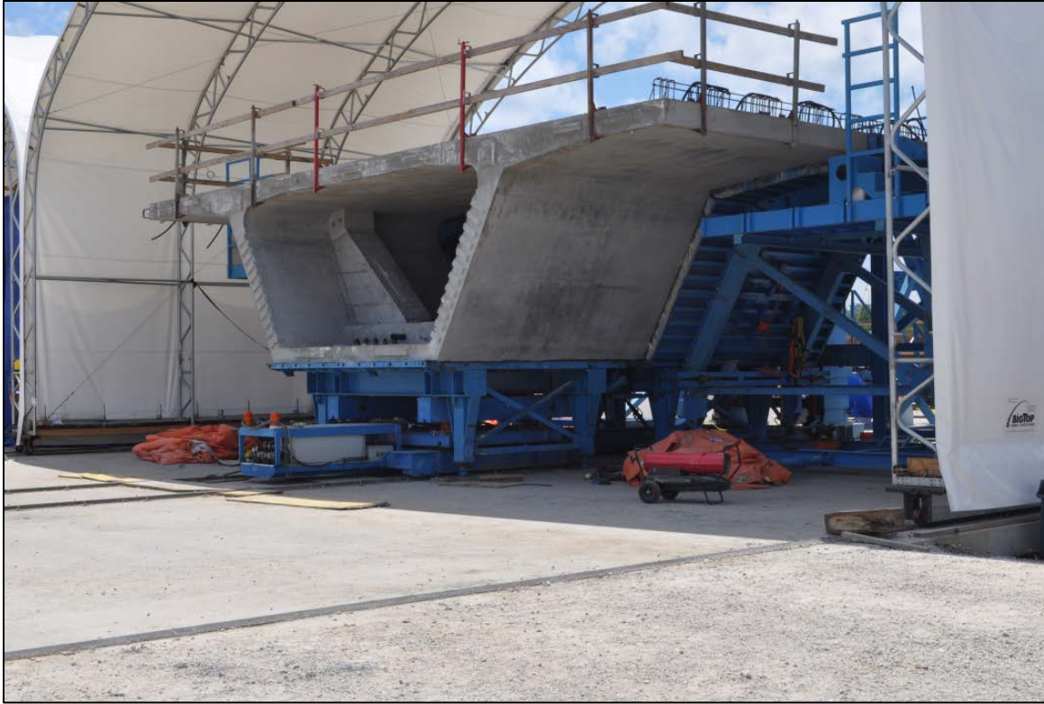
Figure 4-13: Roll-away canopy to protect each form from severe weather
