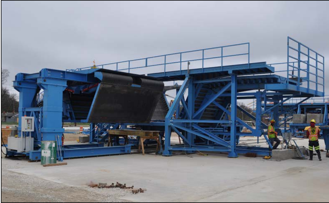
Figure 4-4: System on rails used to remove internal cell of the formwork
