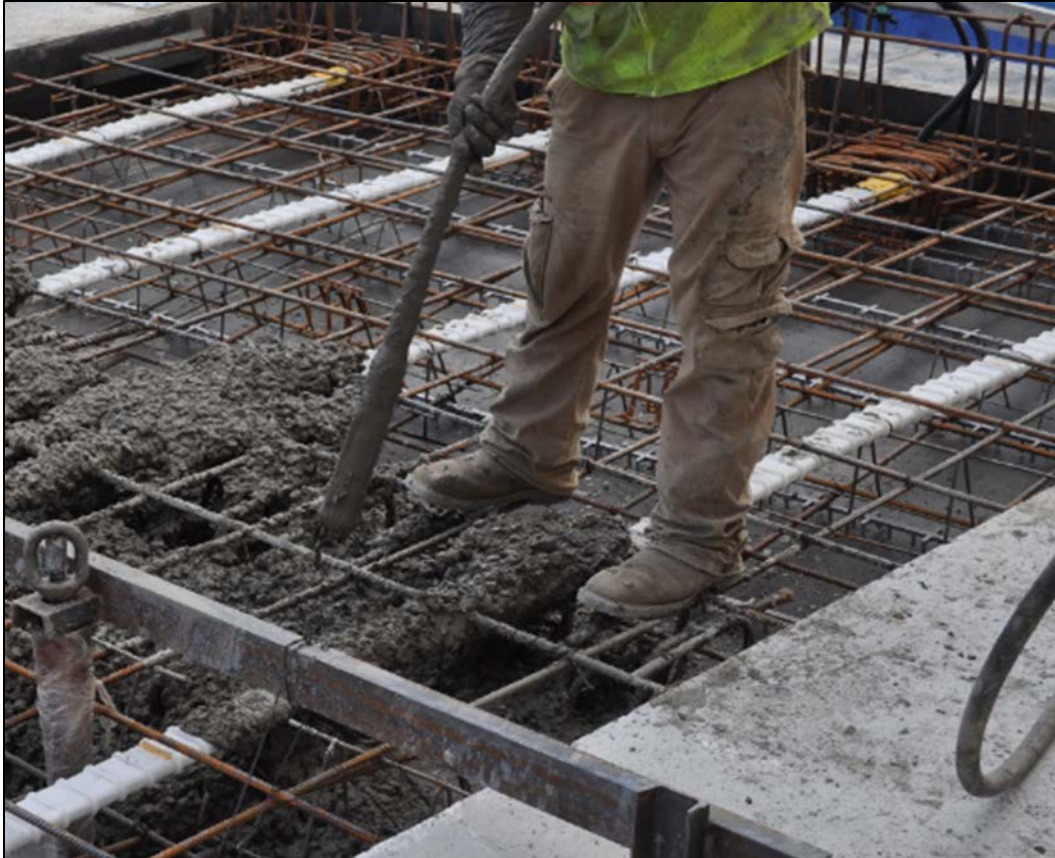
Figure 4-11: Consolidation using a portable vibrator
