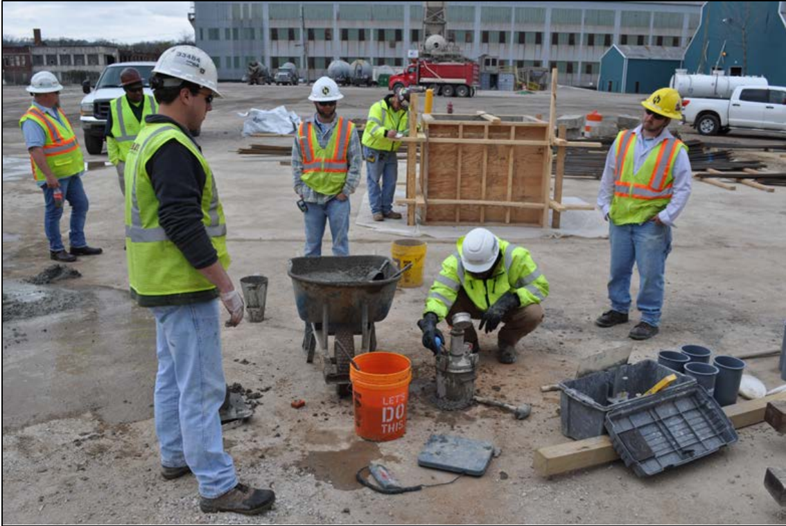
Figure 4-7: Quality assurance testing prior to concrete placement
