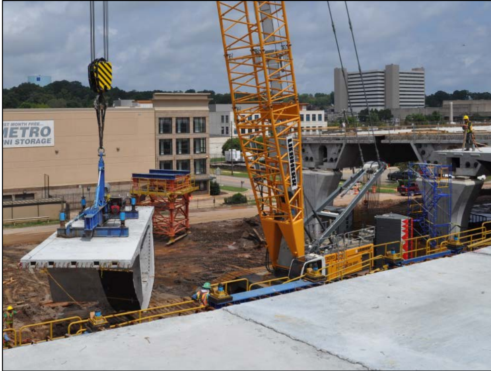
Figure 4-16: Crane lifting a segment into place
