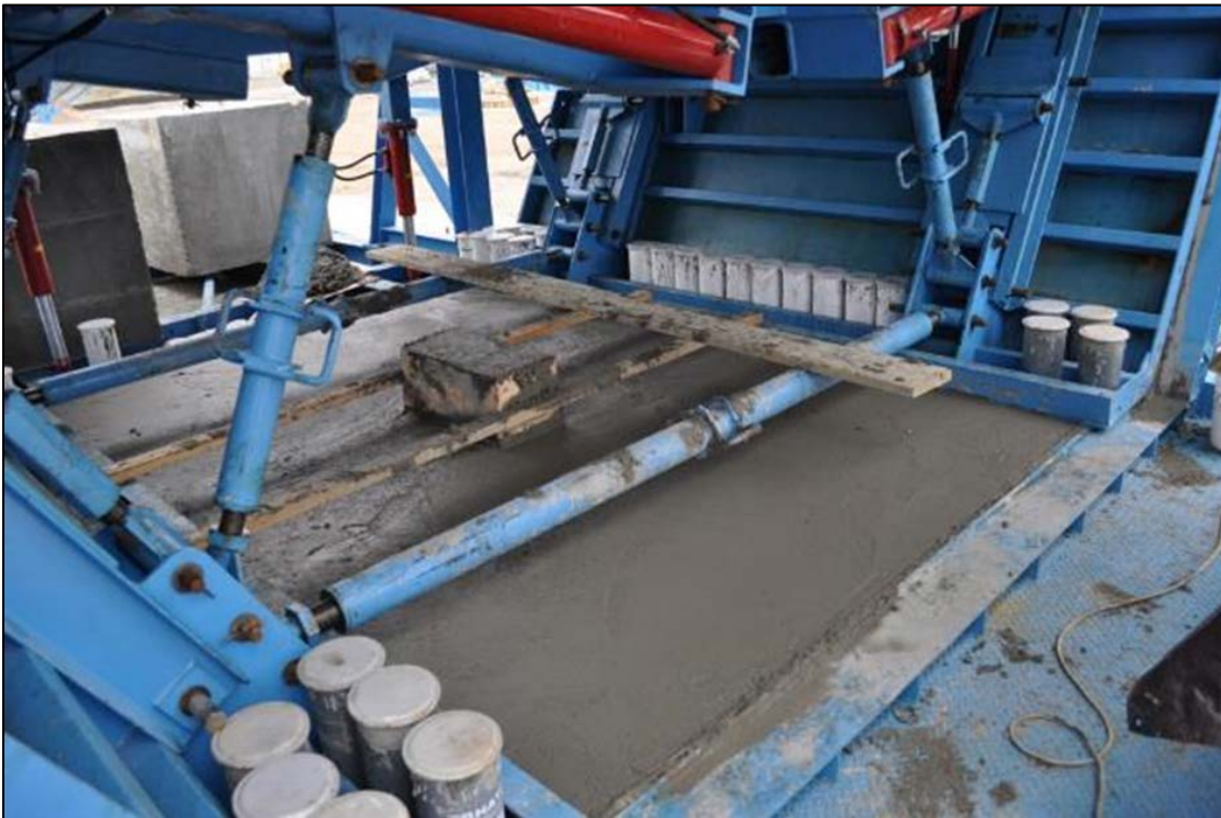
Figure 3-6: Specimens being placed in formwork for on-site curing
