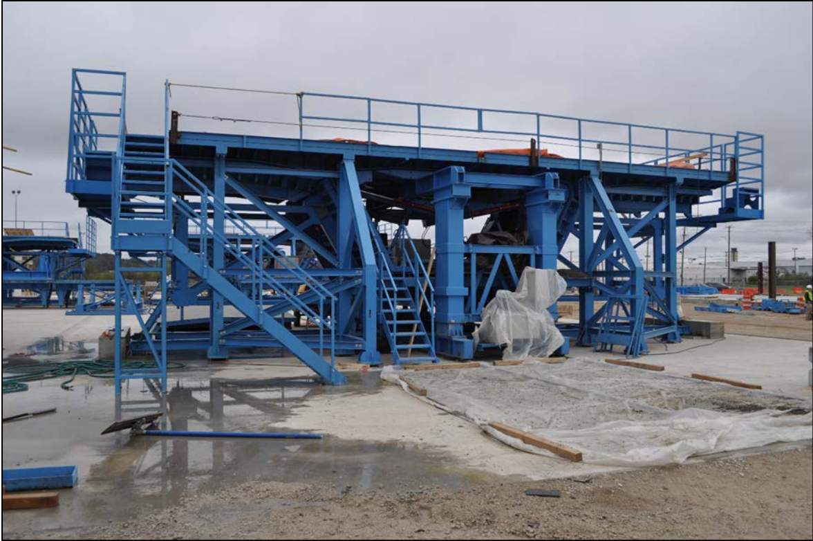
Figure 4-2: Formwork used to cast segments
