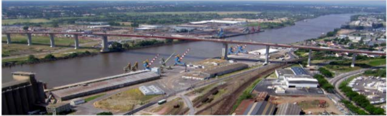
Figure 2-23: Chevre Bridge located in France (Raphael et al. 2018)
