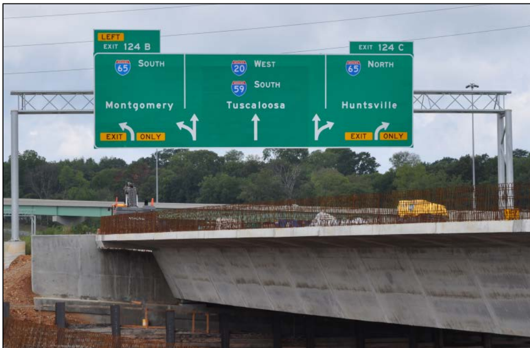
Figure 1-1: Birmingham I-59/I-20 Interchange amid segmental bridge construction
