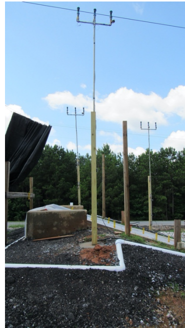
(b) Constructed riser
