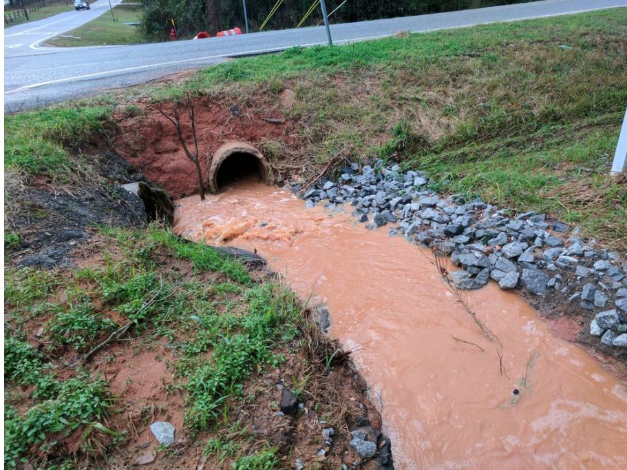
Figure 1-1 Construction Site Stormwater Runoff (Keeper 2017)
