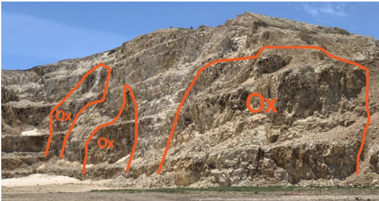
Figure 46. The wall of Stone Cabin open pit. The orange lines outline the more oxidized rock (darker). This area of oxidation is controlled by fractures and faulting.
