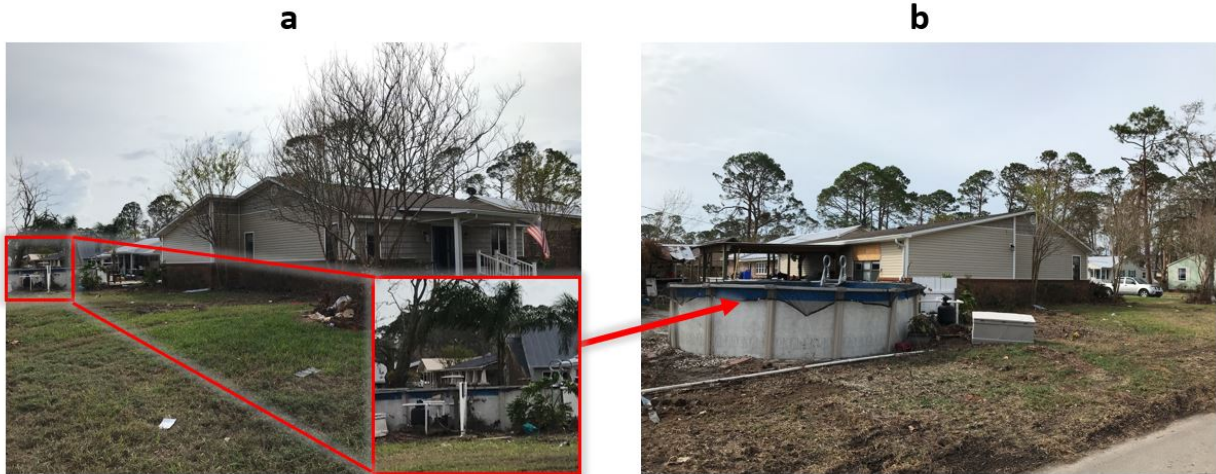
Figure 3.16: An example of how to anchor the different sides of the structure based on details around the structure. a) shows a pool at the back left side of a structure impacted by Hurricane Michael (2018). b) shows a second image of the structure. The location of the pool relative to the structure indicates that this is the back of the structure. The arrow points to the pool.
