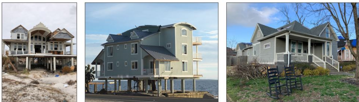
Figure 4.7: Examples of structures that have complex roofs based on StEER’s DE/QC handbook guidelines.
