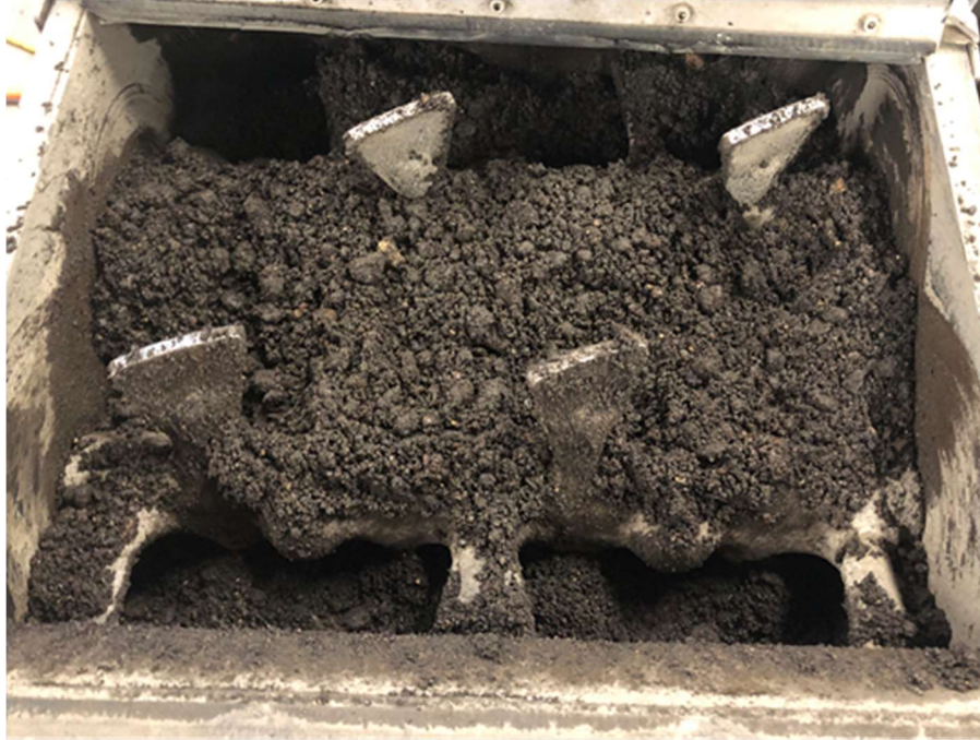
Figure 19: Recycled asphalt mixture in the WLM-30 pugmill before foamed asphalt injected.
