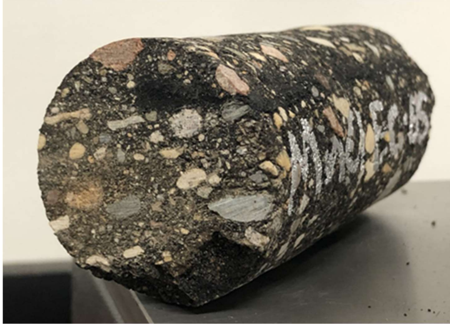
Figure 37: CIR-E PMFC-S specimen with crack seal along its longitudinal axis.
